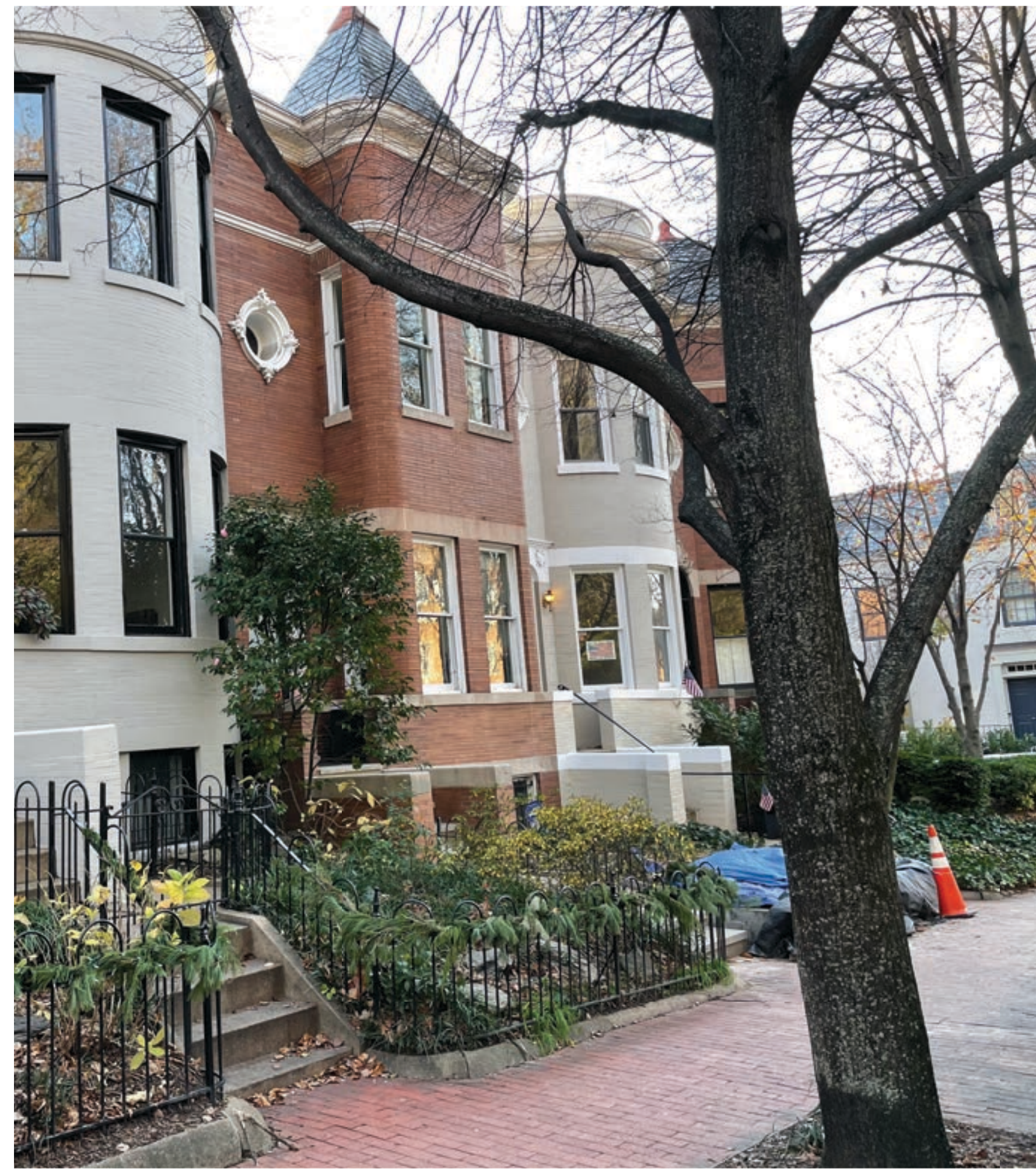
3146 Q ST EXISTING CONDITION FROM EAST
