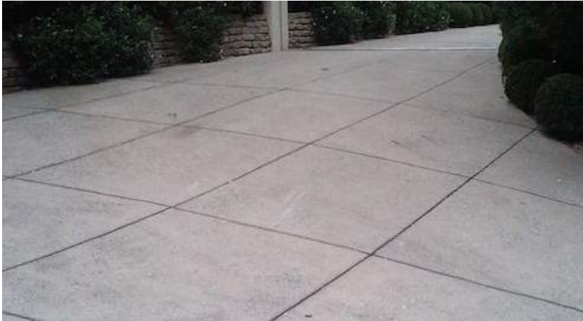
SIDEWALKS AND ENTRY PLAZA - SAWCUT CONCRETE PAVING
