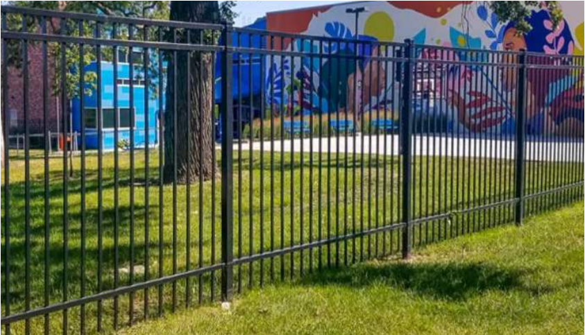
SITE FENCING - METAL PICKET
