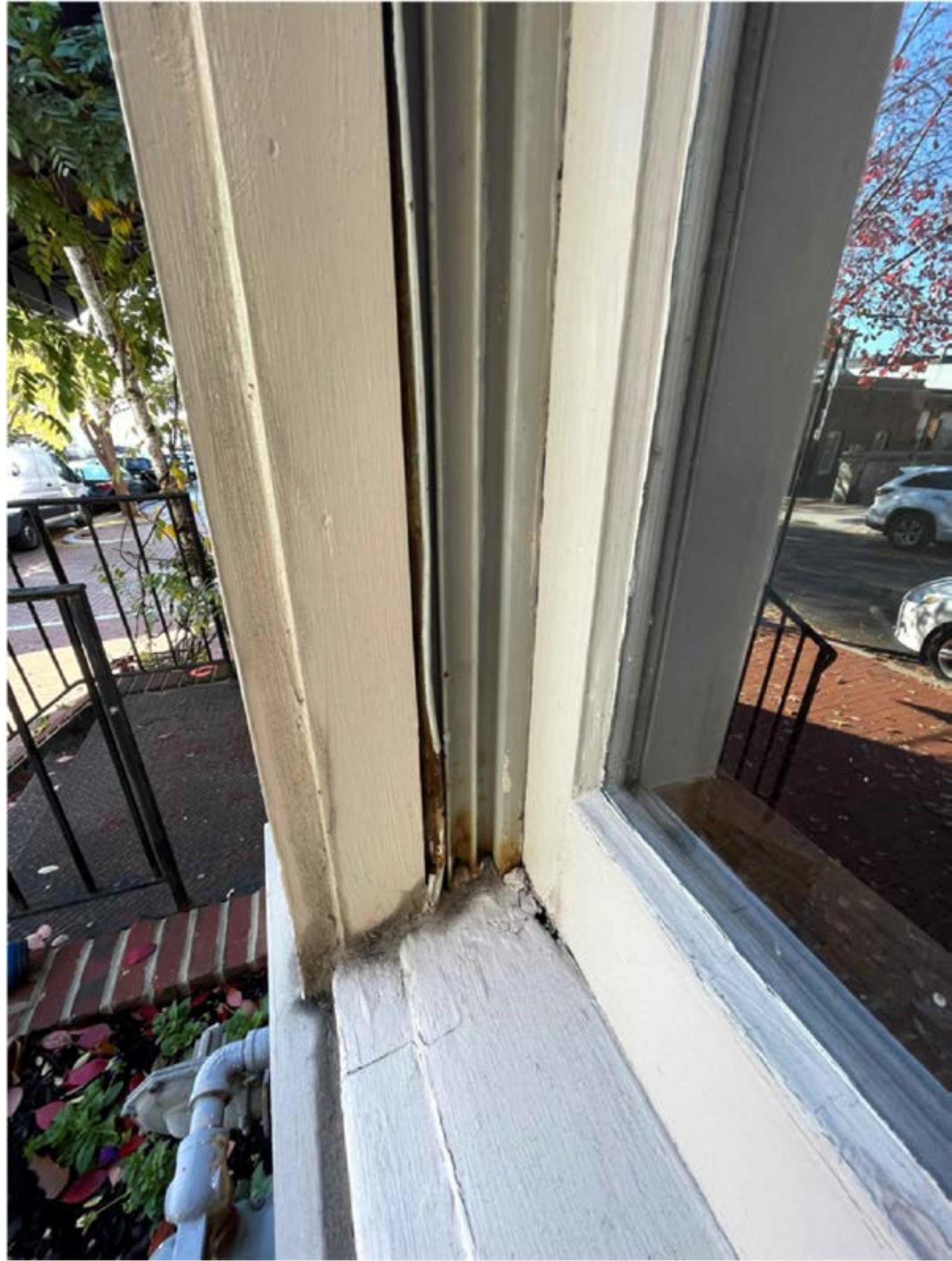
EXAMPLE OF WARPED/ROTTED METAL TRACK
