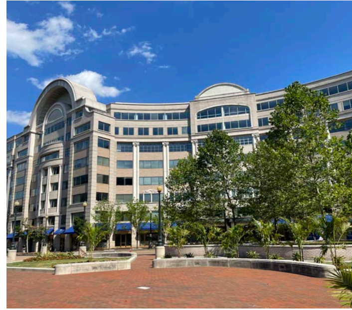
7. MARYLAND AVE FACADE AT CIRCLE
