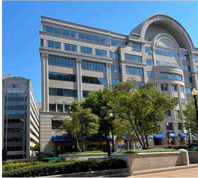
8. MARYLAND AVE FACADE NE CORNER
