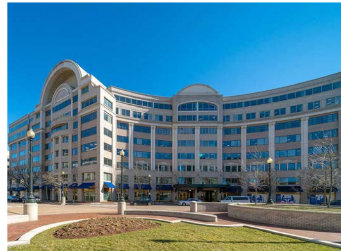
2. MARYLAND AVE FACADE AT CIRCLE
