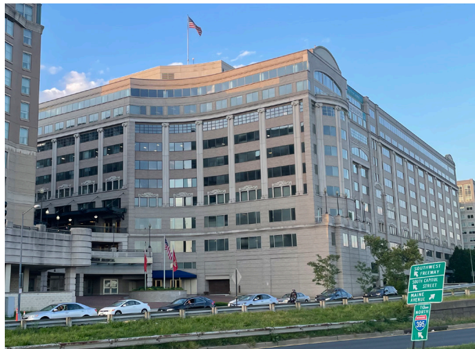
4. WEST FACADE AT SOUTH END
