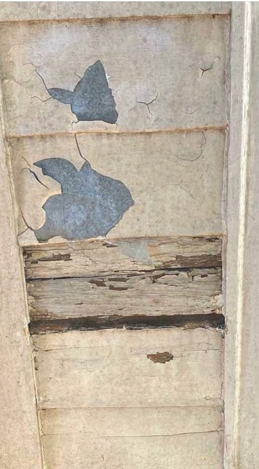
EXISTING METAL SIDING OVER WOOD SIDING
