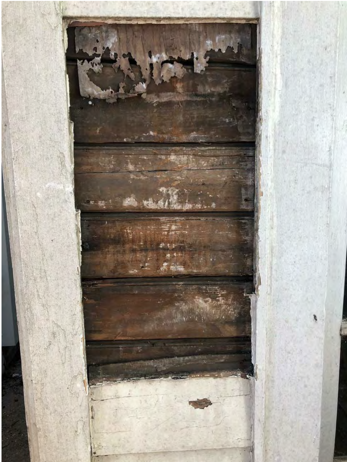
METAL SIDING TO BE REMOVED & WOOD TO BE RESTORED
