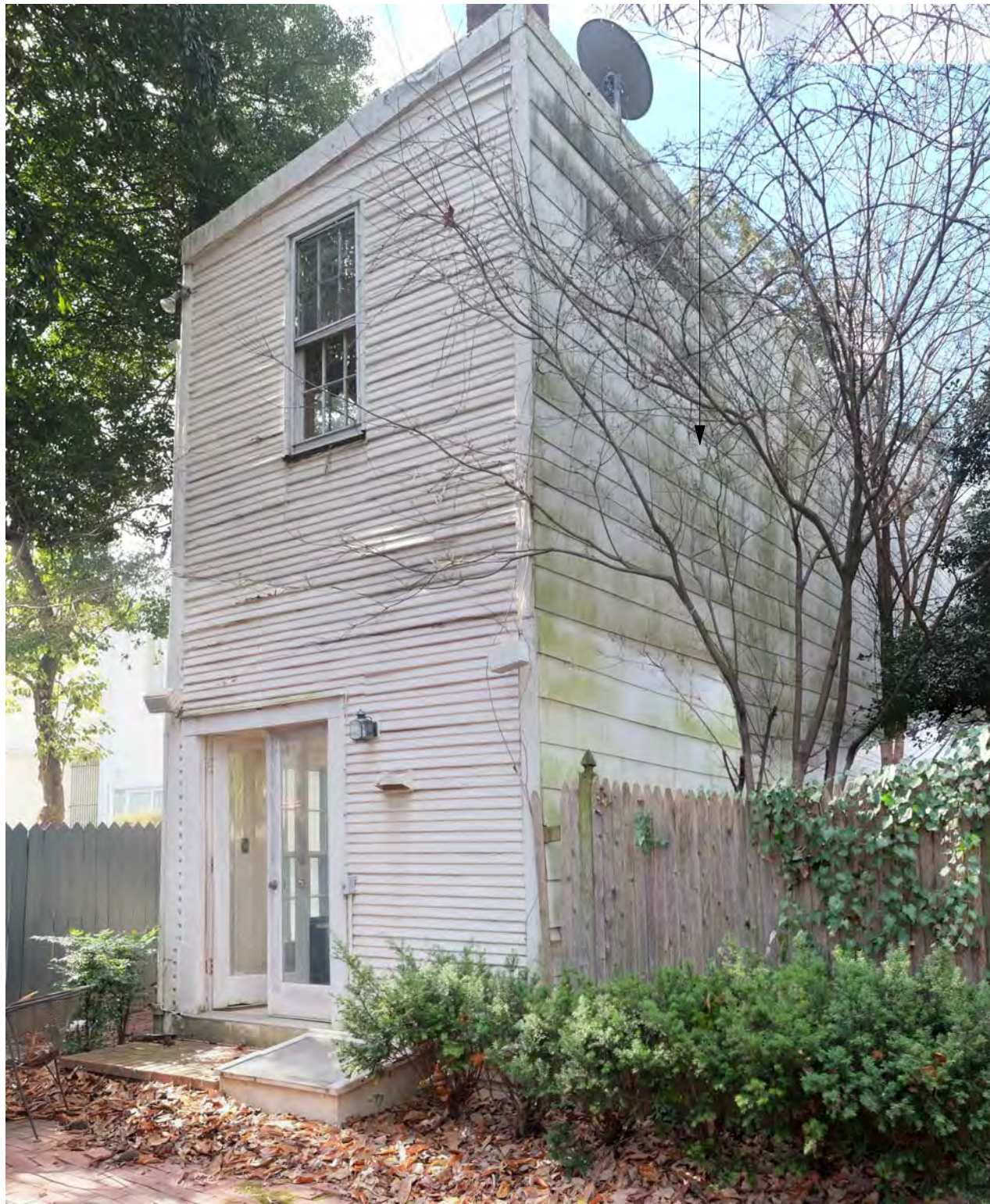
FIBER CEMENT SIDING TO BE REPLACED
