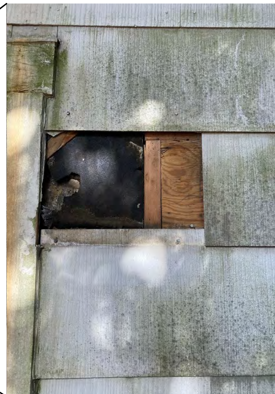
FIBER CEMENT SIDING TO BE REPLACED
