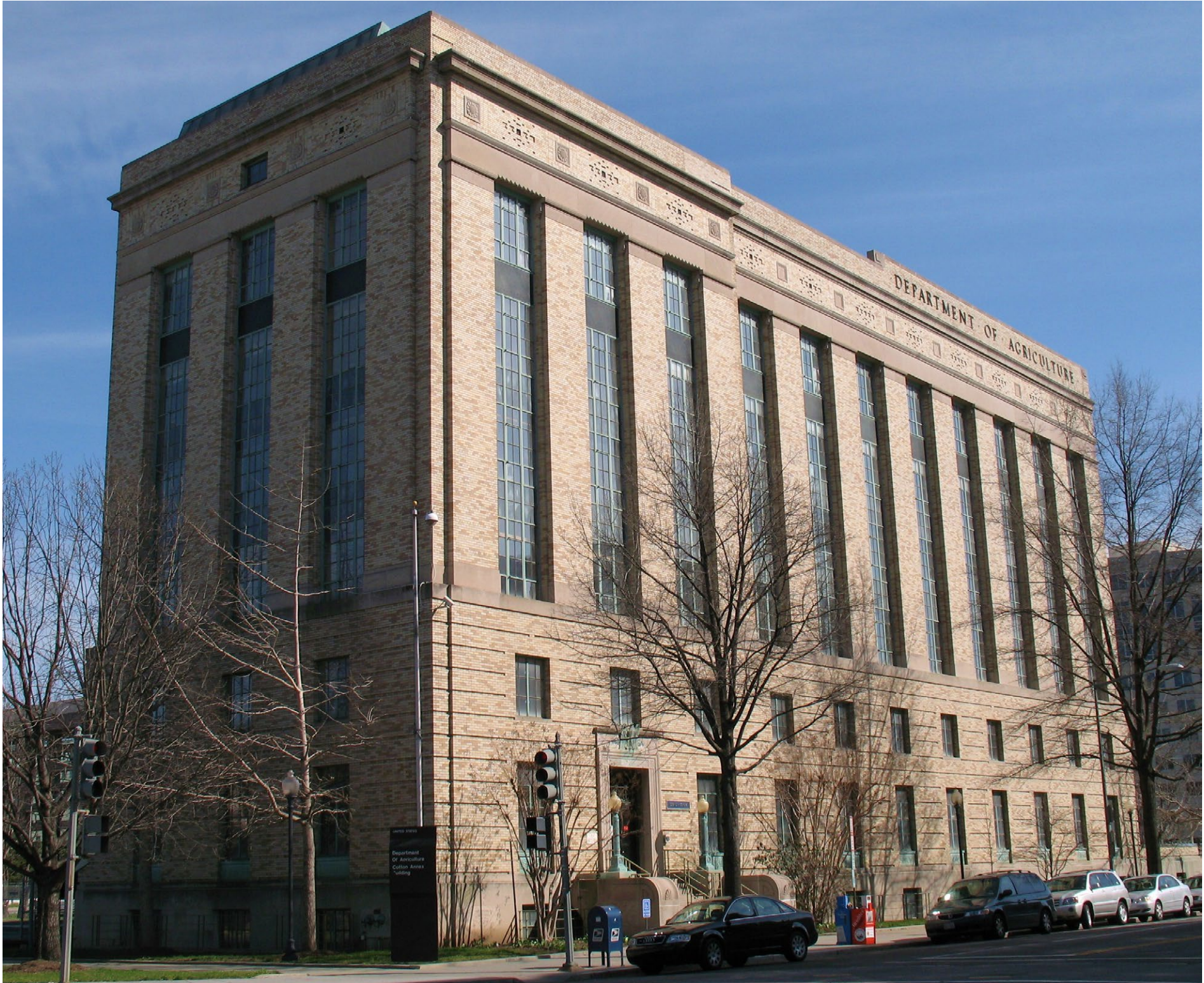
VIEW FROM NORTHWEST (C ST & 12TH ST SW)
