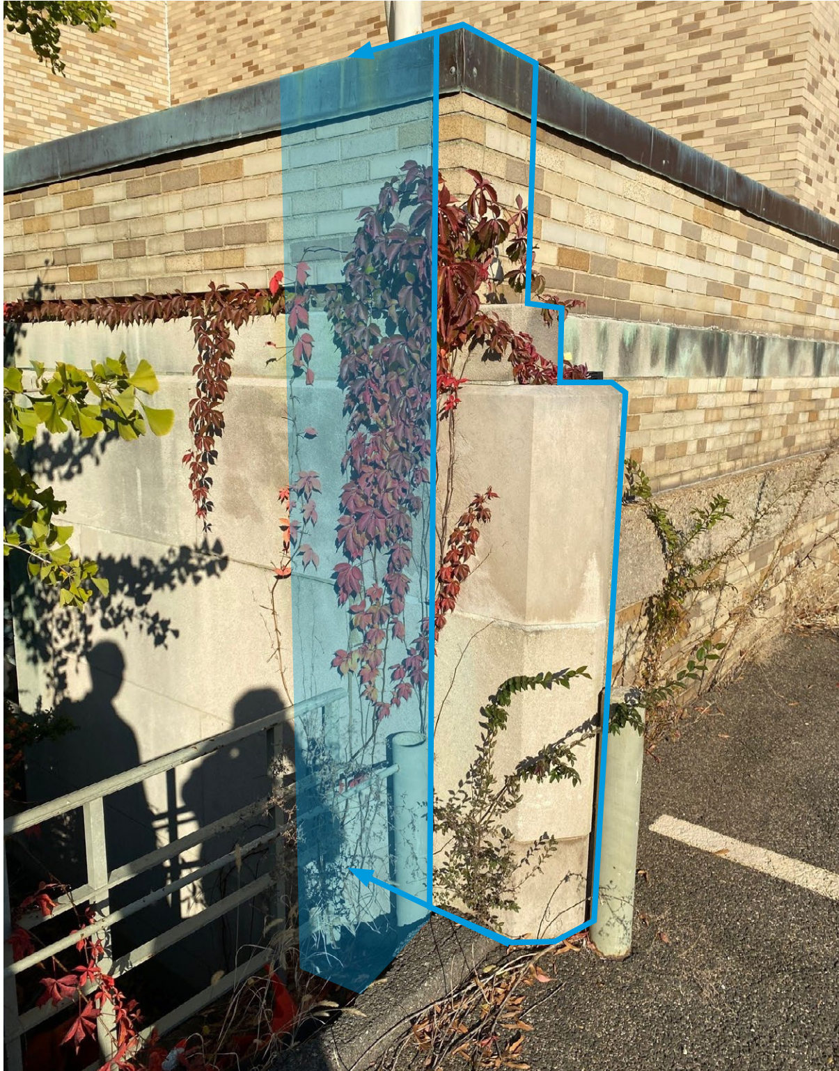
UNMODIFIED UNFINISHED END-WALL CONDITION
