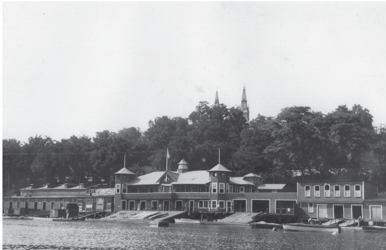
Historic photo East Bay first floor boat bay doors
