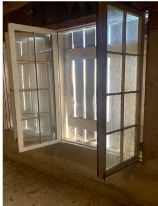
First Floor Grille Room
