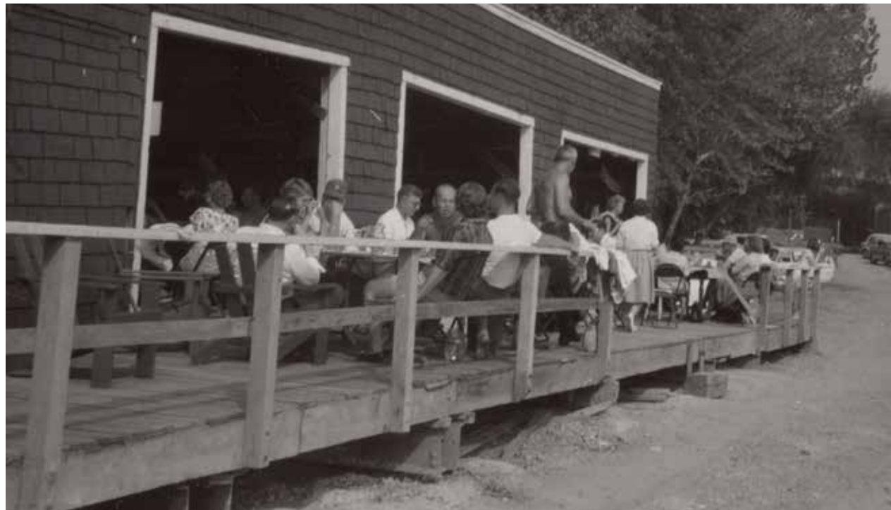
Historic photo East Bay first floor boat bay doors
