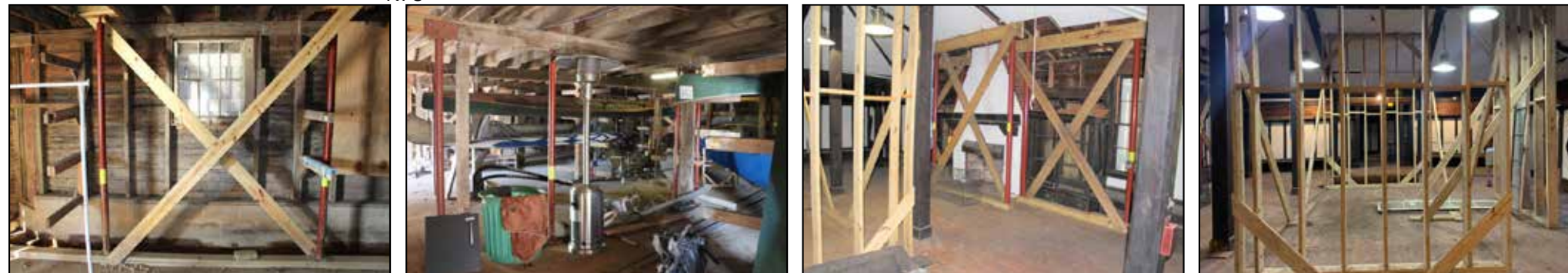
2010-2013: Original portion of WCC and c. 1909 addition closed due to structural instability; temporary stabilization efforts undertaken by NPS
