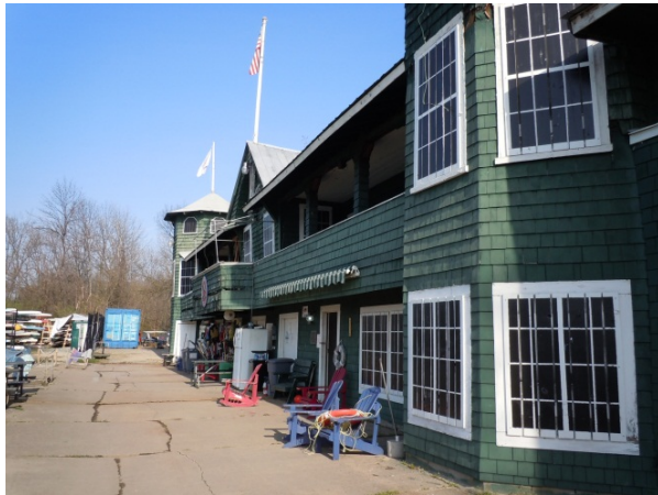
South elevation with concrete apron installed between building and river shore (4/19/13 HPTC).
