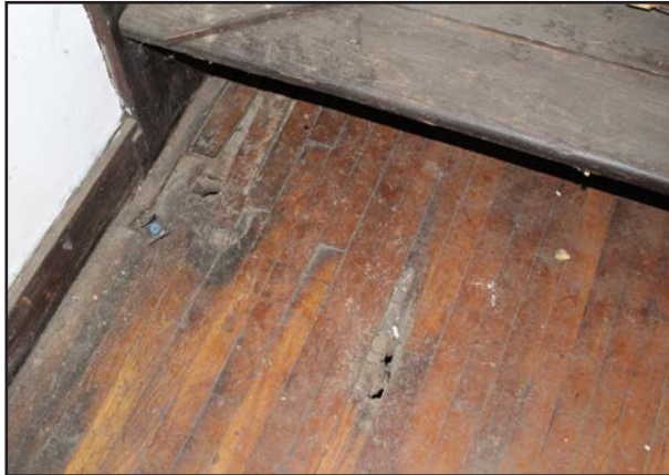
FIGURE 114 Wood floor in Ballroom, second floor.
