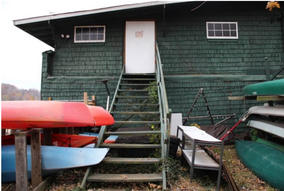
Stairs (ST04) at the east entrance.
