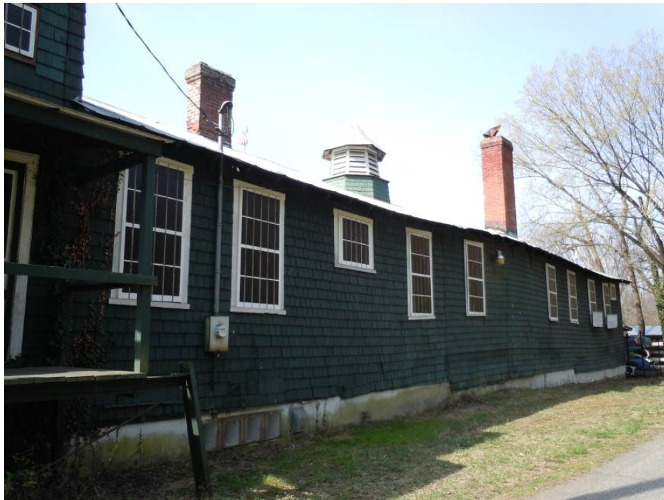
Wood shingle siding on the north elevation.
