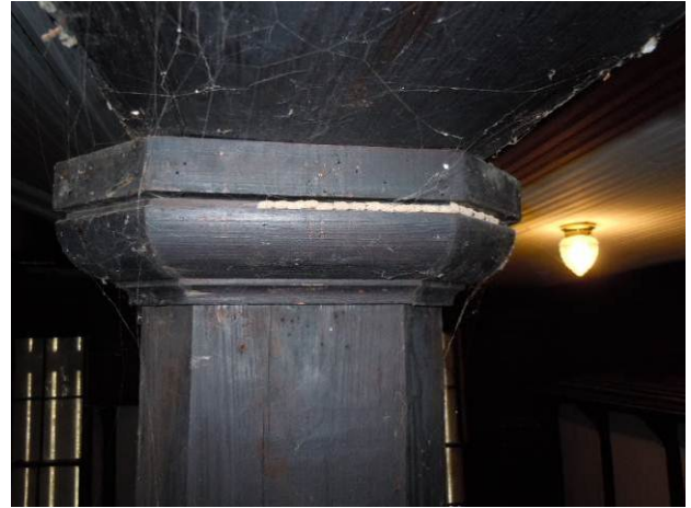
Simple bullnose trim on original interior columns in Ballroom. (HPTC photo)
