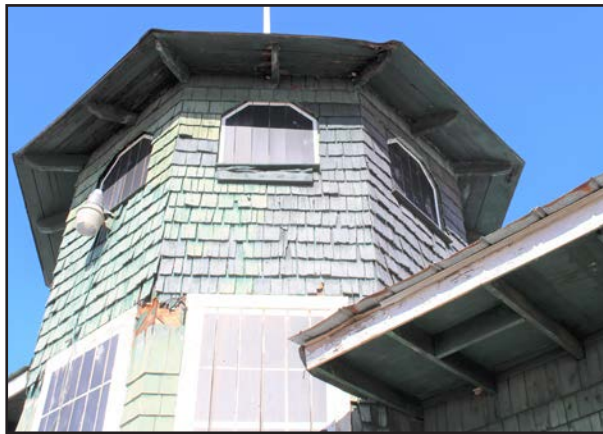
FIGURE 64 Soffit detail on east tower and east bay (right)
