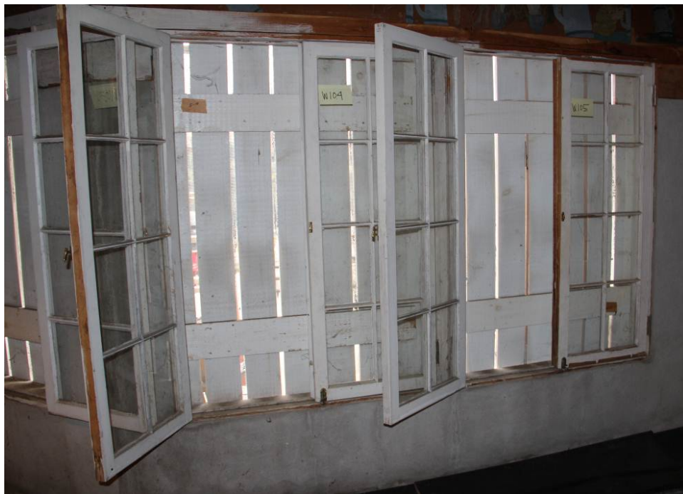
Interior view of Grill Room windows with one sash opened.
