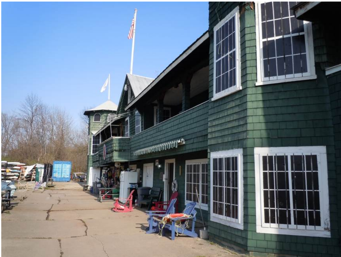
South elevation of the main block.
