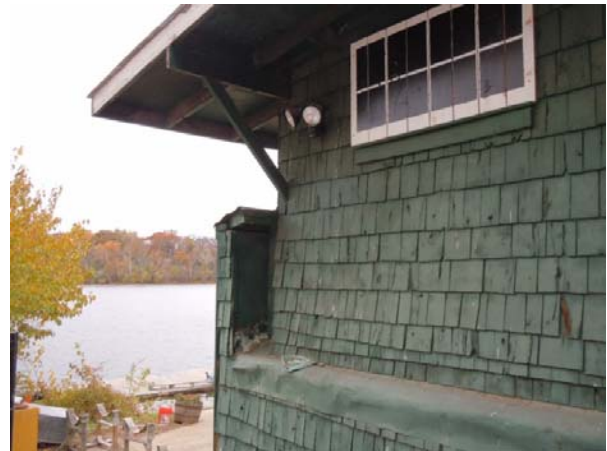
Detail of underside of soffit with roof frame exposed.
