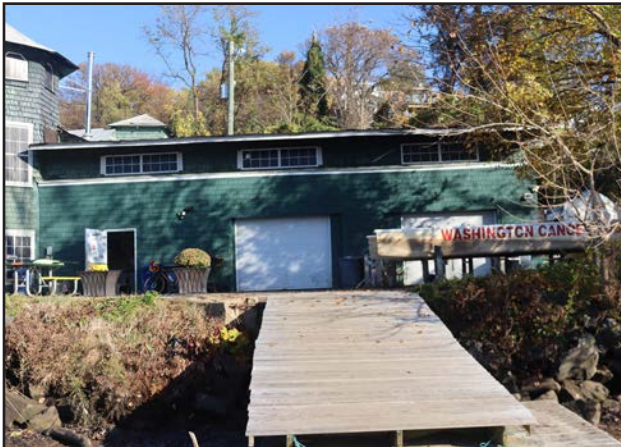
FIGURE 49 Newer shingles on south elevation of east bay.
