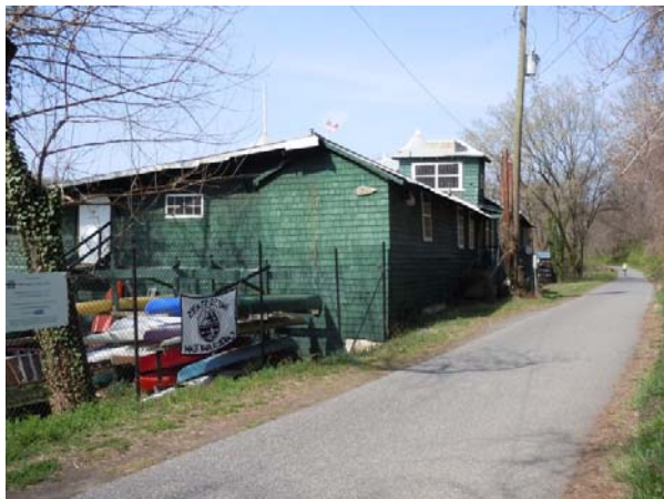
View from bike trail of the northeast corner showing the overlapping roofs of the Women's Locker Room and the Workshop.
