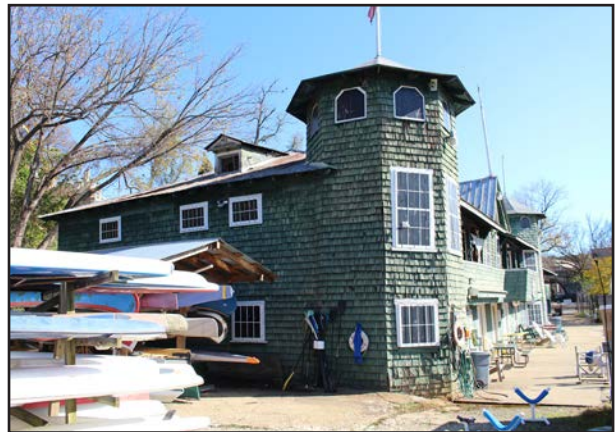
FIGURE 47 Obstructed west and south elevation, looking east.
