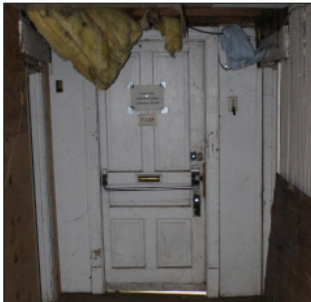
FIGURE 81 Interior of north entrance door with contemporary ADA hardware.
