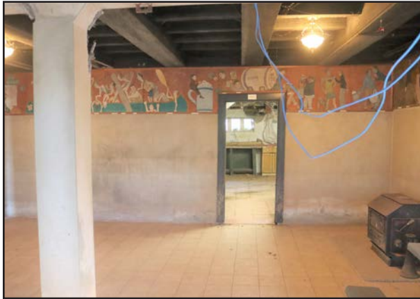
FIGURE 99 Grill Room, first floor, looking north.
