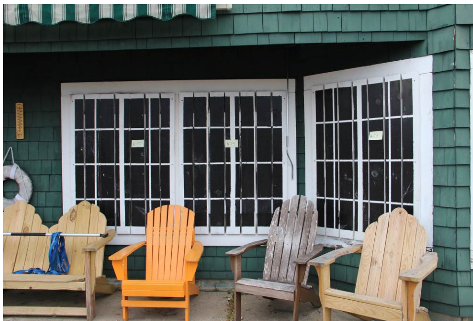
Exterior view of the first-floor windows on the south elevation of the main block. The windows are covered with painted wood planking and screening.
