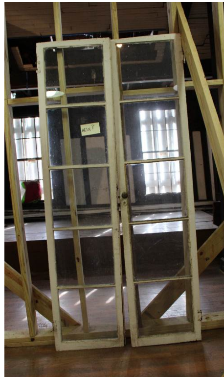
Exterior side of typical full-length double casement windows in the Ballroom.
