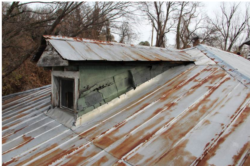
Dormer on the west slope of the main roof.
