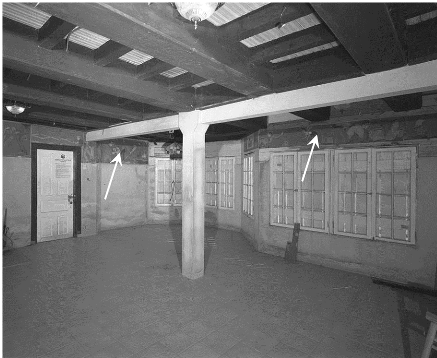
The Grill Room, or Common Room, on the first floor. The bay window, dropped beams, and window openings are character-defining features of this important space. A decorative painted mural (arrows), depicting highlights in the club's history is installed on the upper portion of the walls. (HABS photo)
