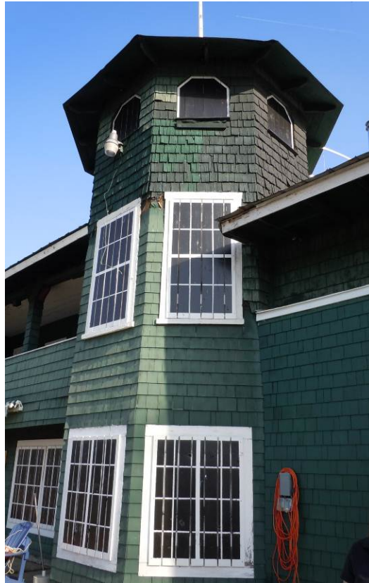
Typical window openings in the towers. The upper tower openings originally did not have window sashes but were open for viewing. (HPTC photo)
