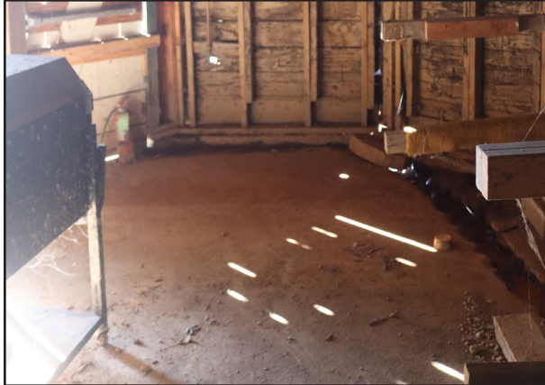
FIGURE 90 Concrete foundation with channel at the right hand side of the image.
