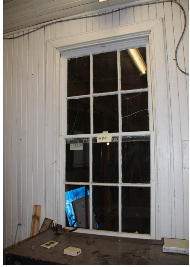
View of window W241 from North Entrance Hall (Room 209).
