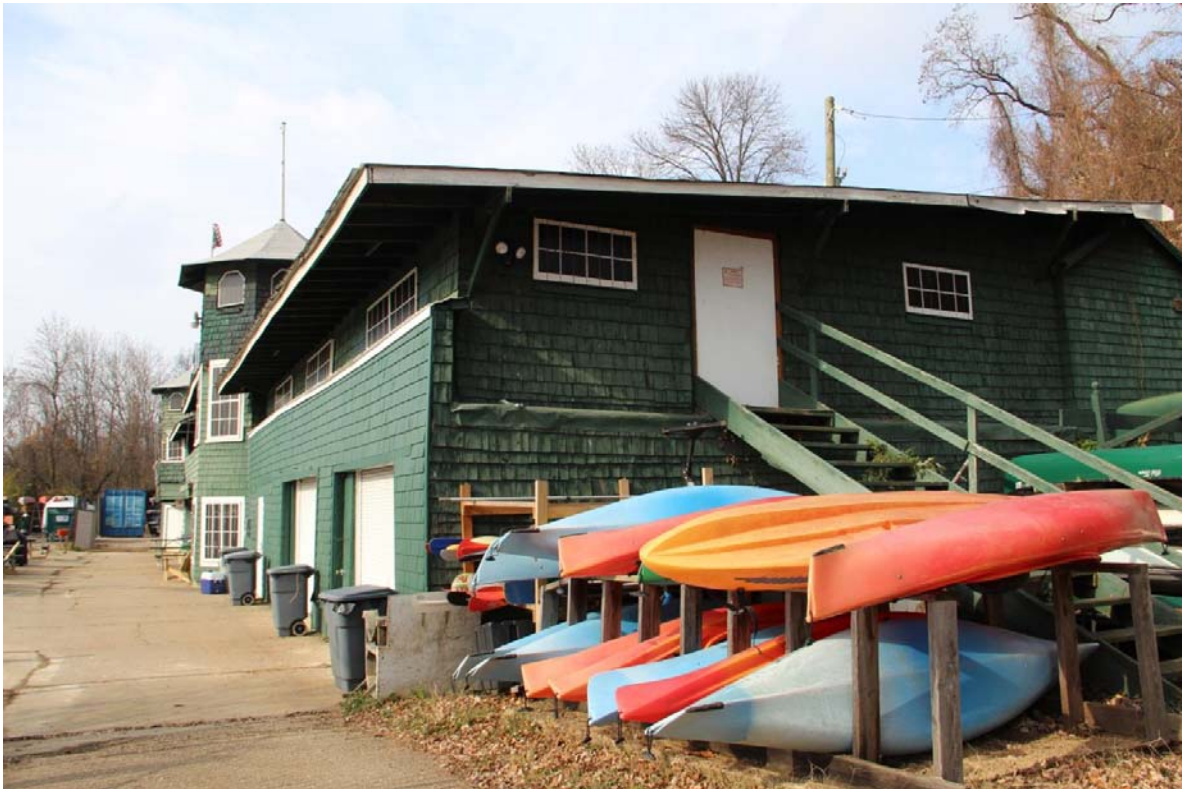
This roof overhangs the exterior walls on the south and east elevations. It is supported by the lightweight roof frame and plywood roof deck. There is a vertical fascia board on both elevations. Materials in generally fair condition.
