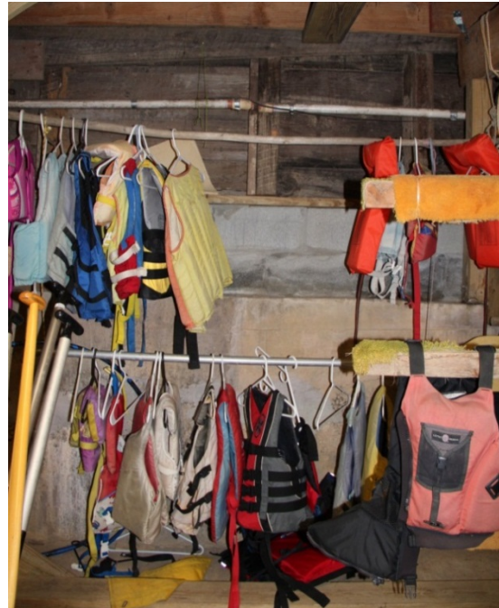
View of north wall in east addition area showing CIP surmounted by CM and north exterior wood frame wall.
