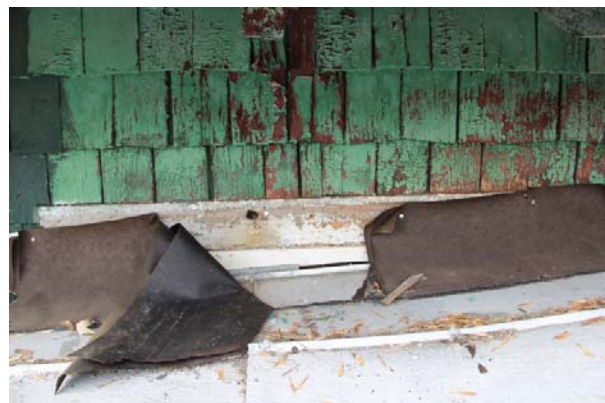
Detail of east elevation under main house roof overhang.
