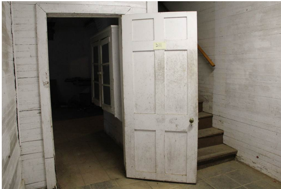
Original 6-panel door (D111) with original hardware.
