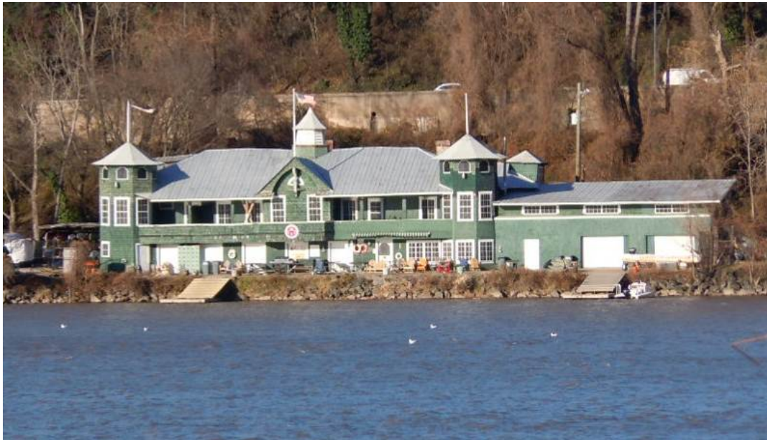
Overall current view of the south elevation of the canoe club building with green siding and white trim.
