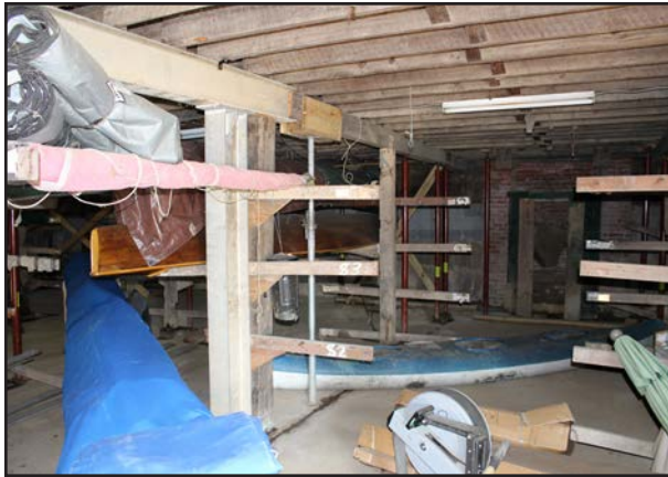
FIGURE 101 West Boat Storage Area, first floor, looking north.
