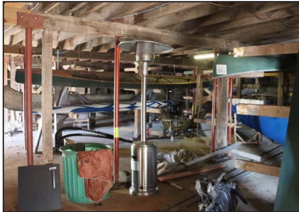
FIGURE 86 Temporary pipe columns installed in West Boat Storage Area.
