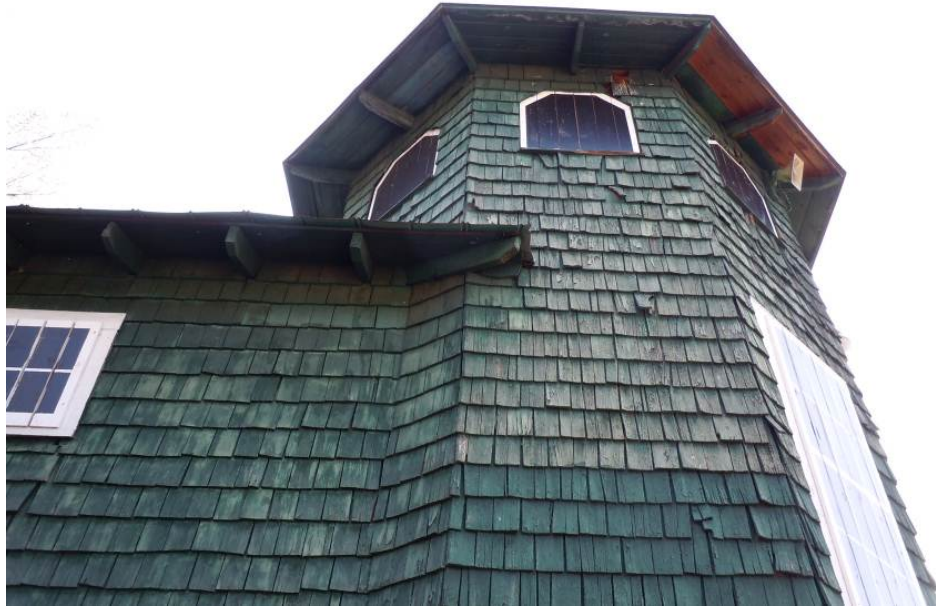
Weathered shingles on the west elevation of the west tower.
