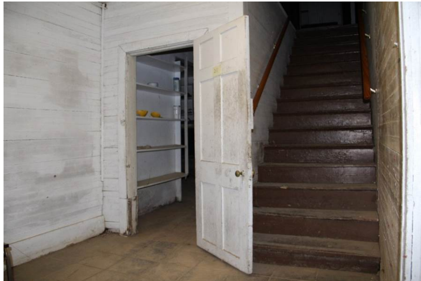
Stairs (ST02) in the first floor hall (Room 104) leading to the second floor hall (Room 207).
