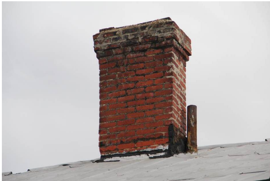
East brick chimney with corbelled top courses. (HPTC photo)
