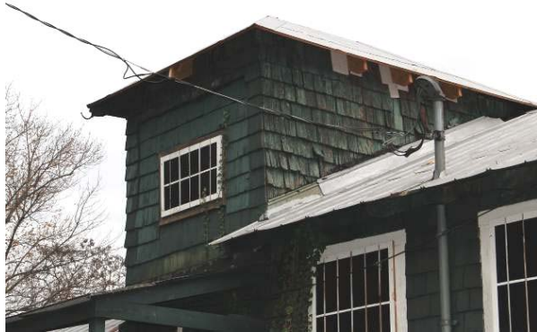
Shingle siding on the northwest elevation of the north tower.
