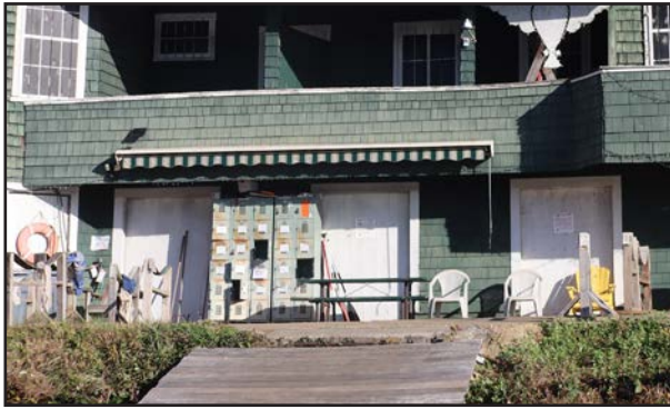
FIGURE 84 Non-original exterior door in the West Boat Storage Area.
