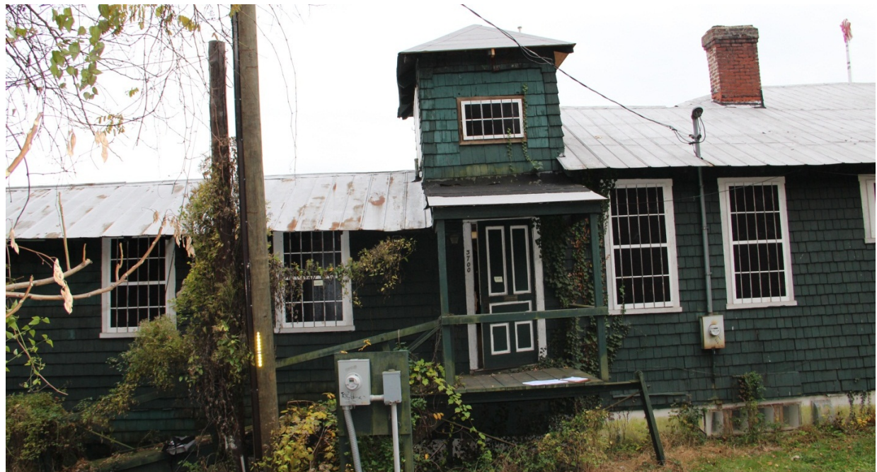
North elevation of the North Tower and shed roof over the north entrance below.
