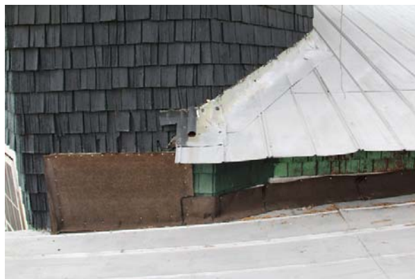
Detail of east elevation at East Tower.
