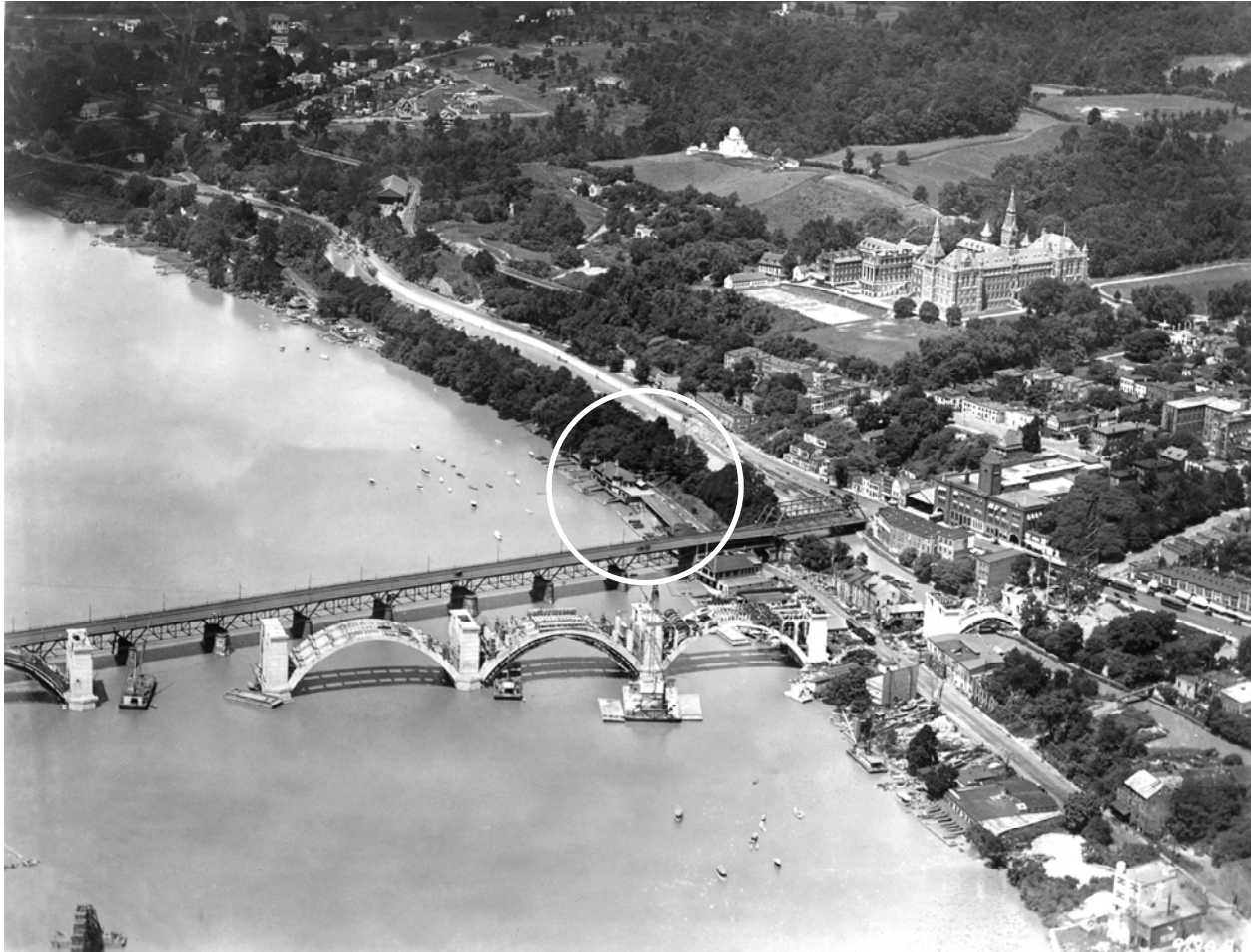
Overview of the arches of the Key Bridge under construction (n.d.). The old Aqueduct Bridge is just north of the arches with Georgetown University visible in the upper right and the Washington Canoe Club building just north of the Aqueduct Bridge on the shoreline (circled). (Office of History, US Army Corps of Engineers, Alexandria, VA; Capital Engineers, page 203)
