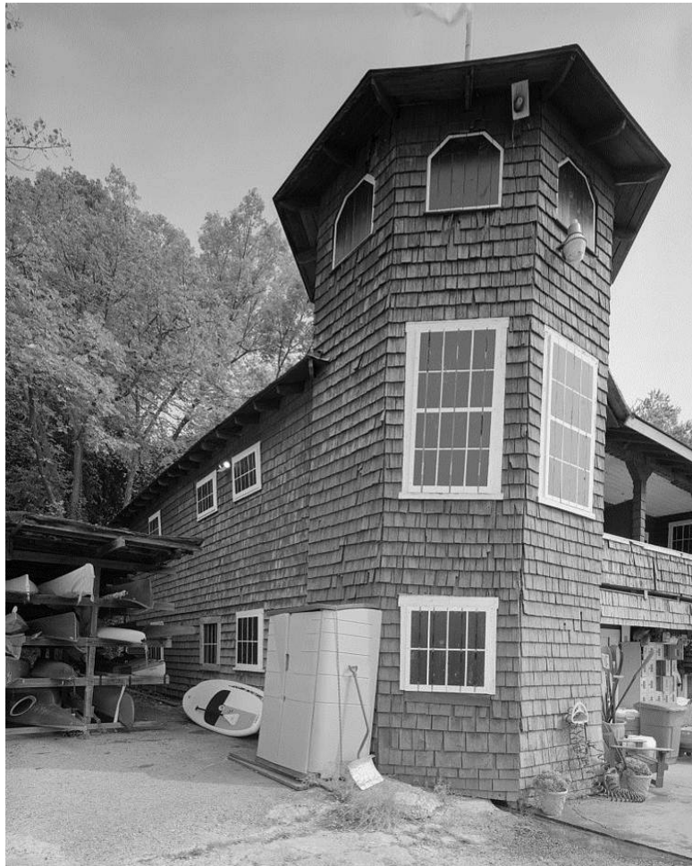
West elevation and west tower. (HABS photo)
