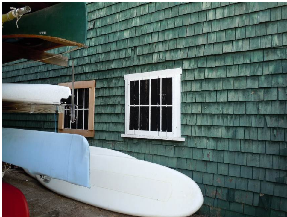
Painted wood shingle siding on the west elevation.
