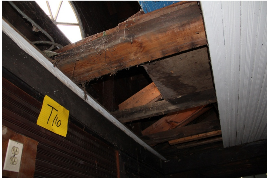
Task 16. Outcome – ceiling structure and roof frame structure exposed.
