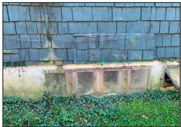
FIGURE 71 Acrylic panel covering Kitchen window.
