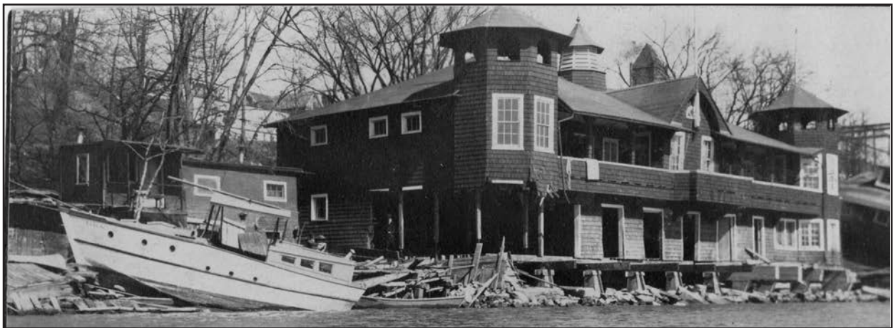
FIGURE 21 The west boat storage area sustained significant damage after a motor boat drove into the building during a flooding event, n.d. Brown, Washington Canoe Club .
