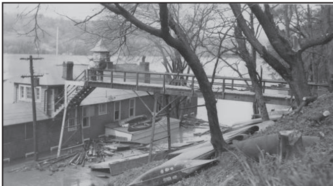
FIGURE 19 Catwalk bridge leading from C&O Canal towpath to entrance within tower at the north elevation, looking southwest, 1936. The elevated entrance comprised of double wood-panel doors with glazing. Note attached shed off of the northern elevation, as well as the openings at the first story level. Also note that by this time, the roof shingles had been replaced with some sort of composite. William "Dusty" Rhodes family
