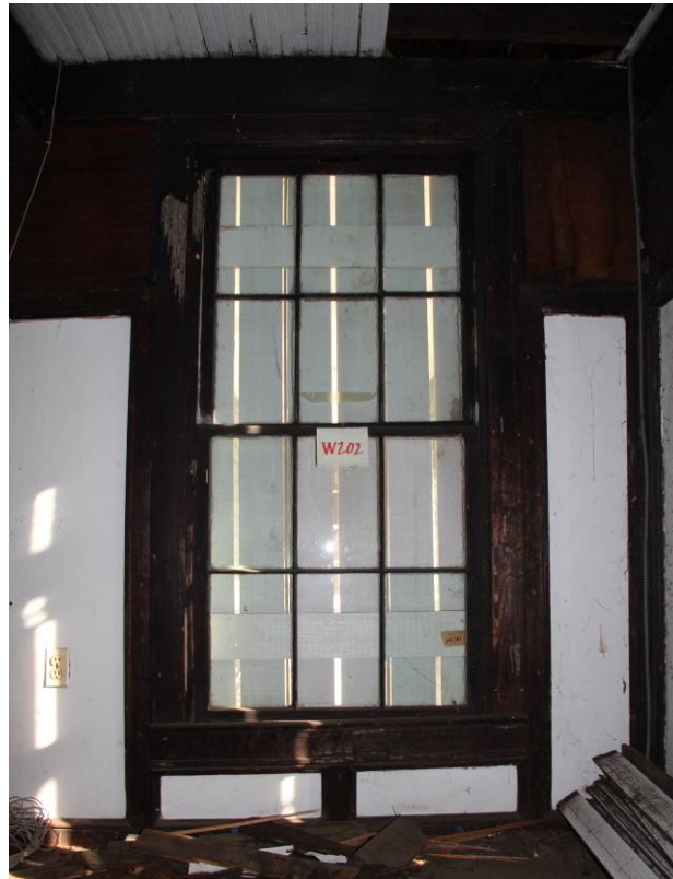
Original 6-over-6 double-hung window with original hardware. (HPTC photo)
