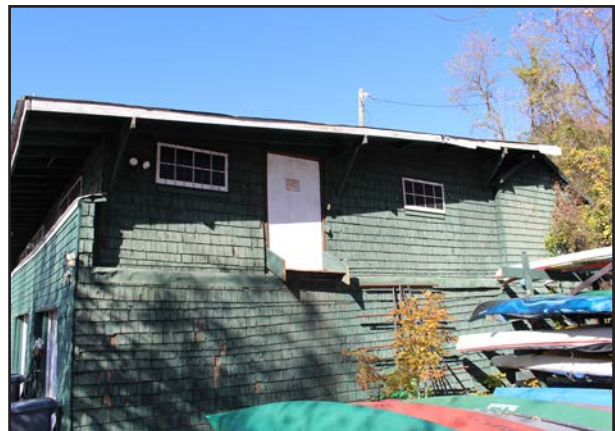
FIGURE 45 East and partial south elevation of c. 1920s addition, looking west.
