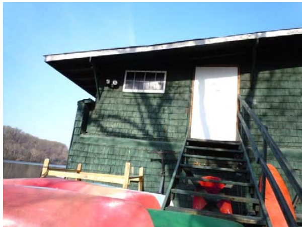
Southeast corner of EBSA with overhanging roof soffit.
