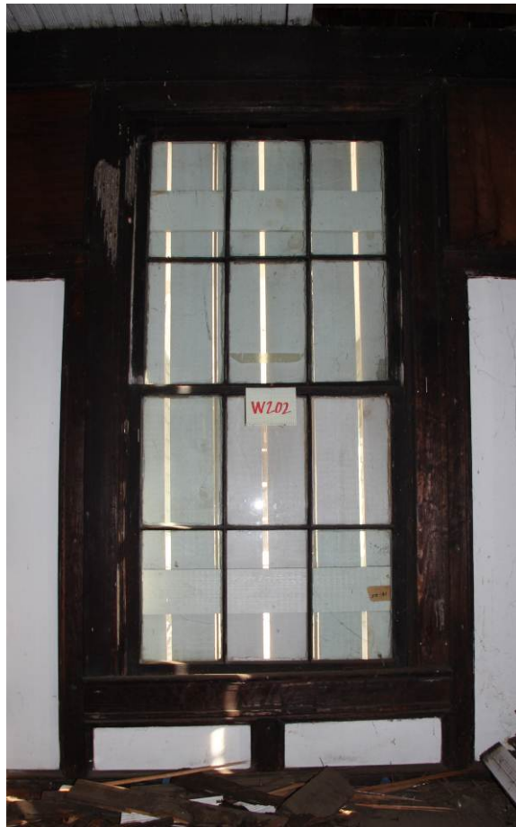
Typical double-hung wood window located in the Ballroom (Room 201).
