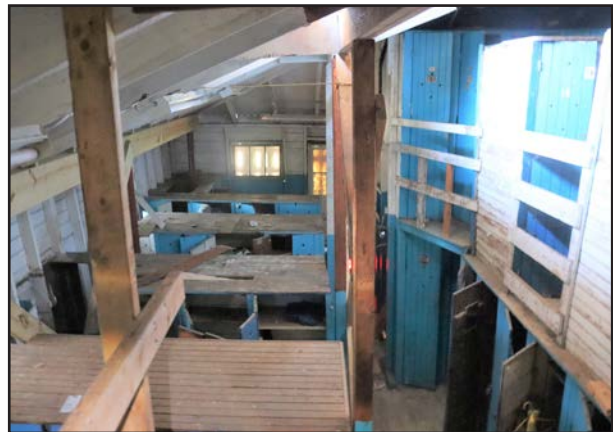
FIGURE 110 Men's Locker Room, second floor and mezzanine, looking north.
