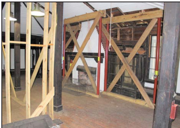
FIGURE 109 Ballroom, second floor, looking northwest.
