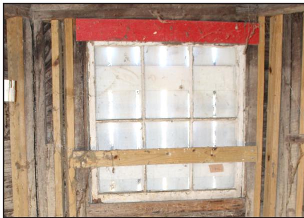
FIGURE 70 Detail of window in West Boat Storage Area.
