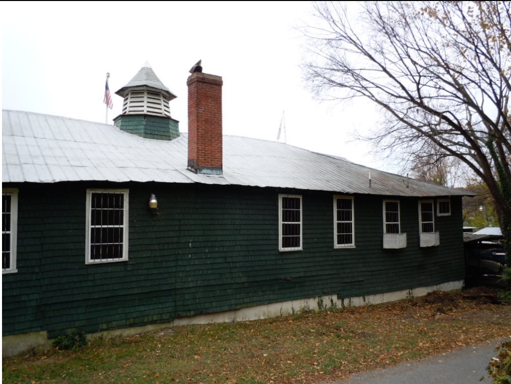
Typical window openings on the north elevation are covered with spaced wood panels painted to mimic window sashes but indicate relative position of window openings in the Men's and Women's Locker Rooms. (HPTC photo)
