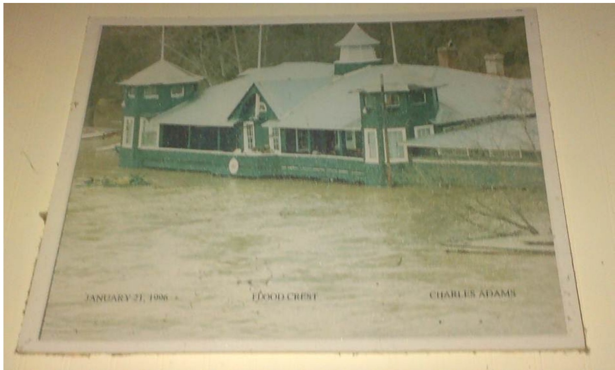
Flood Crest of January 21, 1996, by Charles Adams, found on the wall at the DC Boat House Restaurant. Clearly indicates flood waters inundating the ground floor of the Canoe Club building. Building appears much as it does today (2014).
