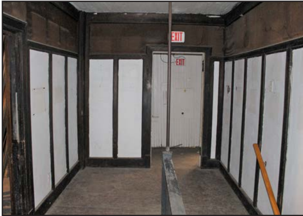
FIGURE 105 Central Hallway, second floor, looking east.
