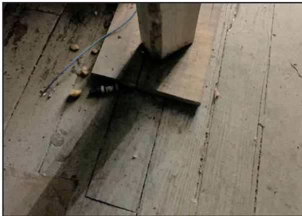
FIGURE 116 Wood plank flooring in Men's Locker Room.
