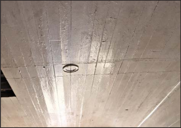
FIGURE 120 Painted bead board, first floor.
