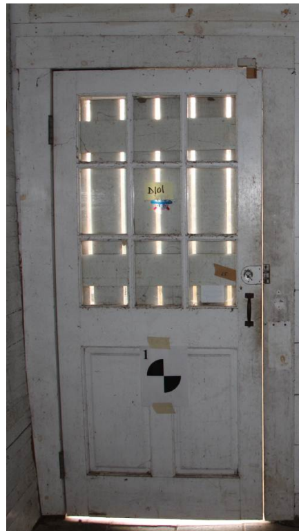
Interior view of door (D101).
