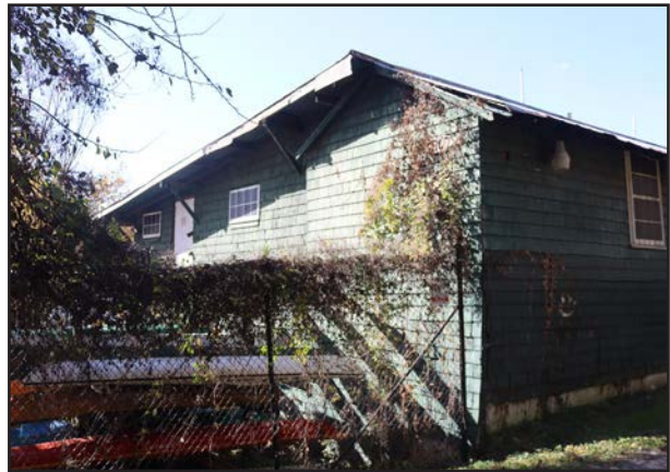
FIGURE 63 Shed roof enclosure of southern portion of East Storage Bay overlapping gable roof of Ladies Locker Room.
