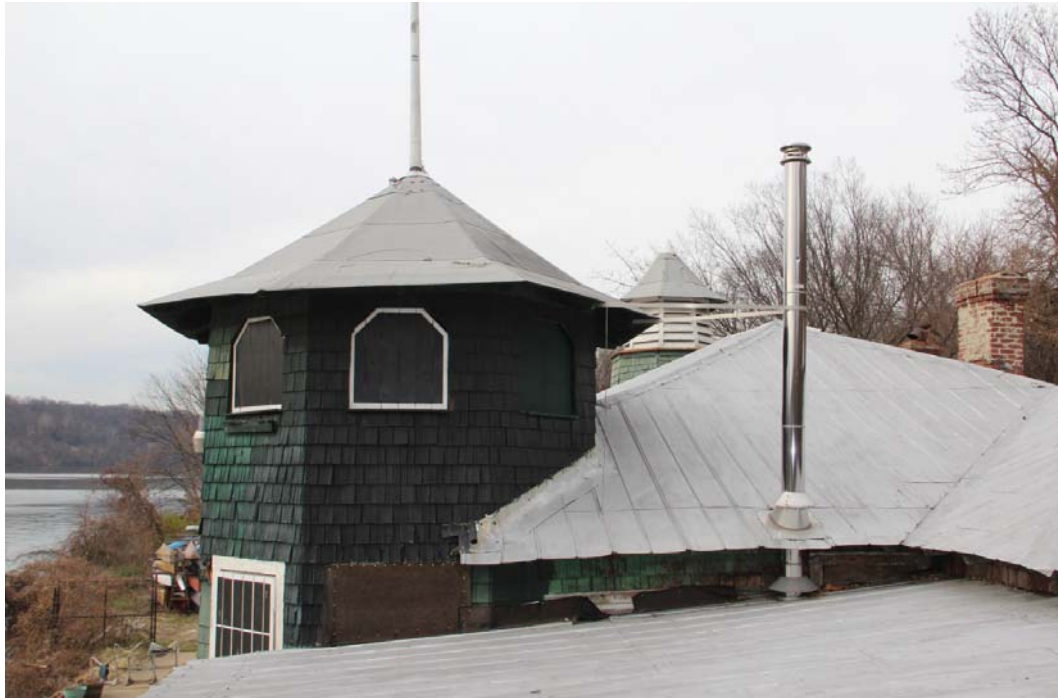
Intersection of Workshop shed roof with east elevation of East Tower. Former window location in East Tower is covered with solid panel.
