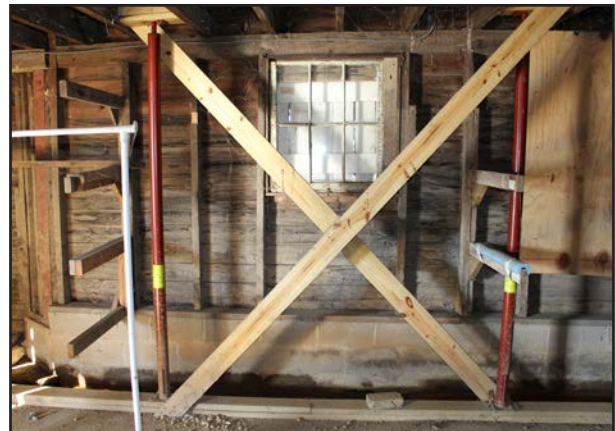
FIGURE 87 Cross bracing in West Boat Storage Area.
