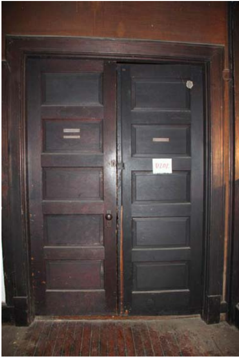
Double 5-panel doors (D202) leading from the Hall (Room 207) on the second floor into the Board Room (Room 208).
