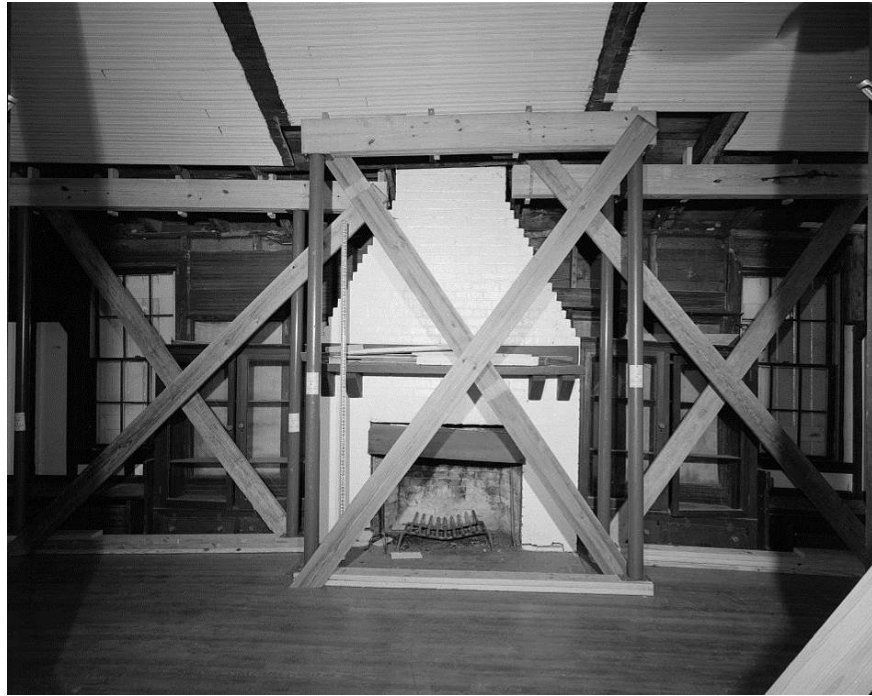
Corbelled brick fireplace and wood mantle in the Ballroom. (HABS photo)
