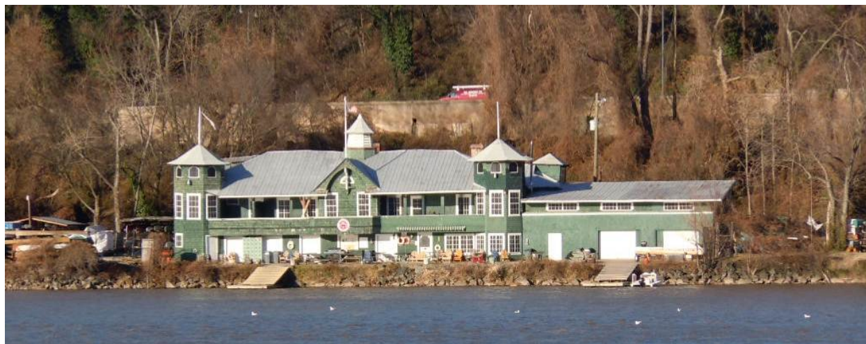
View of river (south) elevation. (12/31/13, HPTC)
