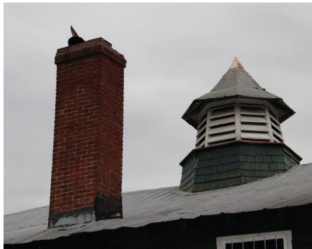
Red brick laid in common bond is an exterior material used to construct the two extant chimneys on the north roof slope. (HPTC photo)
