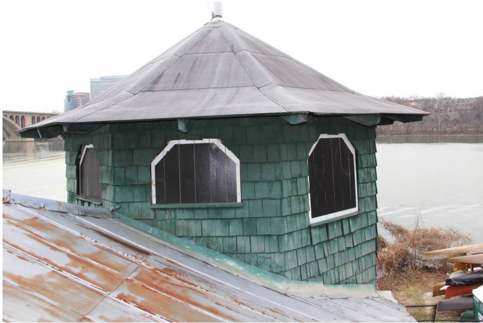
Exterior view the window openings in the West Tower Chamber (Room 302). Note the smaller size of the window openings facing the roof.
