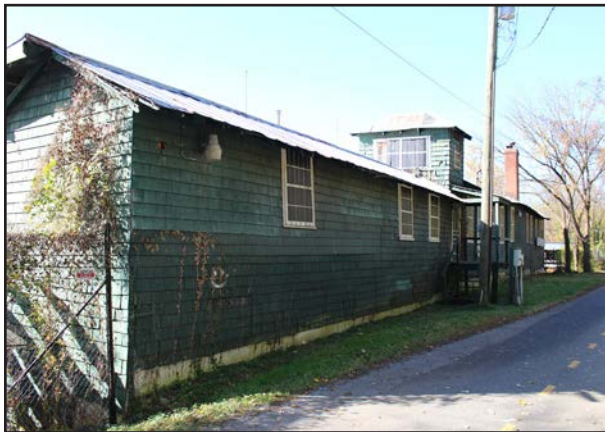
FIGURE 46 North and partial east elevation, looking west.
