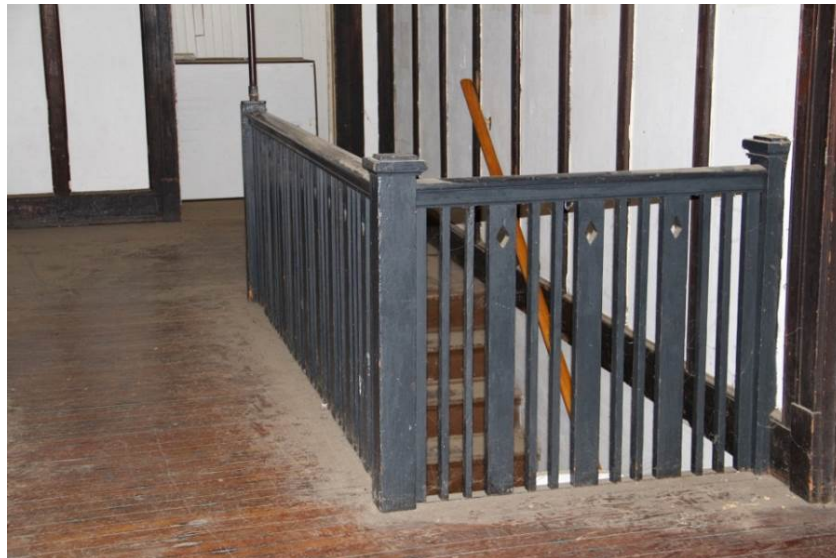
Balustrade surrounding the main stairs (ST02) on the second floor.
