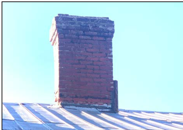
FIGURE 69 North side of chimney that serves the ballroom..
