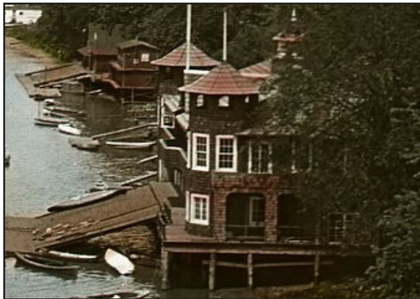
FIGURE 60 Washington Canoe Club, looking west, c. 1910-1920. The building's original roof likely featured wood shingles. By the 1910s, however, the roofing comprised of either sheet metal pans or some type of synthetic asbestos-cement shingle (widely available after 1920). Washington Canoe Club Historic Structure Assessment Report.
