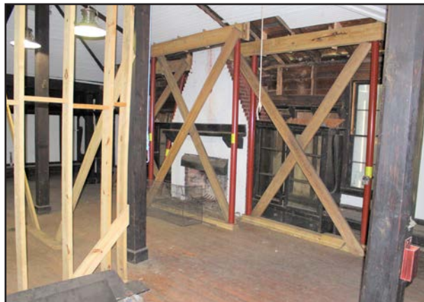
FIGURE 88 Bracing in the Ballroom.
