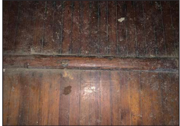
FIGURE 115 Wood floor, second floor.
