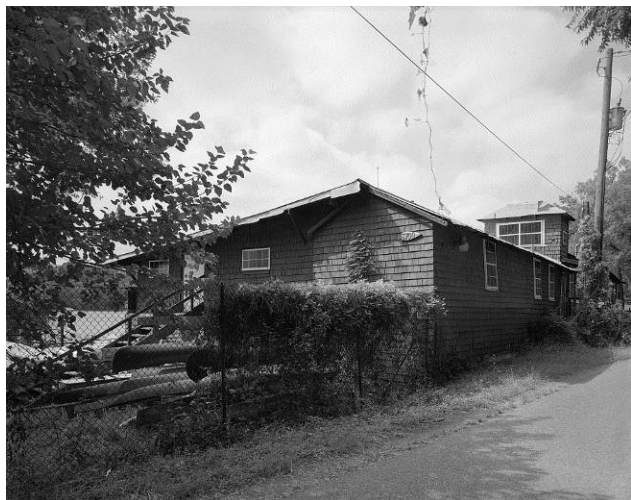
Northeast elevation. (HABS photo)
