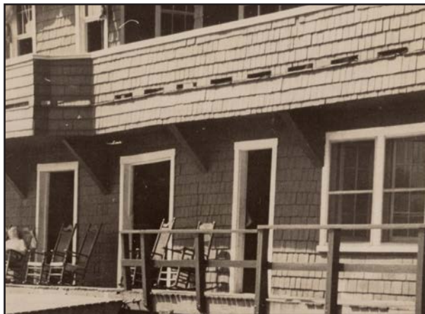
FIGURE 57 Detail of brackets under balcony, looking northwest, c. 1950s. Washington Canoe Club.
