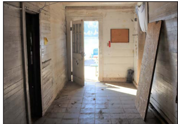
FIGURE 104 Central Hallway, first floor, looking south.
