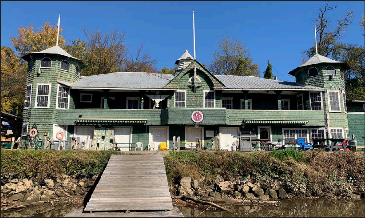
FIGURE 01 Washington Canoe Club, south elevation, looking north from dock.
