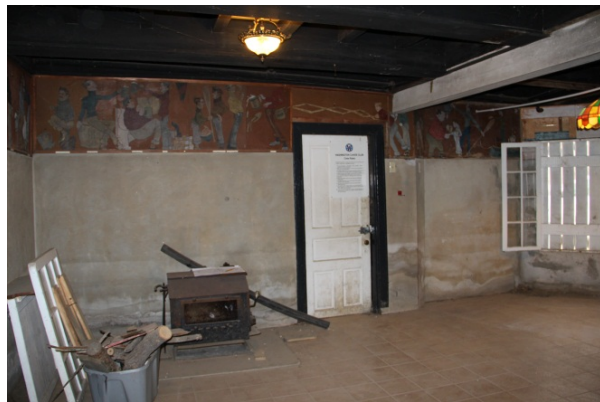
View of extant wood stove in Grill Room with dismantled stove pipe (11/22/13 HPTC).
