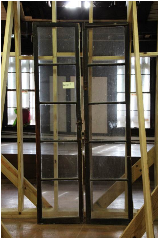
Interior side of typical full-length double casement windows in the Ballroom.
