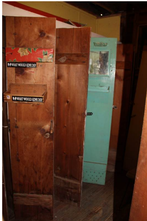
Vertical T&G lockers in the Women's Locker Room. (HPTC photo)
