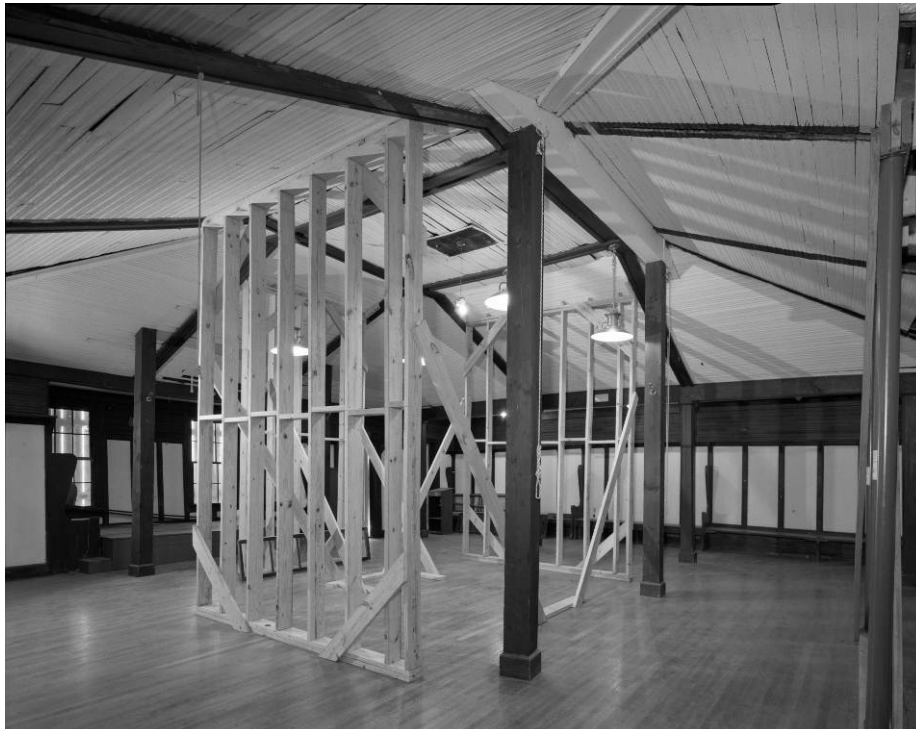
Interior hipped ceiling with bead-board wood strip finish at Ballroom. The large unobstructed open space of this room is a character-defining feature (although currently obscured by the temporary supports). HABS 876-020.
