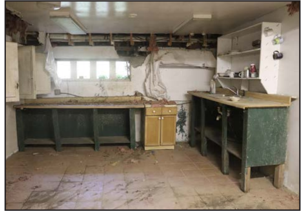
FIGURE 100 Kitchen, first floor, looking north.
