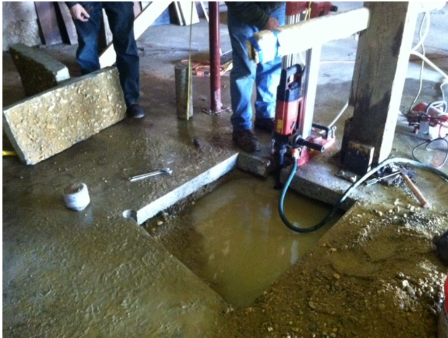
Task 12: Overview or saw cutting of slab area 1.
