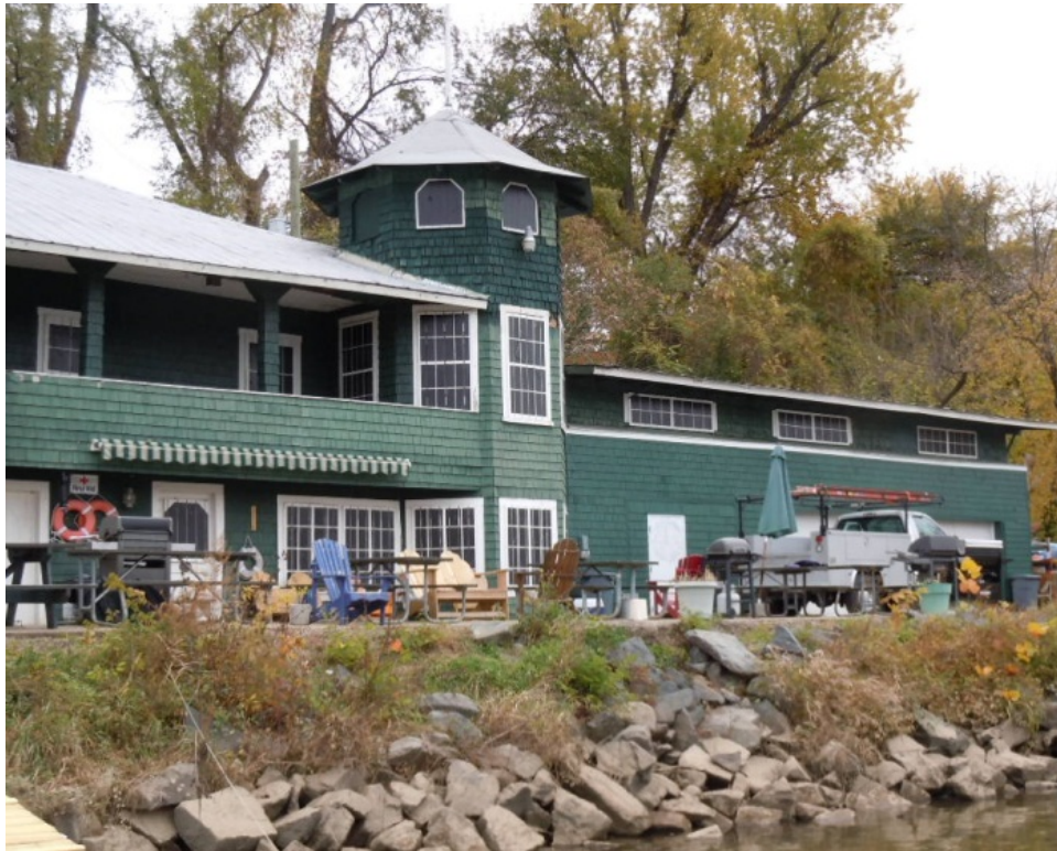
South elevation of EBSA with recessed south elevation and triple paired awning windows into boat work room area.
