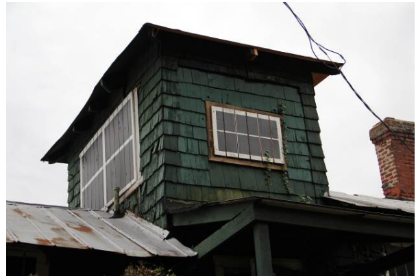
Shingle siding on the northeast elevation of the north tower.
