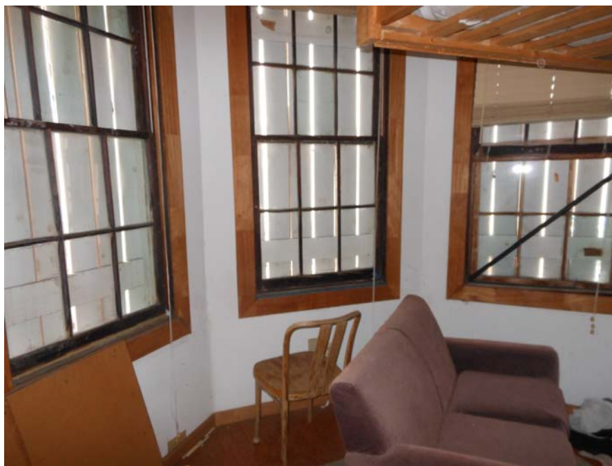
The West Tower Lower Chamber (Room 202) has 6-over-6 double-hung wood windows.
