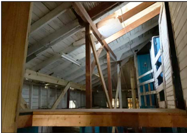
FIGURE 93 Framing in men's locker room.
