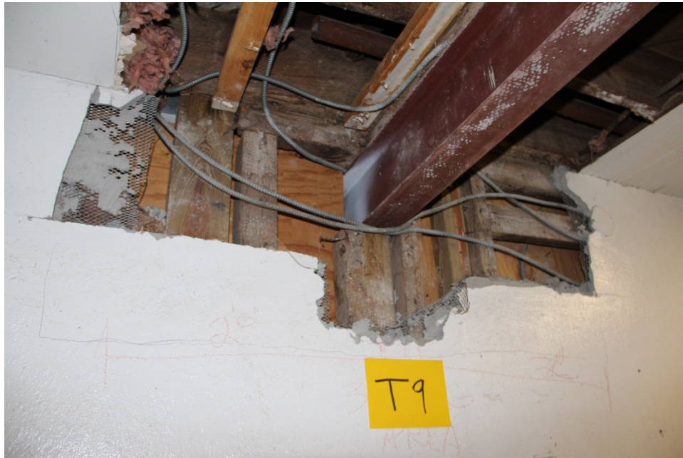
Task 9 Outcome: steel beam connection with wood wall frame revealed.
