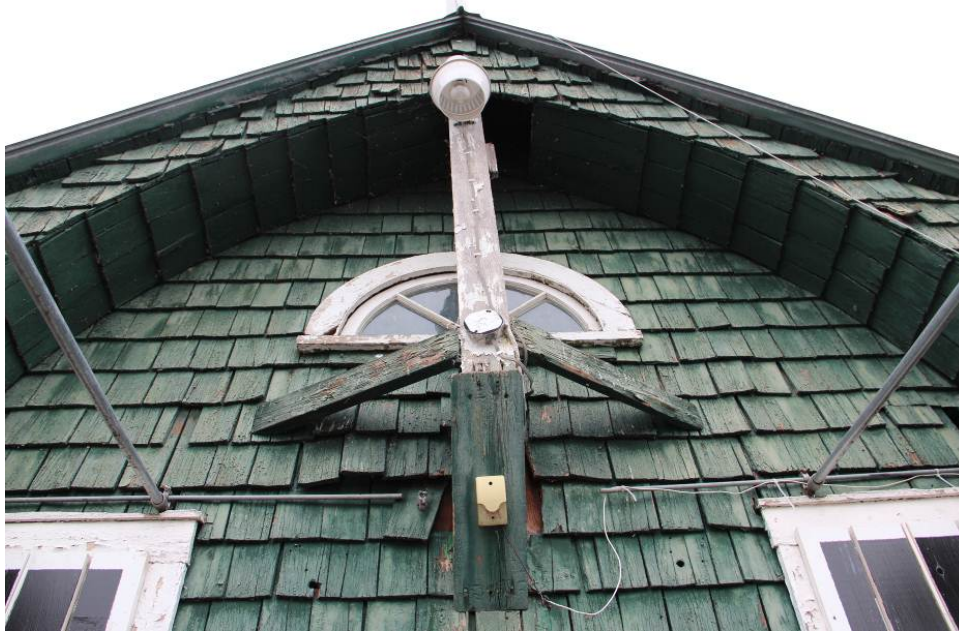
Exterior view of the fan window (W321) in the south gable.
