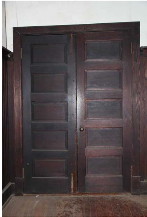
View of doors (D202) from the Board Room (Room 208).
