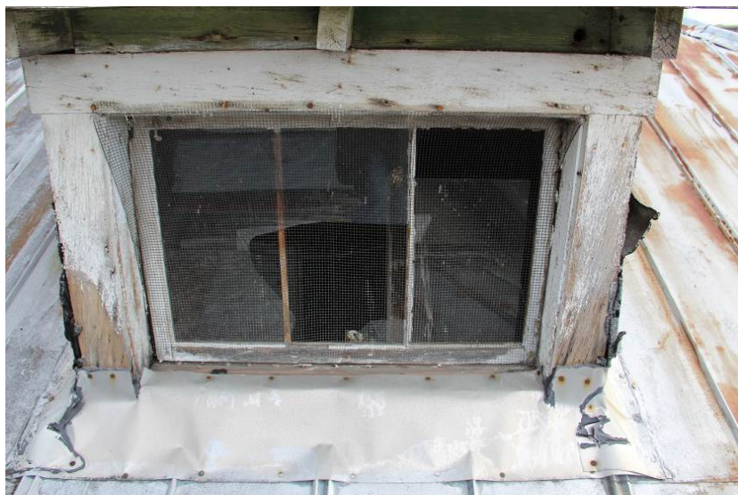
Window (W320) in the west dormer.
