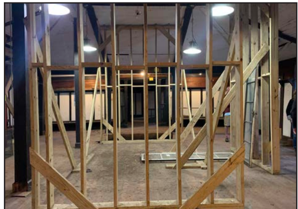
FIGURE 89 Bracing in Ballroom.
