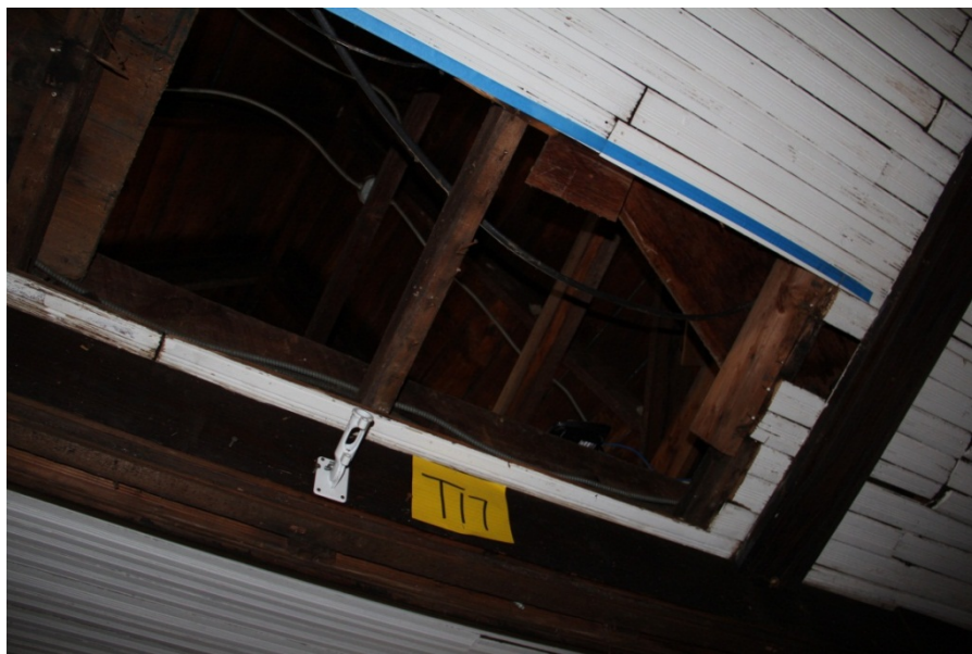
Task 17. Outcome: sample successfully removed, ceiling structure exposed.
