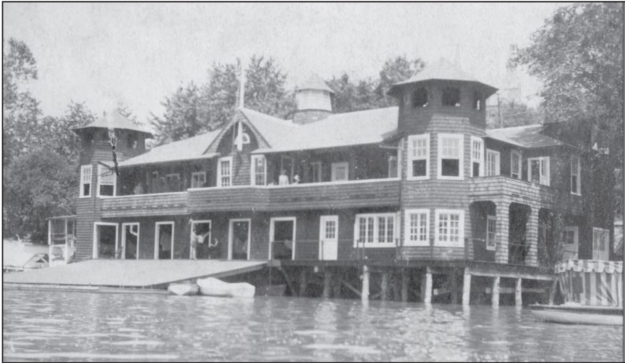
FIGURE 18 The WCC boathouse as it appeared after completion of the second construction phase c. 1910. Downspouts visible on the east and west ends of the balcony, and rectangular drainage holes ran across the balconies. Washington Canoe Club.
