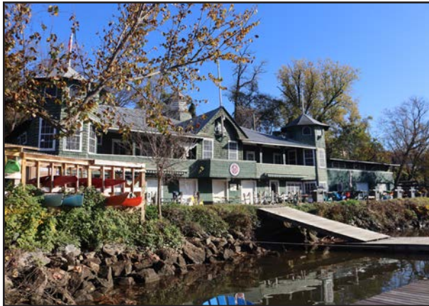
FIGURE 44 Partially obstructed south elevation, looking northeast.
