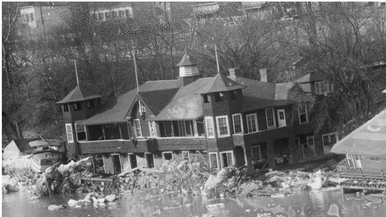
Image enlarged from Potomac Flood, Georgetown, D.C.; LOC Call Number: LC-F81-44573, undated. Thought to be the same flood event as depicted in ca. 1918 image. Clearly illustrated the east elevation of the building prior to any additions.
