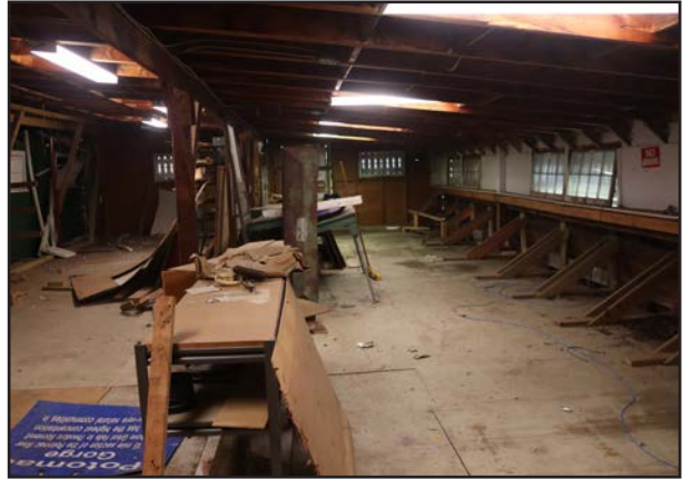
FIGURE 106 Workroom, second floor, looking east.
