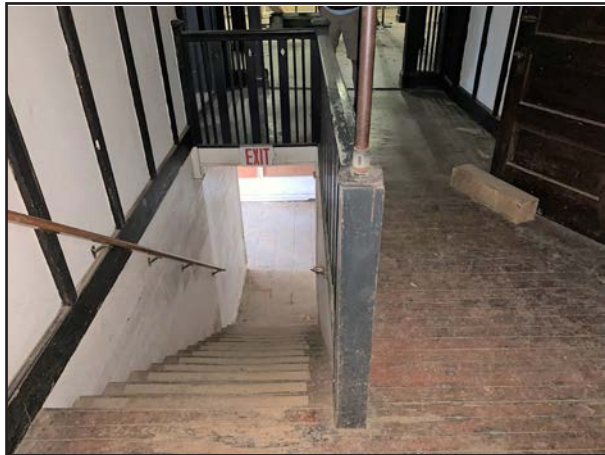
FIGURE 111 Main staircase, looking west.
