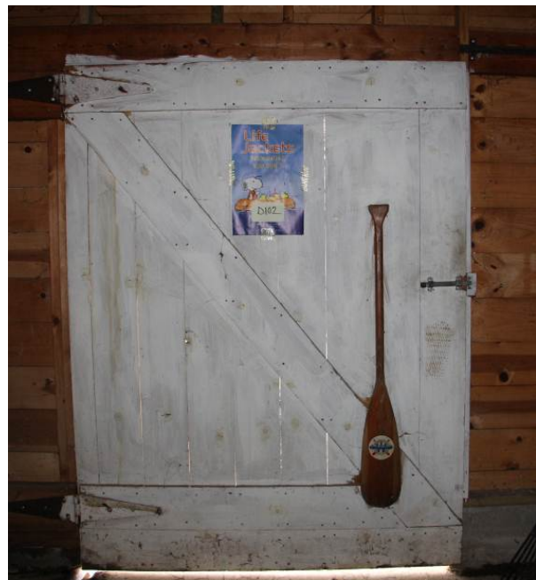
Interior view of door (D102).
