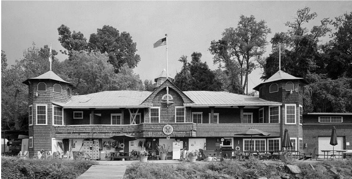
Gable roof over the central bay and octagonal roofs over the flanking towers. Note the flagpoles on each of the towers and the central gable roof. Sheet metal roofing provides a vertically oriented pattern that is not in keeping with the American Shingle Style of the building. (HABS photo)
