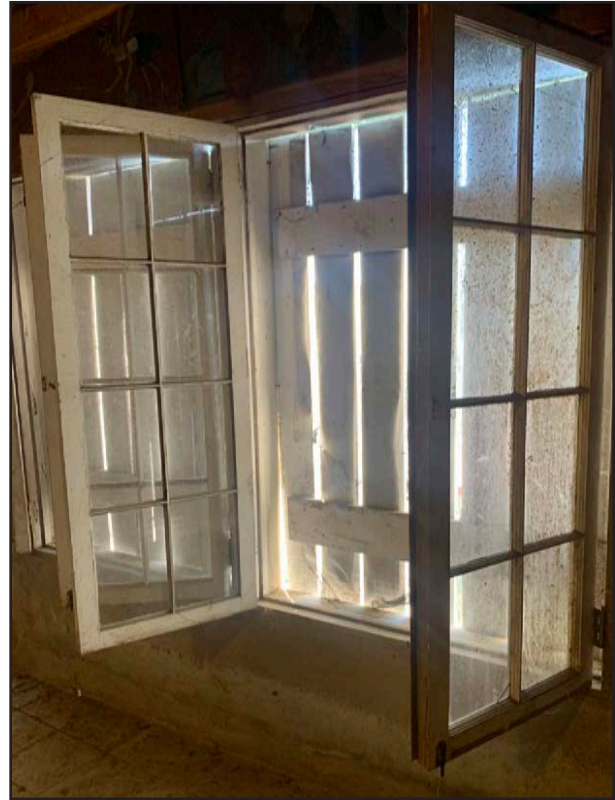
FIGURE 72 Windows in Grill Room, looking south. Windows are in fair condition.
