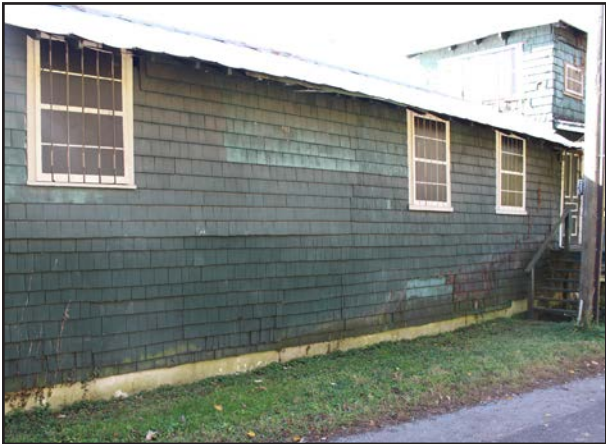
FIGURE 50 Wood shingle siding on north elevation
