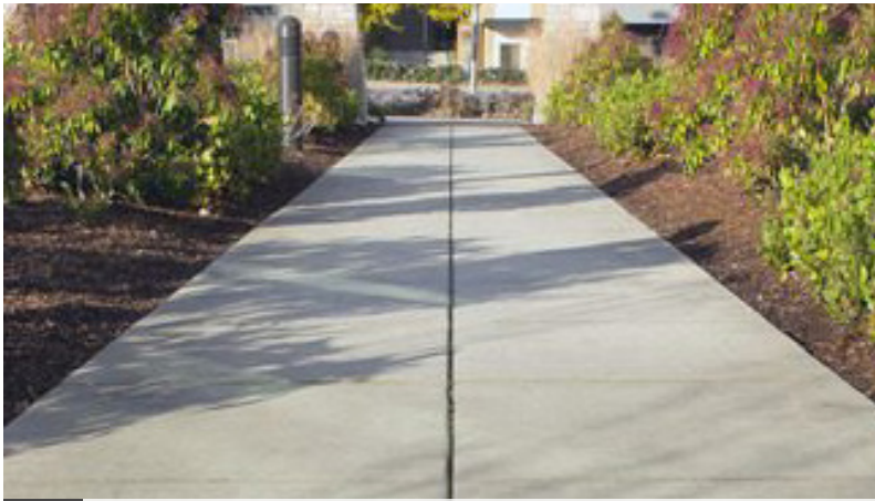
1 PEDESTRIAN CONCRETE BROOM FINISHED SIDEWALK
