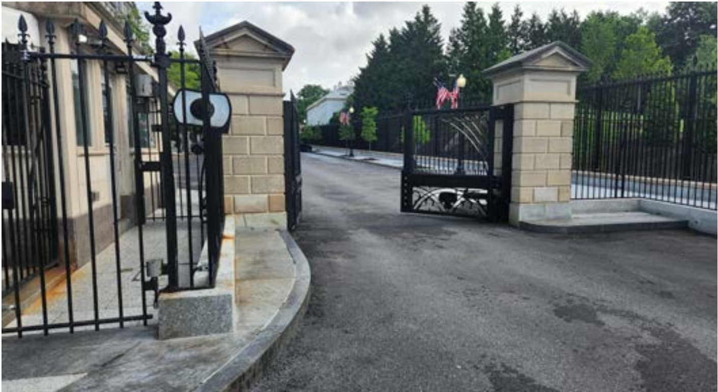
VIEW OF EXISTING VEHICLE AND PEDESTRIAN GATES, LOOKING NORTH FROM STATE PLACE. TEMPORARY SPIKES TO BE ADDED TO EXISTING FENCE AND GATES TOP RAIL.
