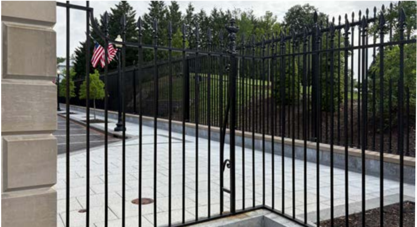
DETAIL OF EXISTING DECORATIVE METAL FENCE WITH FLEUR-DE-LIS FINIALS. TEMPORARY SPIKES TO BE ADDED TO EXISTING FENCE TOP RAIL
