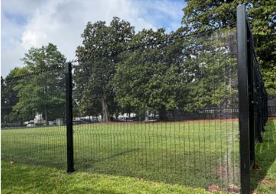
TEMPORARY ANTI-CLIMB MESH FENCE, INSTALLED AT EEOB FALL 2024. PROPOSED FENCE WILL MATCH, BUT WILL BE SUPPORTED BY ABOVE-GRADE BALLASTS TO AVOID DAMAGE TO PAVEMENT.
