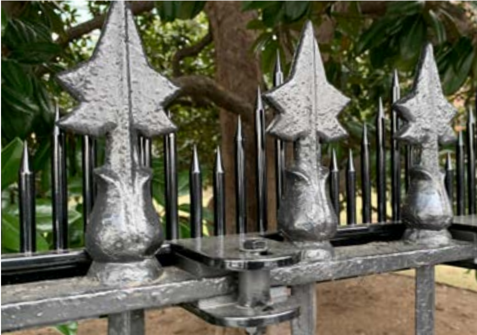
VARIABLE HEIGHT SPIKES TEMPORARILY ATTACHED TO DECORATIVE METAL FENCE, INSTALLED AT EEOB FALL 2024.
