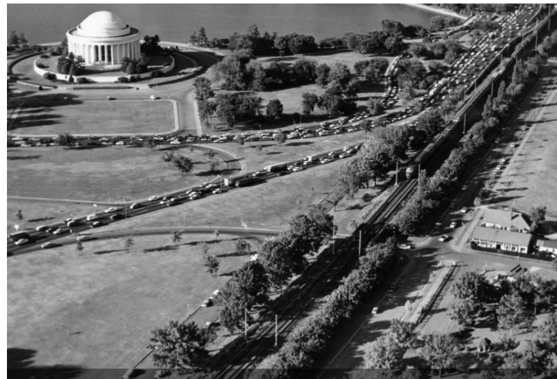
Historic Image of 14 th Street and Long Bridge Rail Corridor With Landscape Screening
