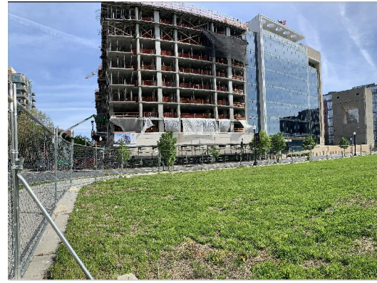
P 12 SITE PHOTO
