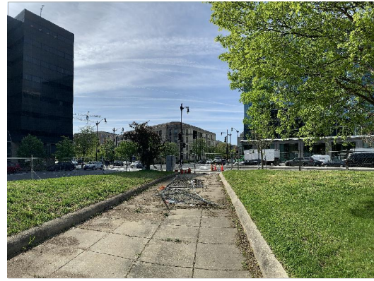
P 2 SITE PHOTO
