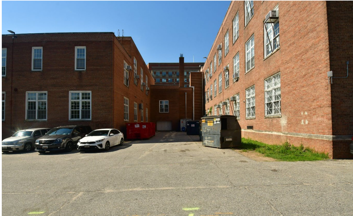
Existing exterior service courtyard
