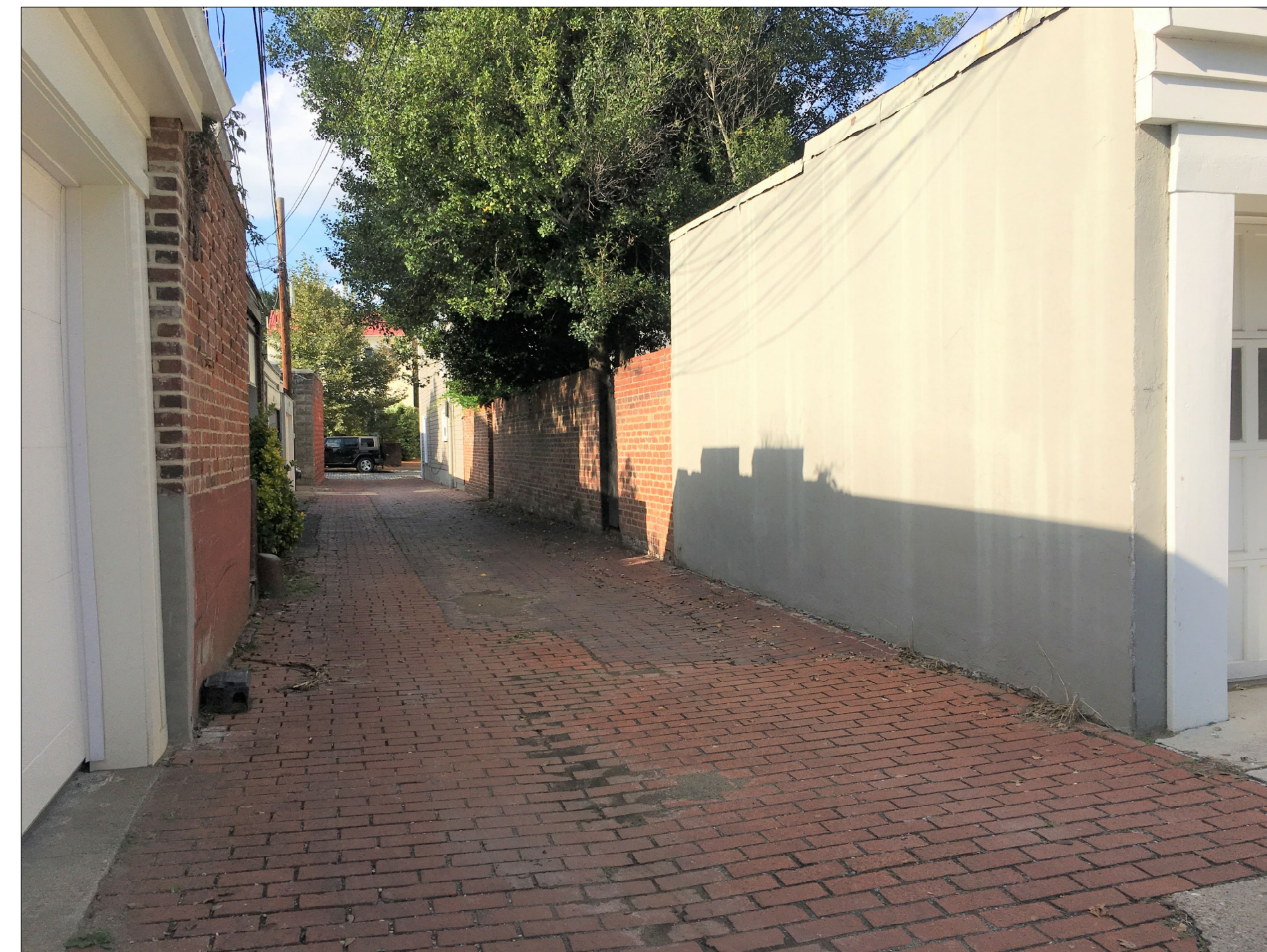
Alley View - 2 Toward P Street NW
