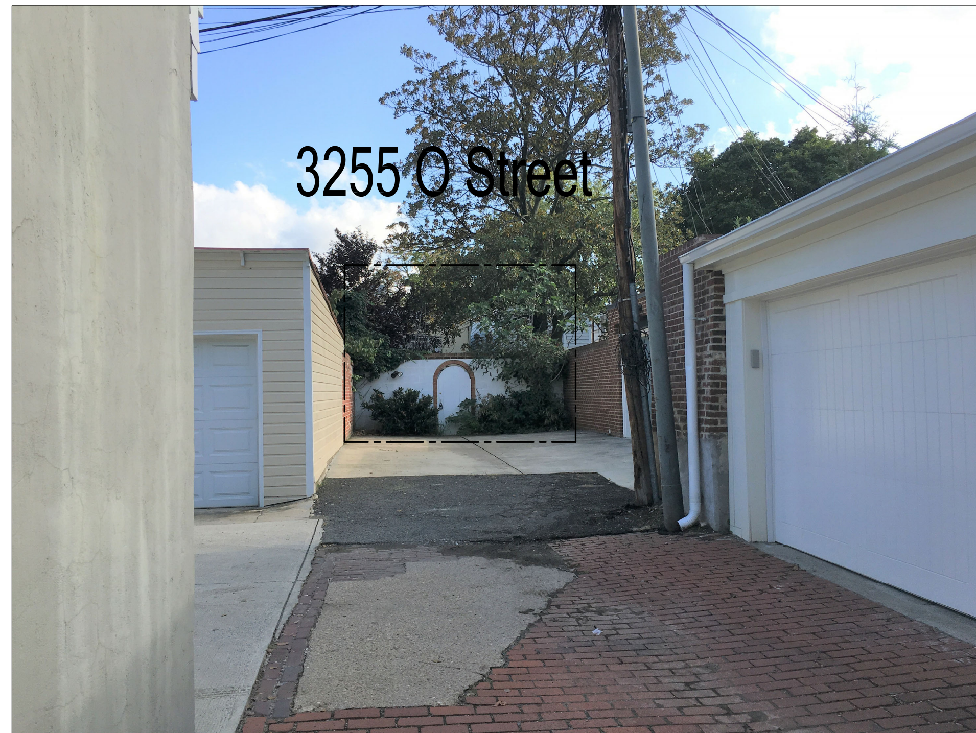
Alley View - 1 Toward Rear of 3255 O Street NW
