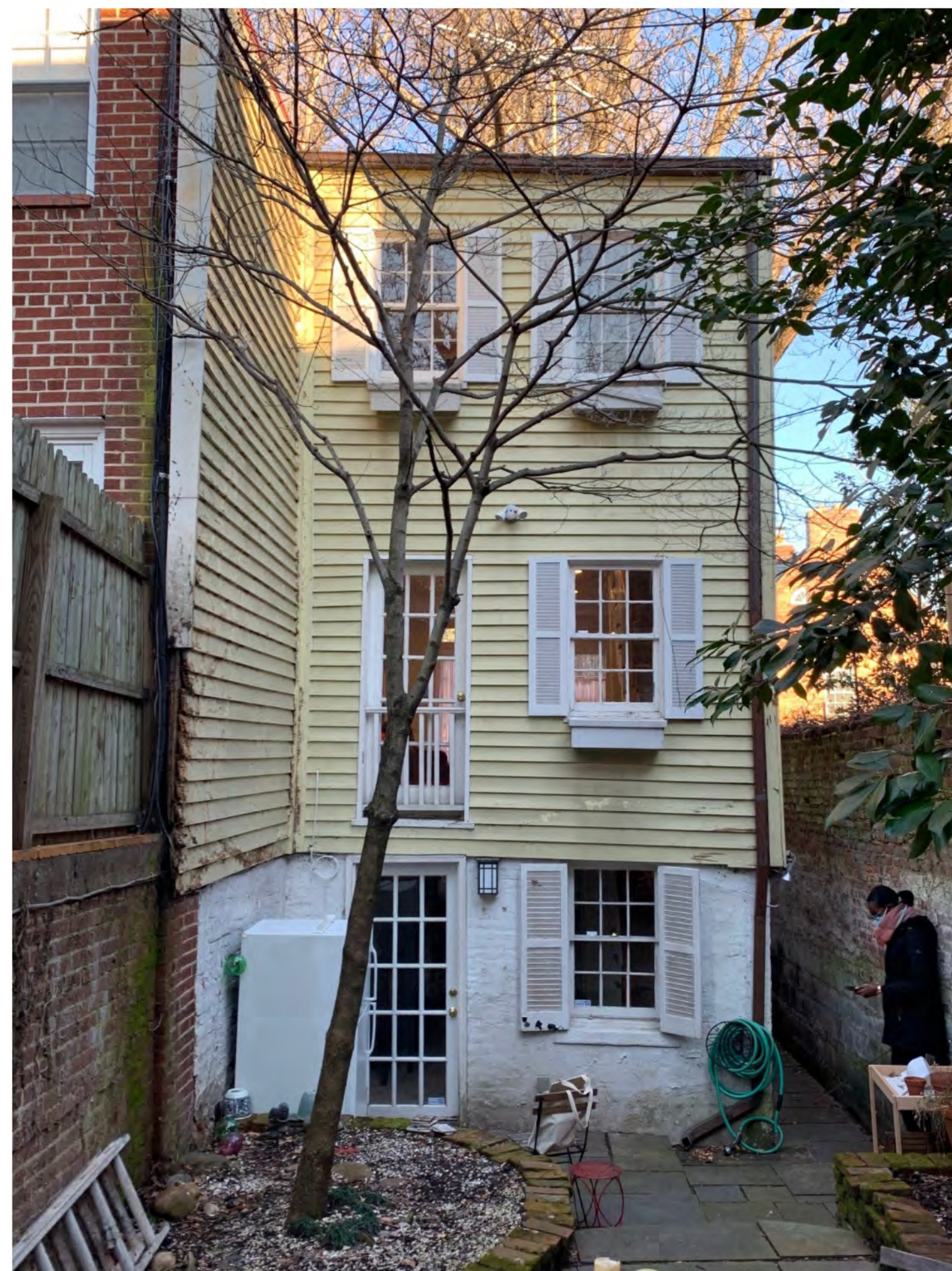
REAR FACADE/ WEST ELEV.
