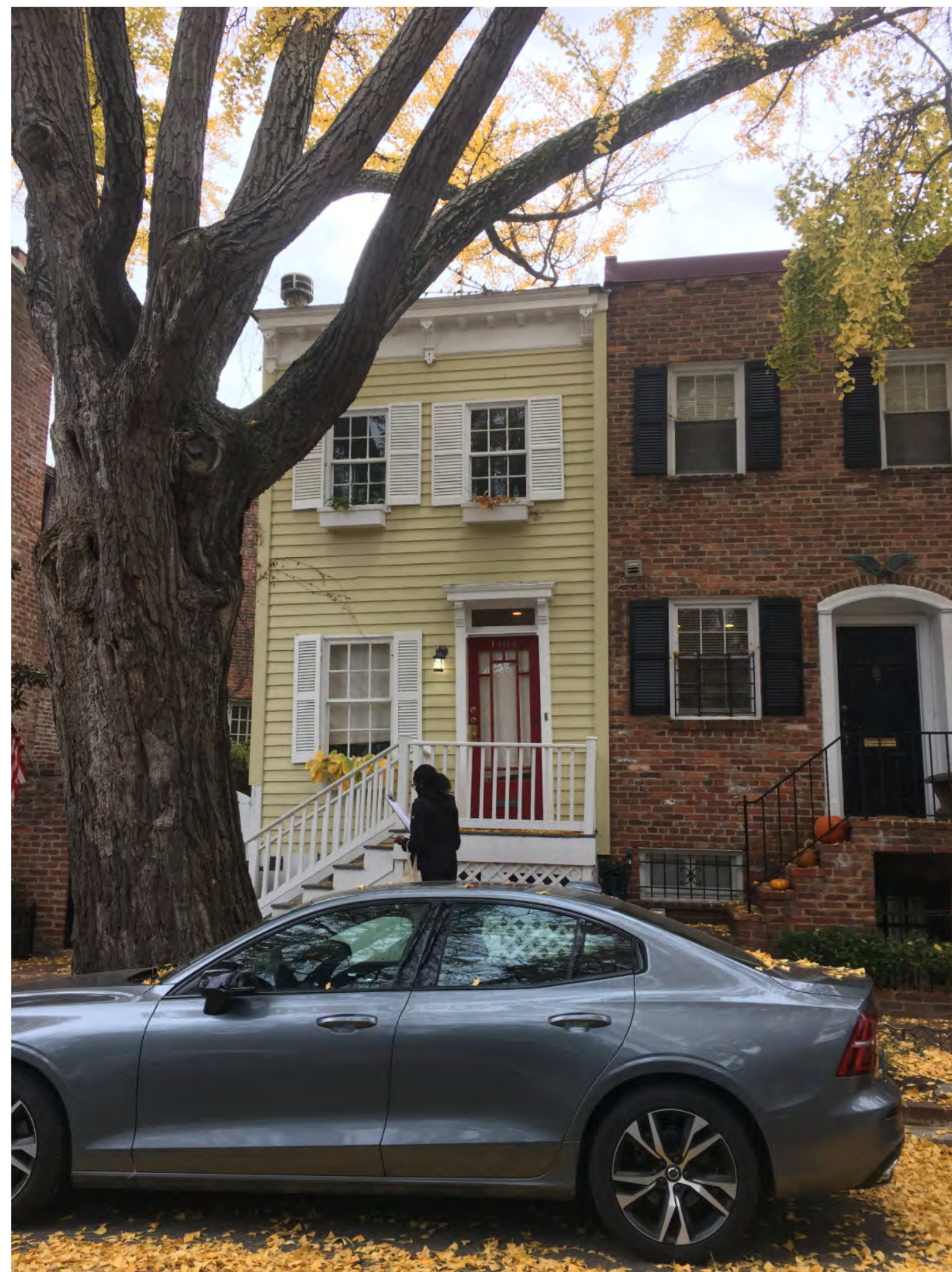
VIEW OF FRONT FACADE/ EAST ELEV.
