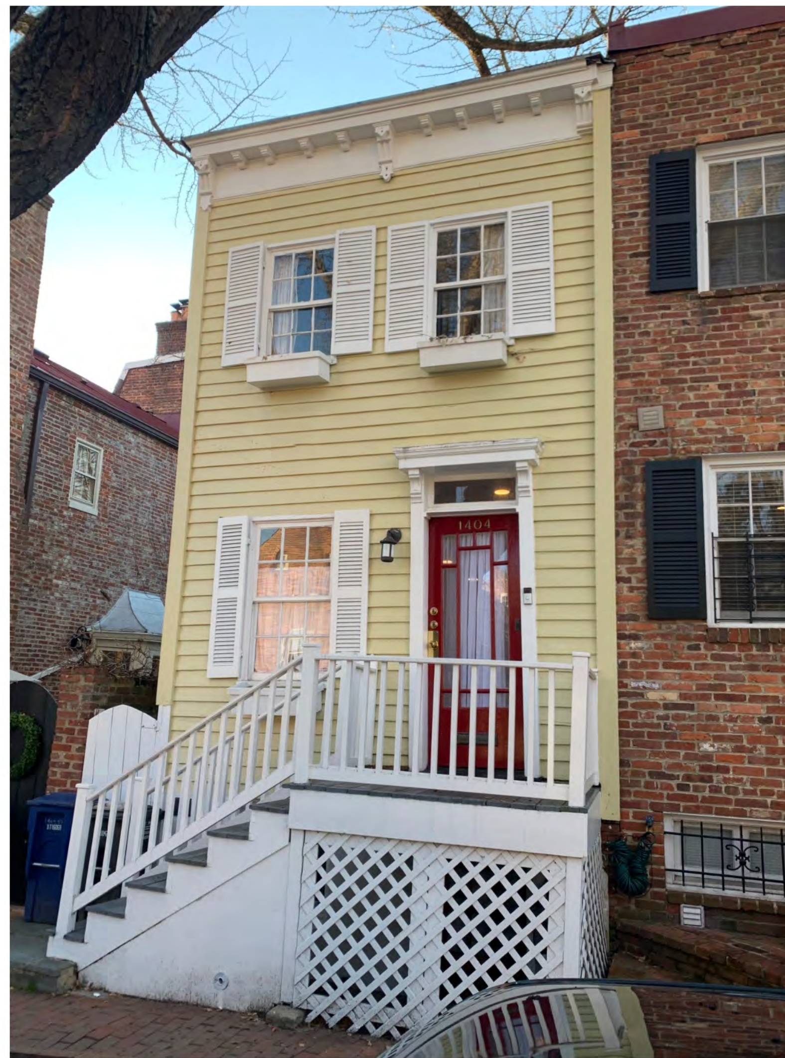
VIEW OF FRONT FACADE/ EAST ELEV.
