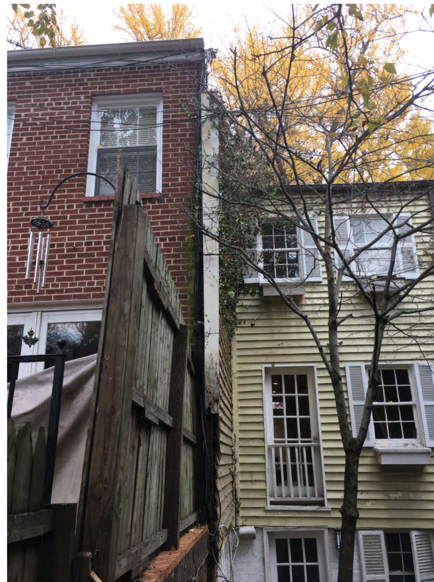
REAR FACADE/ WEST ELEV.
