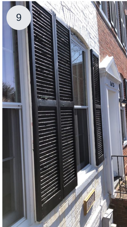
Replacement of 5 pair of shutter that are beyond repair with identical vinyl shutters
