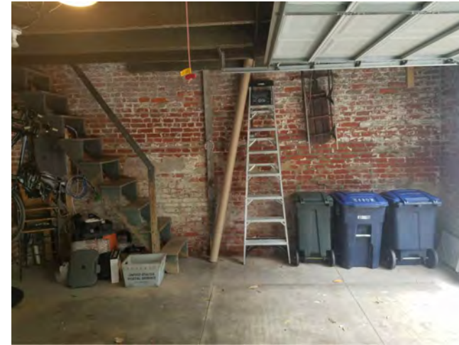
3 FIRST FLOOR INTERIOR: NORTH WALL
