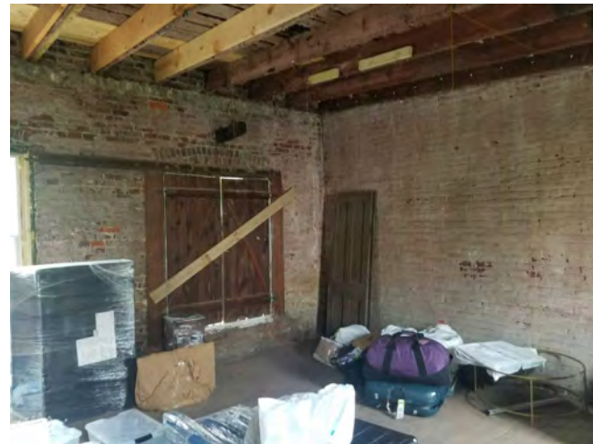
5 SECOND FLOOR INTERIOR
