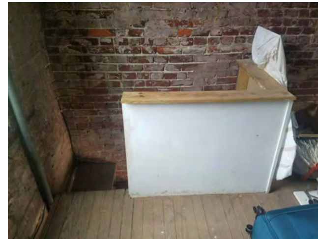
6 SECOND FLOOR INTERIOR: STAIR OPENING
