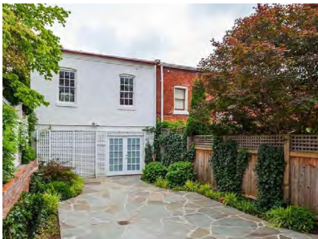
7 EXTERIOR: WEST ELEVATION (GARDEN SIDE)
