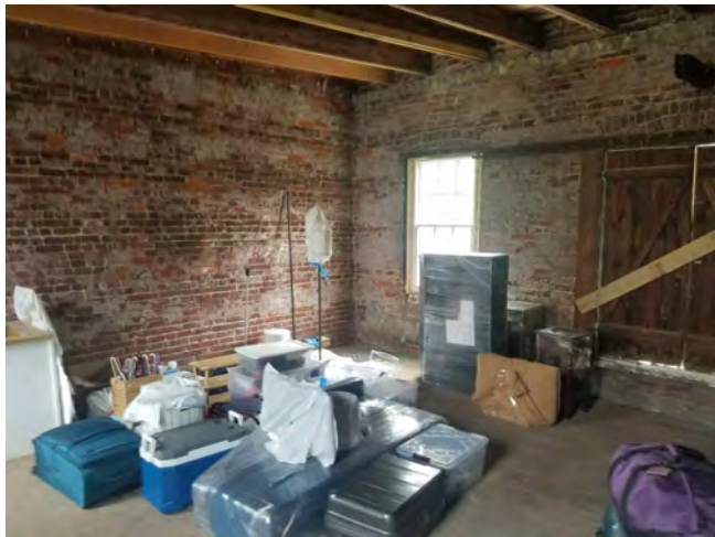
4 SECOND FLOOR INTERIOR
