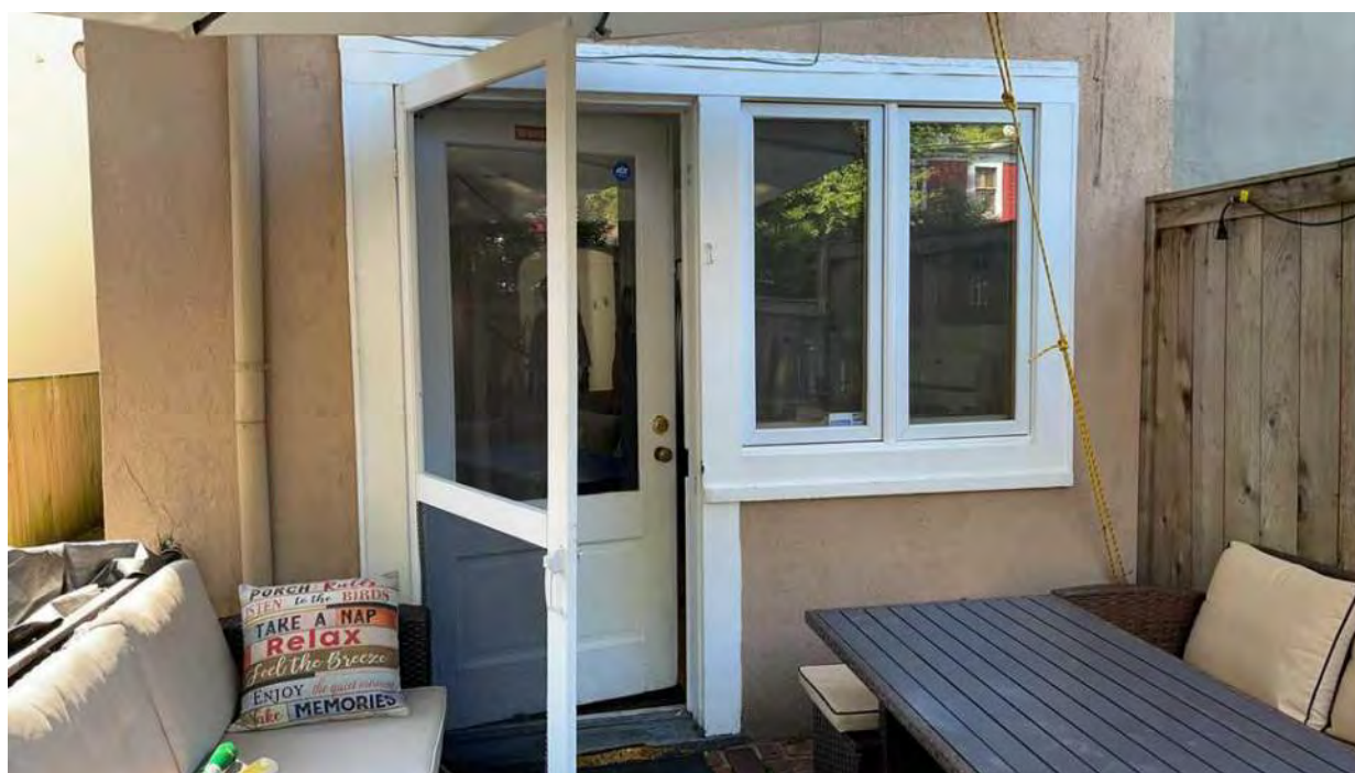
REAR VIEW- EXISTING DOOR & WINDOWS TO BE REPLACED W/ NEW SLIDING DOOR
