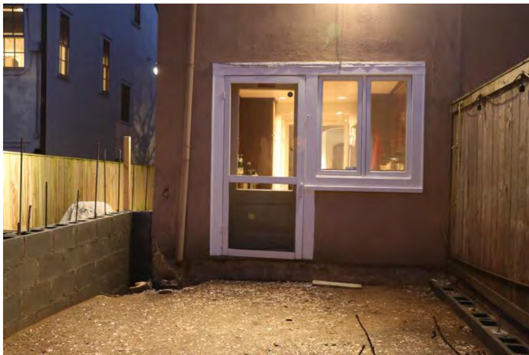
REAR VIEW- EXISTING DOOR & WINDOWS TO BE REPLACED W/ NEW SLIDING DOOR
