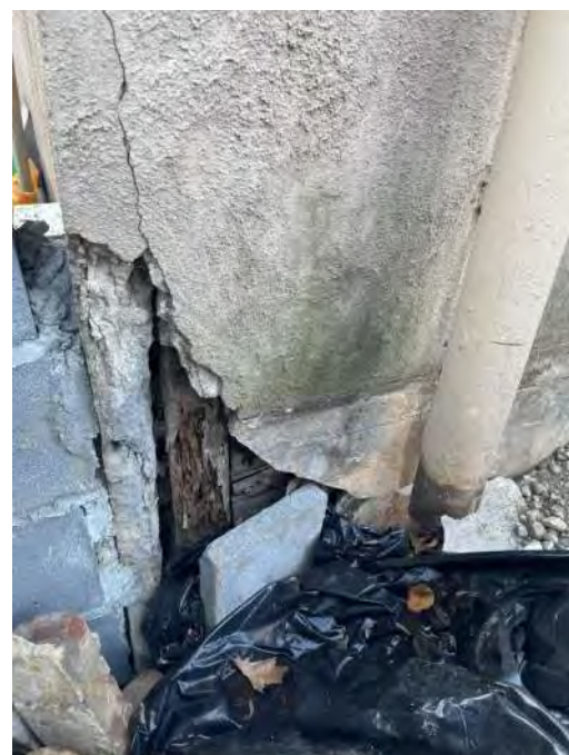
REAR CORNER DAMAGED STUCCO AND WALL (CAUSED BY TREE ROOTS)
