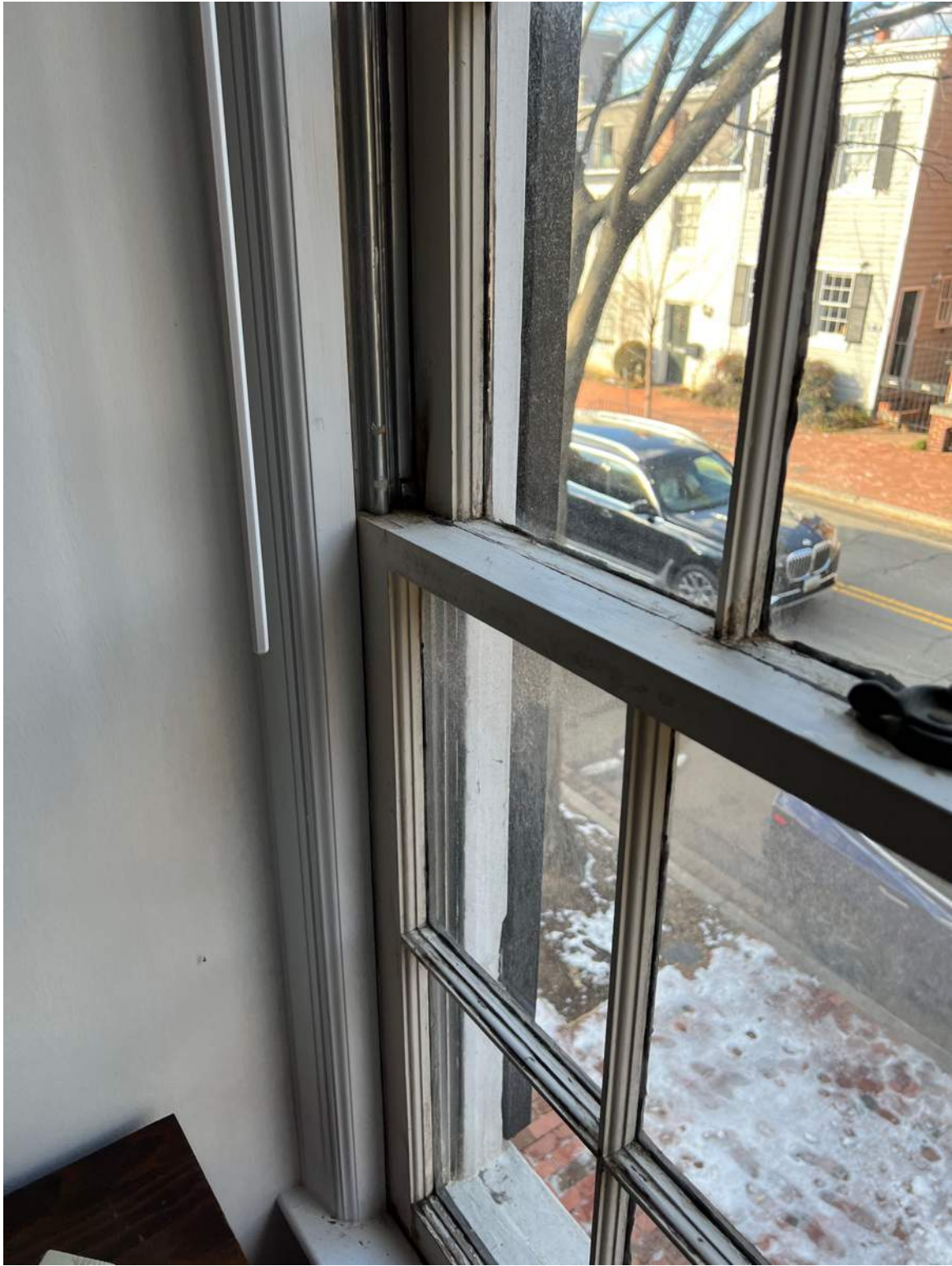
FRONT WINDOW - INTERIOR
