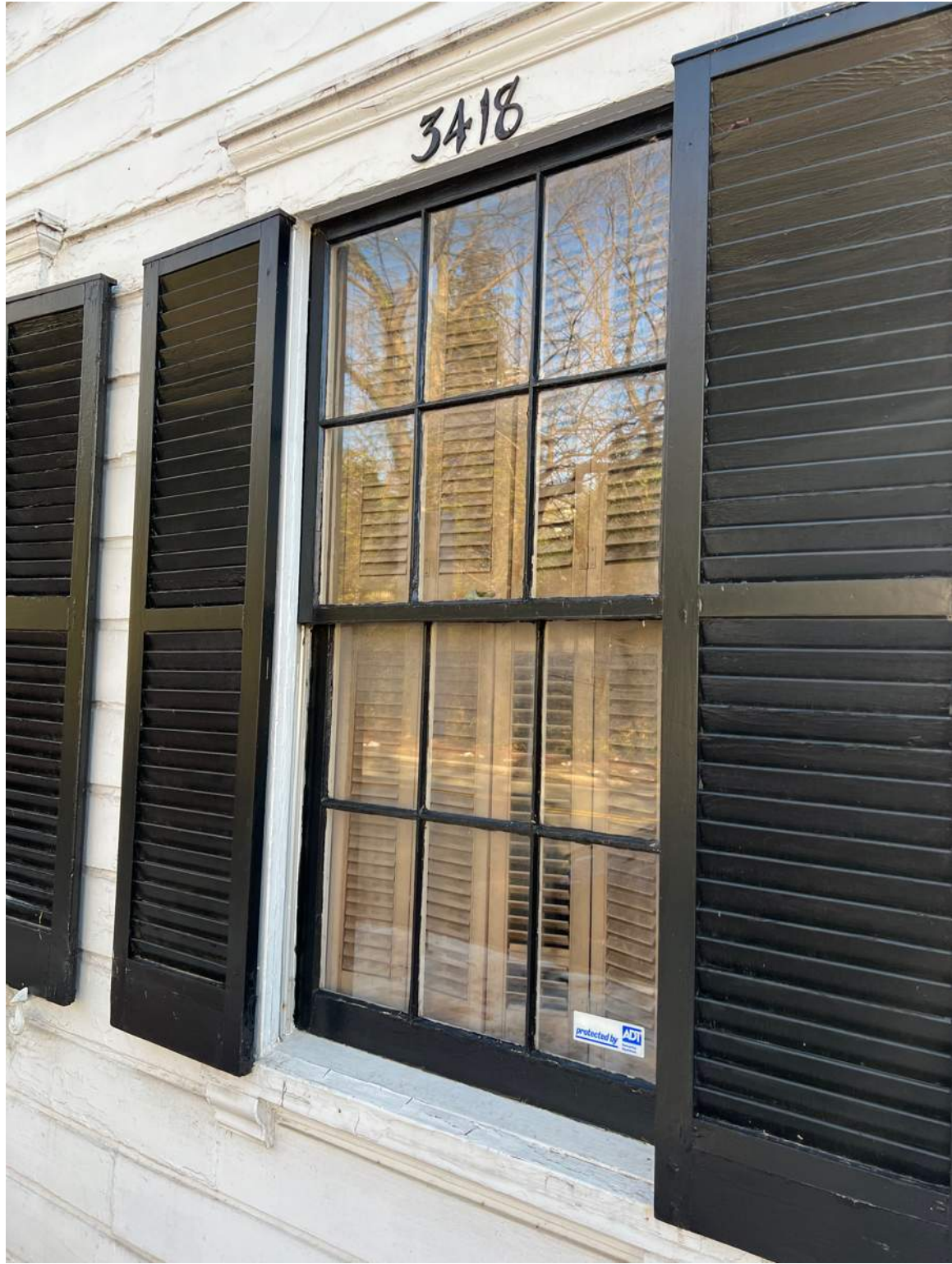
FRONT WINDOW - EXTERIOR
