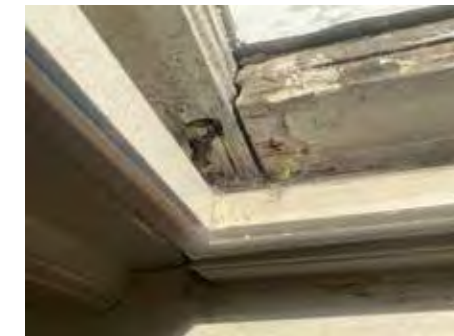
Example window sash rot and damage
