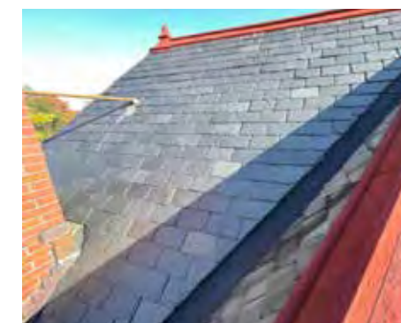
Replacement slate roof tiles at west hip section
