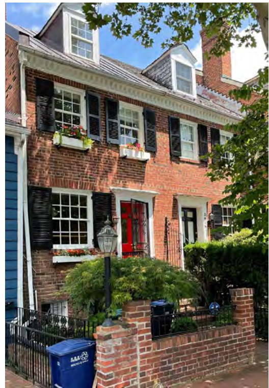
③ O STREET (BUILT 1942)
