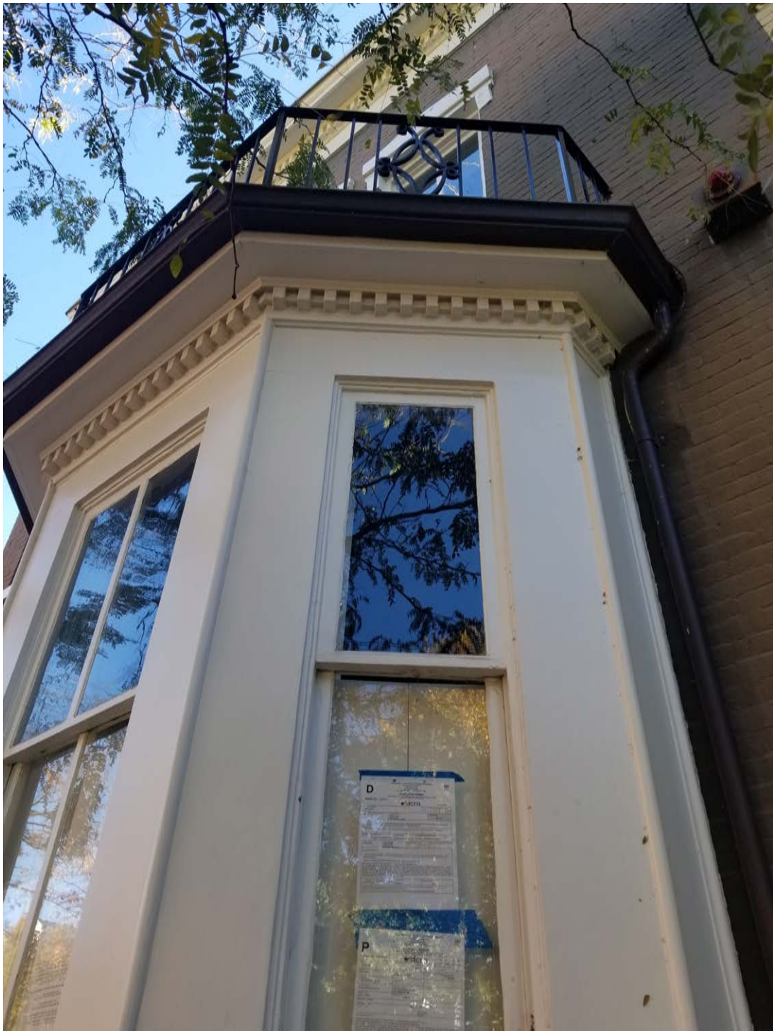
Existing front windows to remain - Four pane with flat bar muntins.
