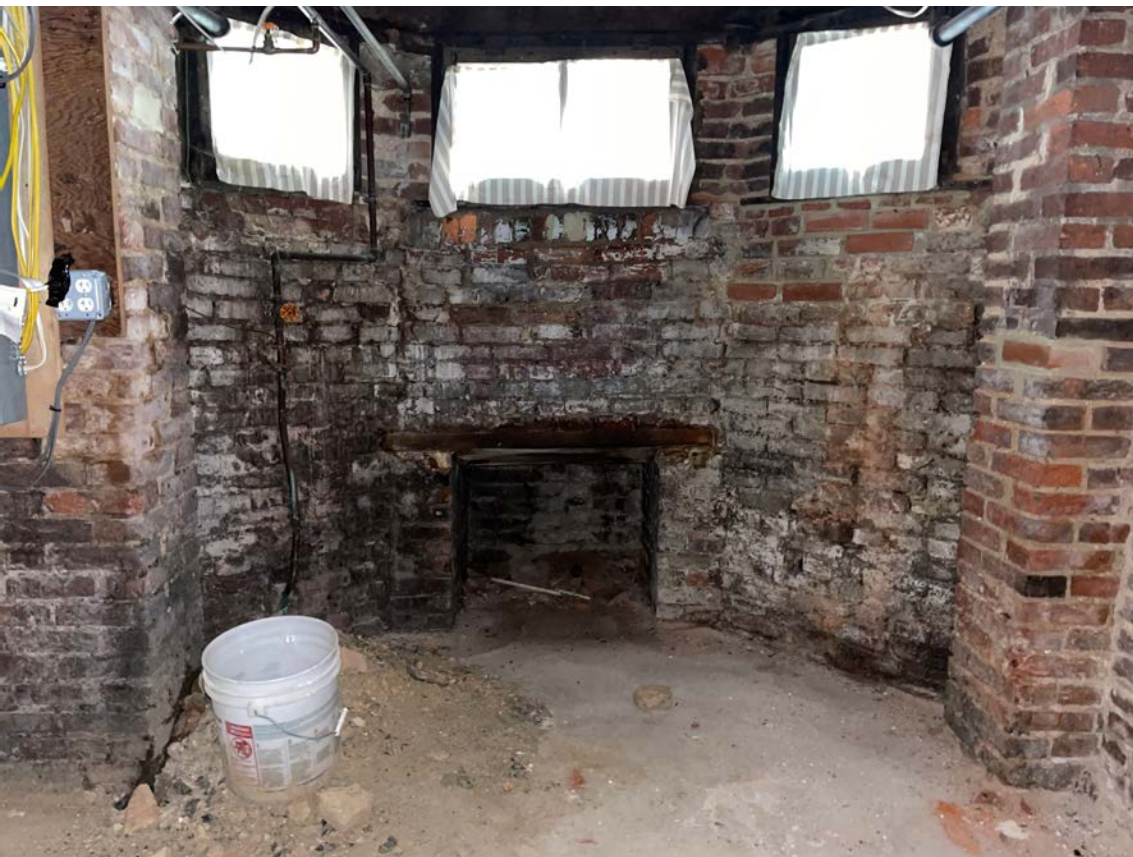
Existing Basement at Front Bay Showing Blocked Up Chute
