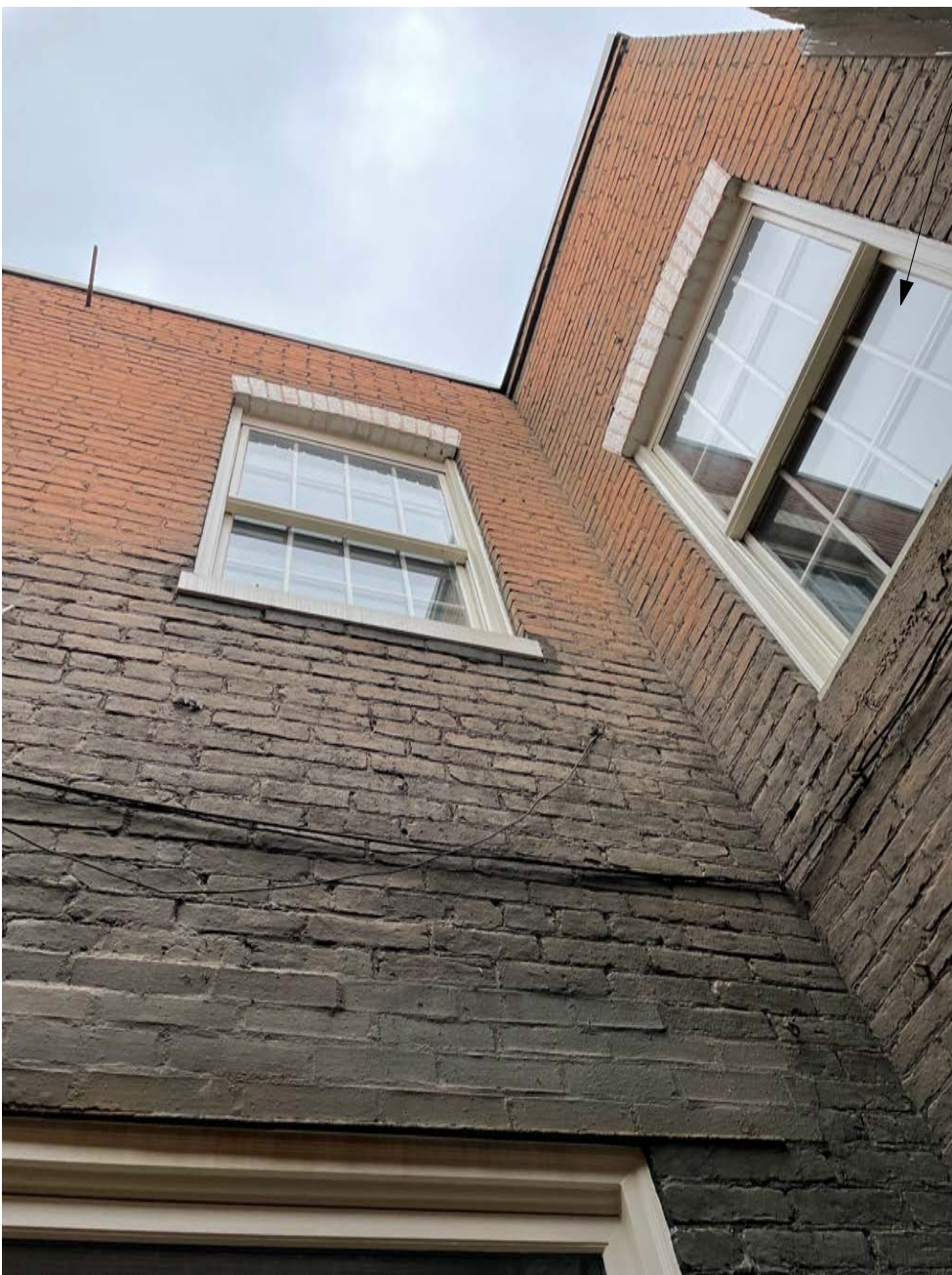
Existing Rear Windows - Simulated divided lite without muntins on exterior with snap in grilles on interior.
