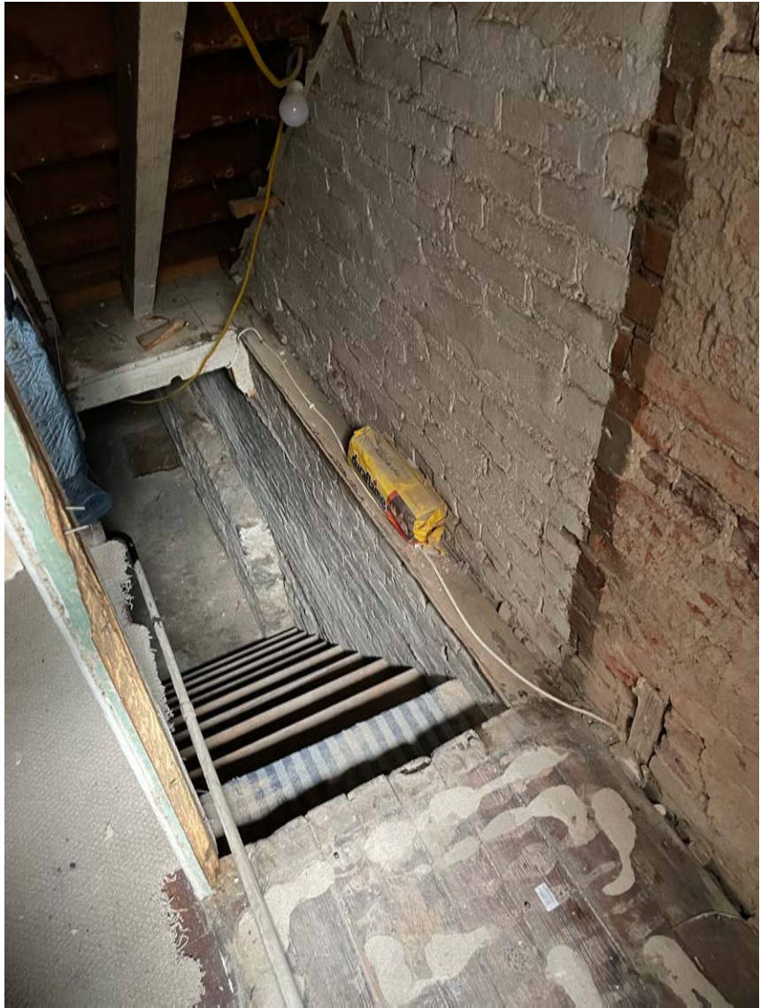
Existing Basement Stair - not to code and not required head room clearance.
