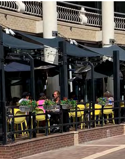
7 Steel Posts w/ Canopy Connections
