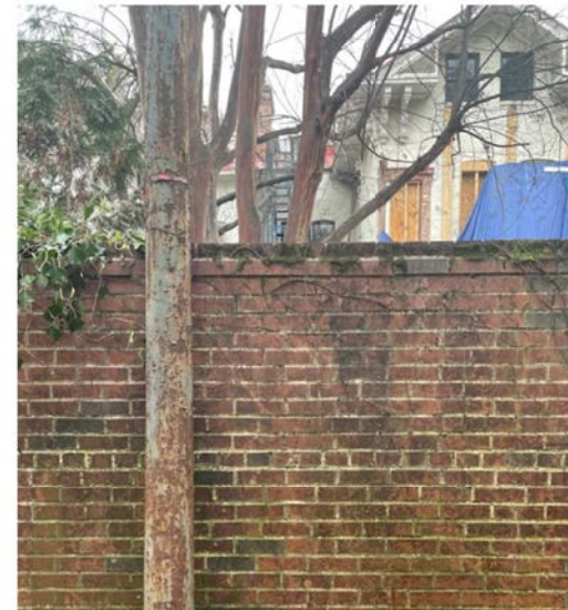
VIEW OF NORTH FACADE FROM ALLEY
