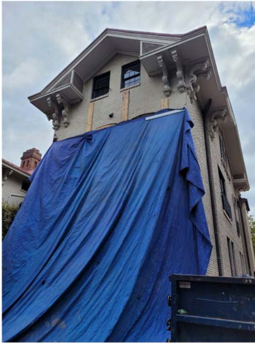
CURRENT VIEW OF DEMO'ED REAR ADDITION (FACING SOUTH)
