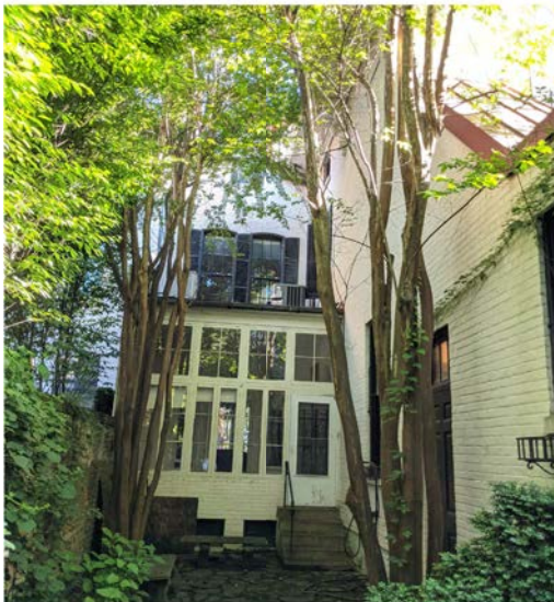
EXISTING SUNROOM ADDITION VIEW W/ EX. AC UNITS (FACING SOUTH)
