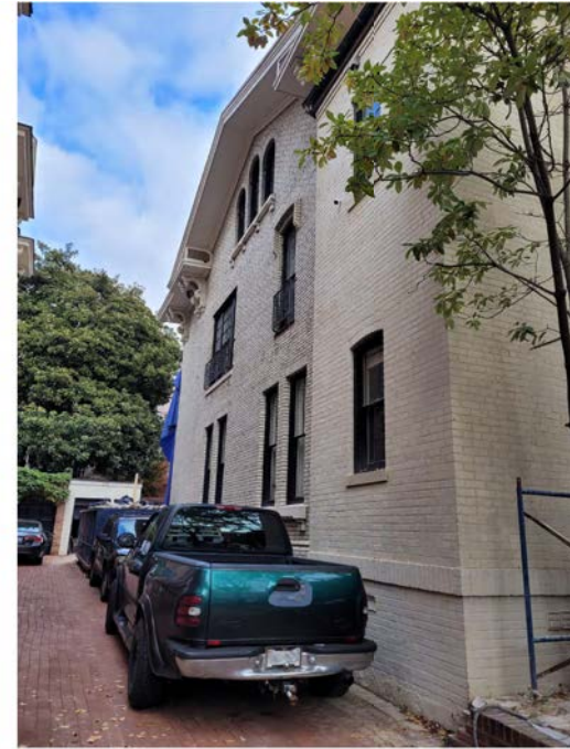
DRIVEWAY (EX. WEST FACADE)
