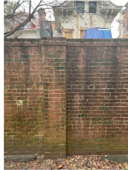
VIEW OF NORTH FACADE FROM ALLEY
