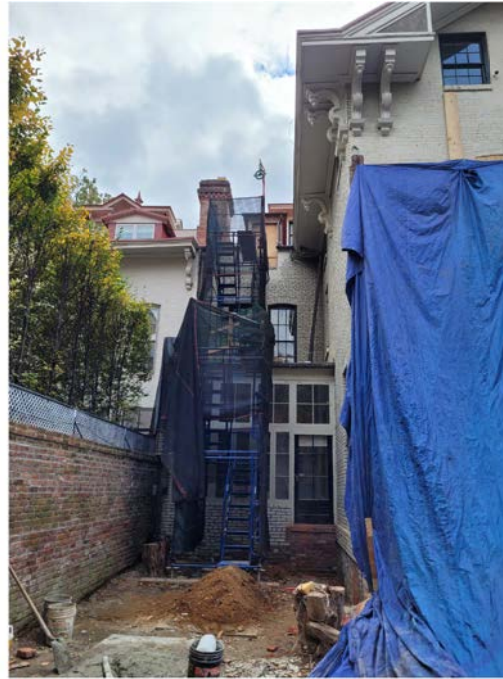
CURRENT VIEW OF SUNROOM (FACING SOUTH)
