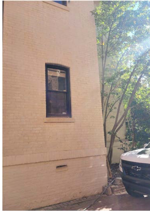
EX. WINDOW (WEST FACADE)
