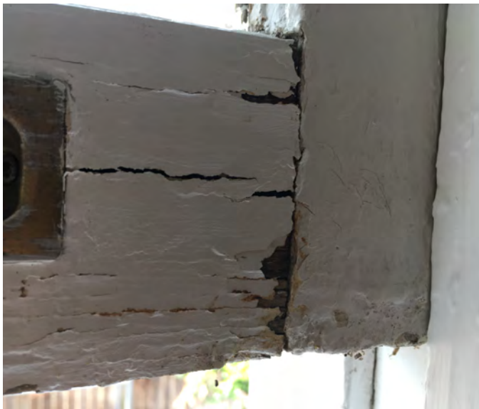
INTERIOR UNIT A (Lower sash, twin window right side from INT) - Lower rail is rotted and splitting from side rail. Failure of joinery. Both upper and lower sash have significant rot issues
