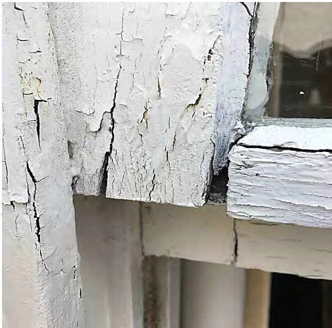
EXTERIOR UNIT B (Upper sash, bathroom window right side from INT) - Sash meeting rail is rotted and splitting and has separated from side rail. Sash is in danger of collapse.
