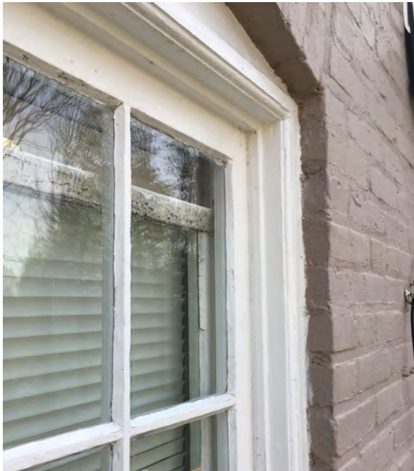
Existing brickmould to be replicated
