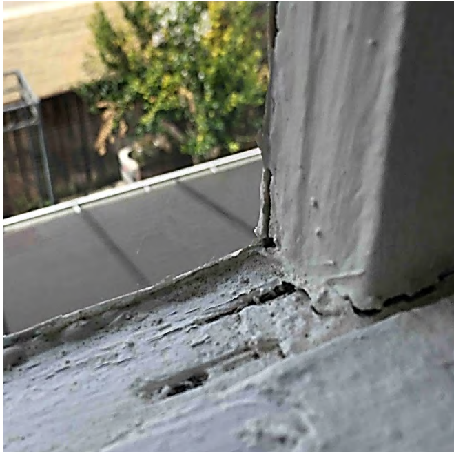
INTERIOR UNIT A (upper sash, twin window right side from INT) - Meeting rail is rotted and splitting. Attempts at repairs with bondo have failed.
