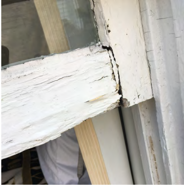
EXTERIOR UNIT A (Lower sash, twin window right side from INT) - Sash lower rail is severely rotted and has separated from side rail.
