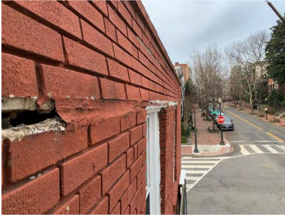
Photograph #3: Closeup View of Brick Masonry Displacement & Horizontal Separation along Mortar Joint & Window Head Lintel
