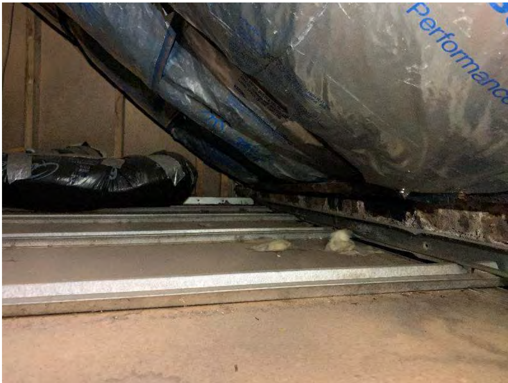
Photograph #8: View of Roof Structure Bearing onto Brick Masonry Veneer at Exploratory Probe – Interior
