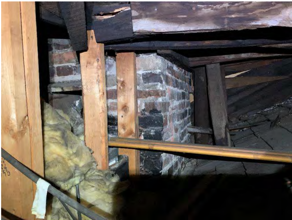
Photograph #10: View of Roof Framing & Vertical Stud Framing at Interface with Adjacent Building Multi-Wythe Wall
