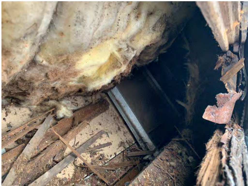
Photograph #6: View of Wood Rot & Steel Studs at Gutter Exploratory Probe – Exterior
