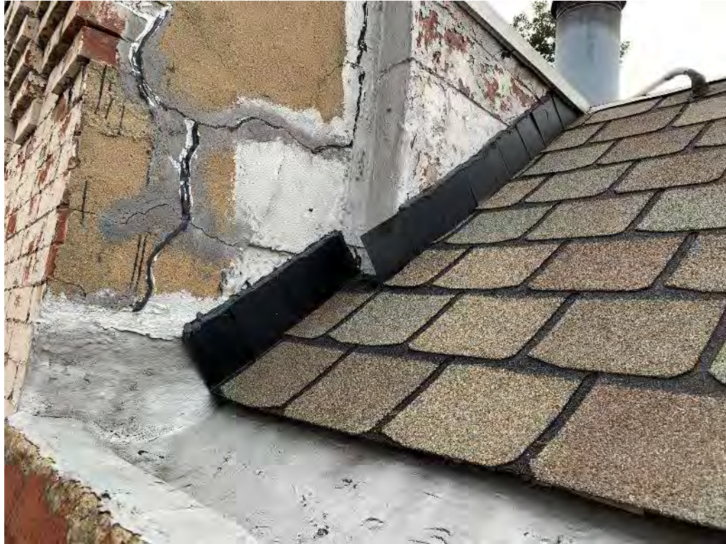
Photograph #5: View of Roof Flashing & Roof Gutter at Interface with Adjacent Building
