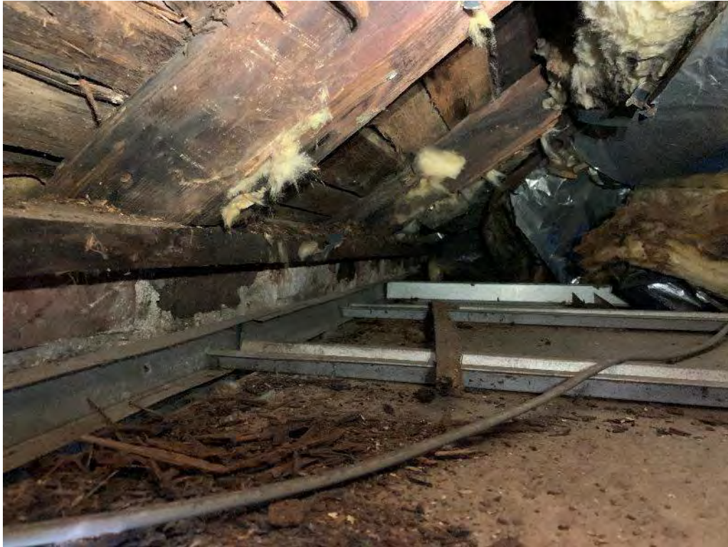
Photograph #7: View of Roof Structure Bearing onto Brick Masonry Veneer at Exploratory Probe – Interior
