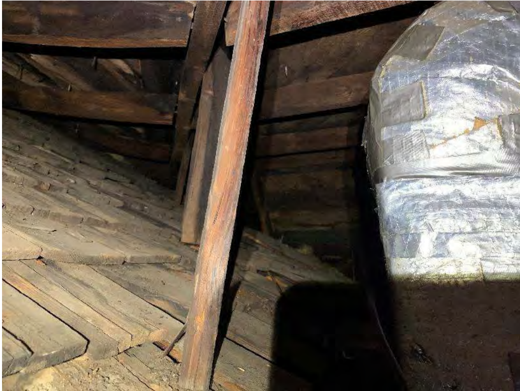
Photograph #9: View of Typical Roof Framing Elements Bearing onto Original Roof Below
