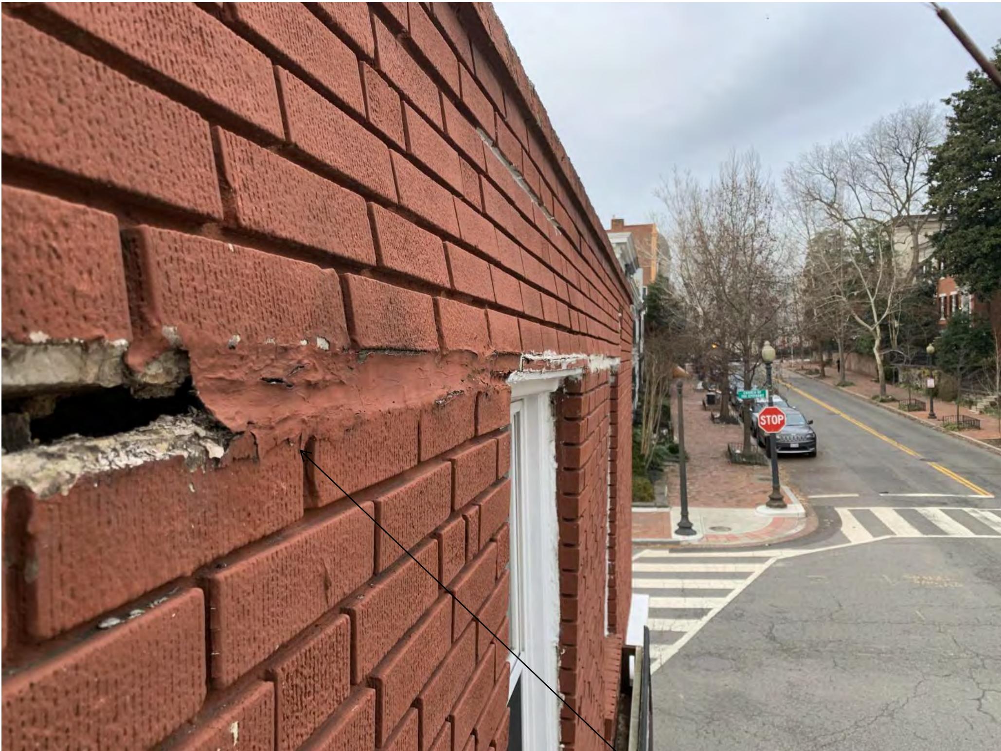
VIEW OF DISPLACED BRICK VENEER & HORIZONTAL SEPARATION ALIGNED WITH WINDOW HEAD
