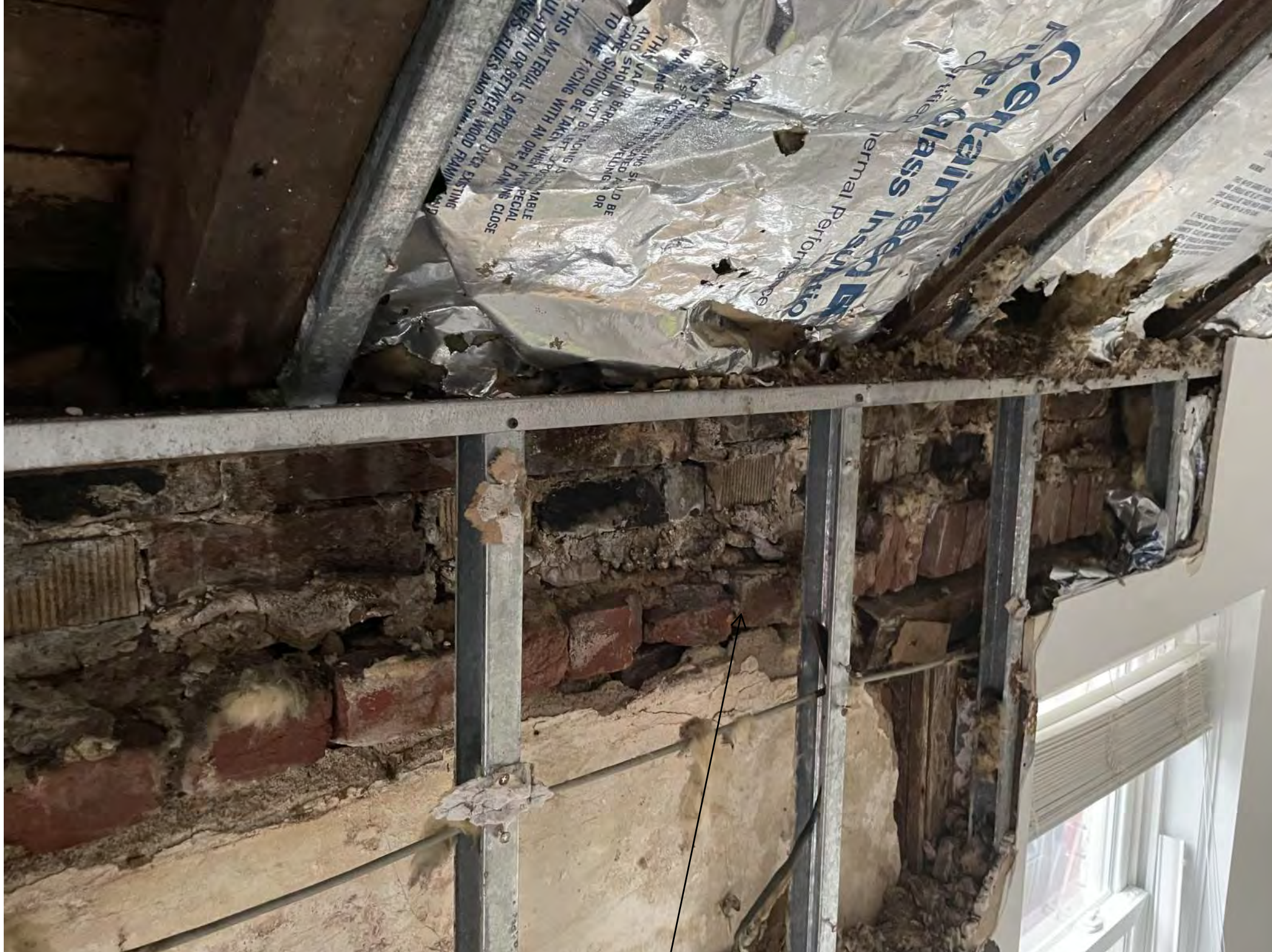
INTERIOR VIEW OF BRICK MASONRY & HIP ROOF FRAMING BEARING ONTO WALL
