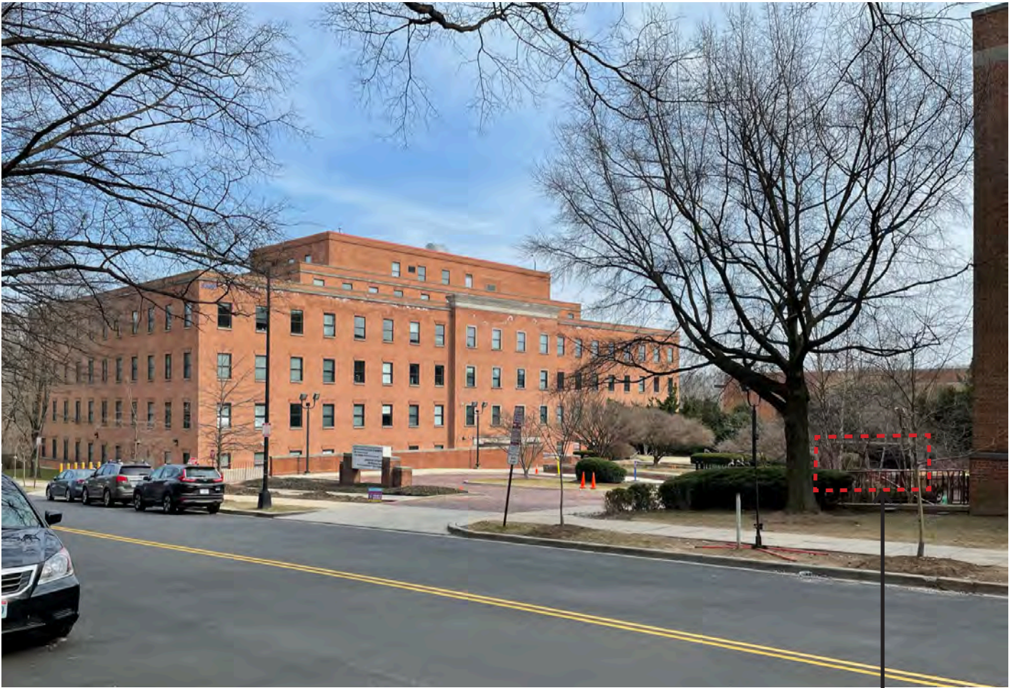
View of existing conditions
