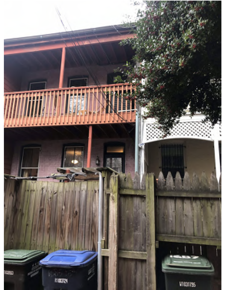
VIEW OF NEIGHBORING YARD FROM ALLEY
