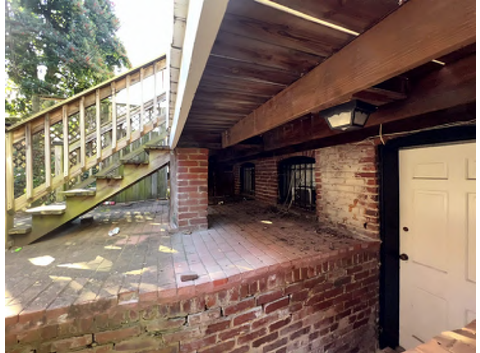
VIEW OF EXISTING MASONRY PIER FOUNDATION.
