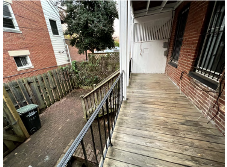
VIEW OF REAR YARD FROM EXISTING DECK.
