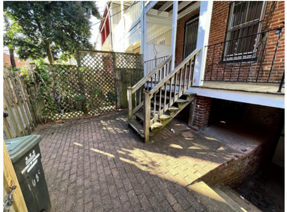
VIEW OF EXISTING DECK FROM REAR YARD.
