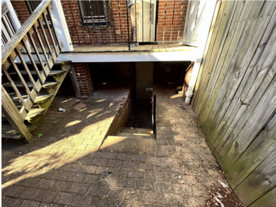
VIEW OF EXISTING AREAWAY FROM REAR YARD.
