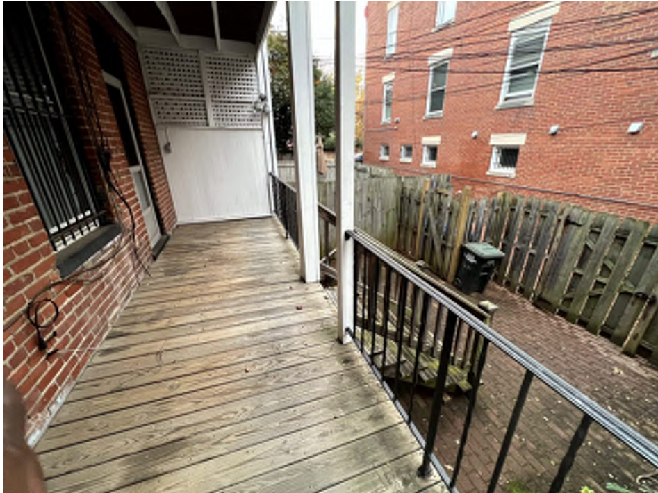
VIEW OF REAR YARD FROM EXISTING DECK.
