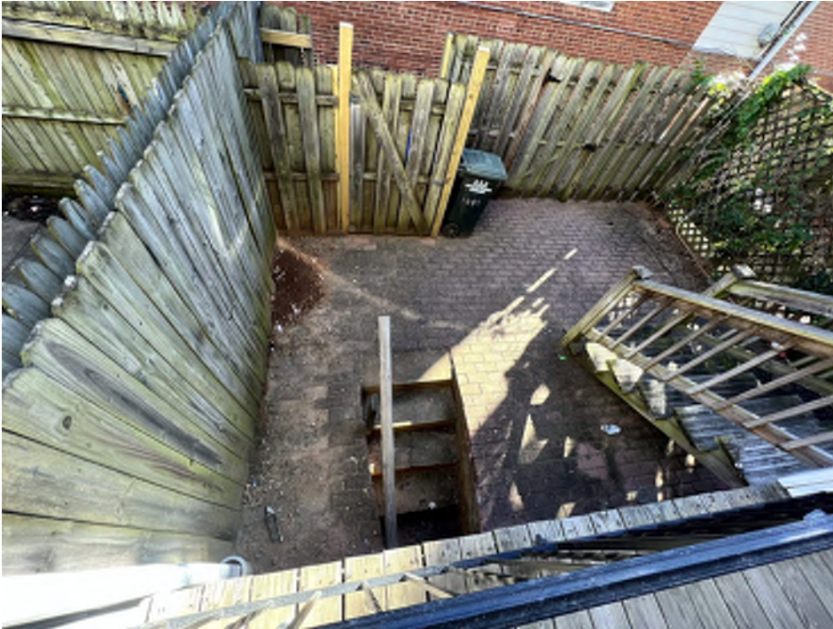
VIEW OF REAR YARD FROM EXISTING DECK.
