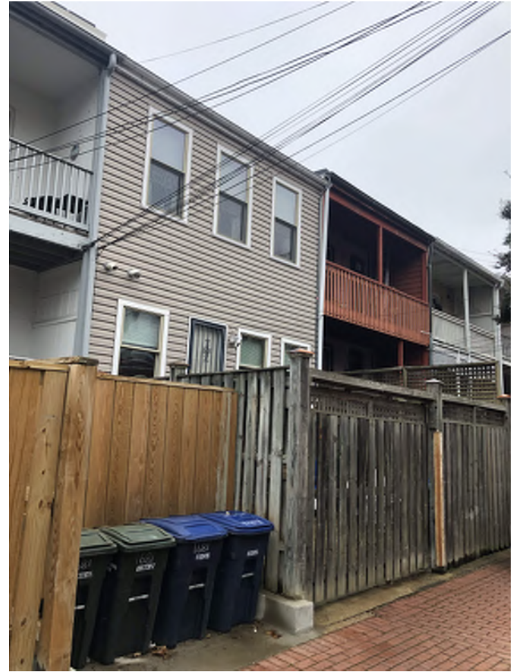
VIEW OF NEIGHBORING YARD FROM ALLEY
