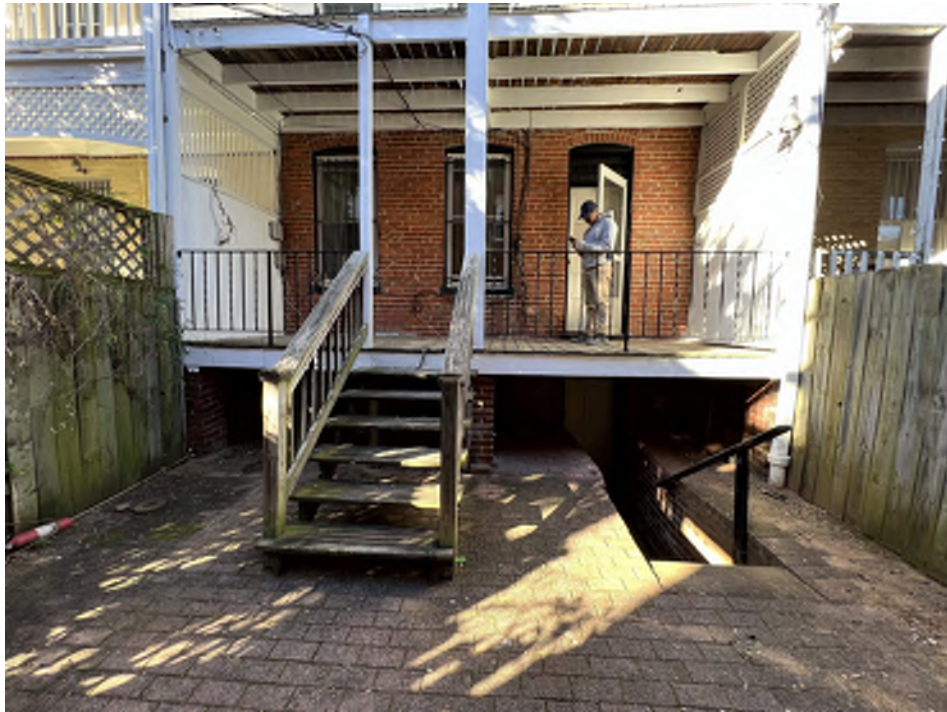
VIEW OF EXISTING DECK FROM REAR YARD.
