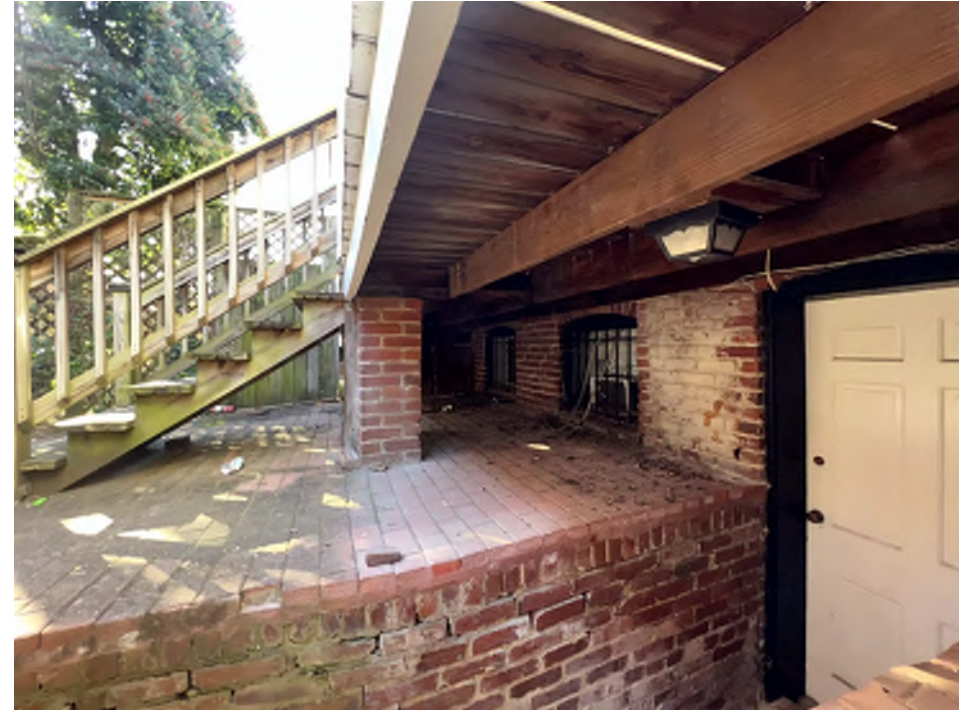
VIEW OF EXISTING MASONRY PIER FOUNDATION.
