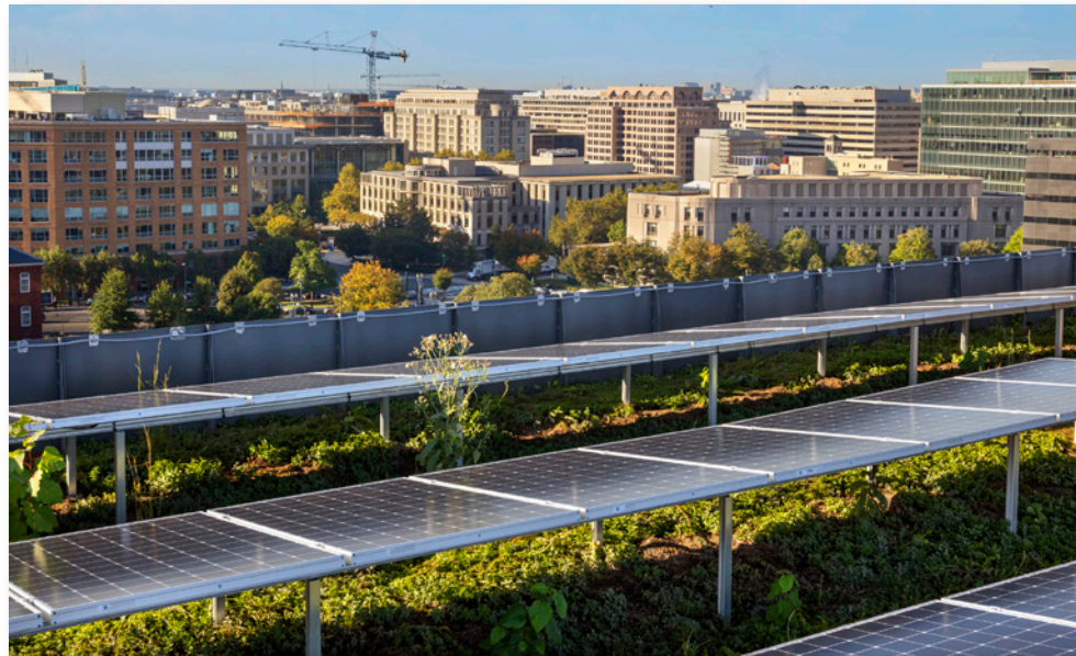
SOLAR-OVER-GREEN ROOF - GU PRECEDENT
