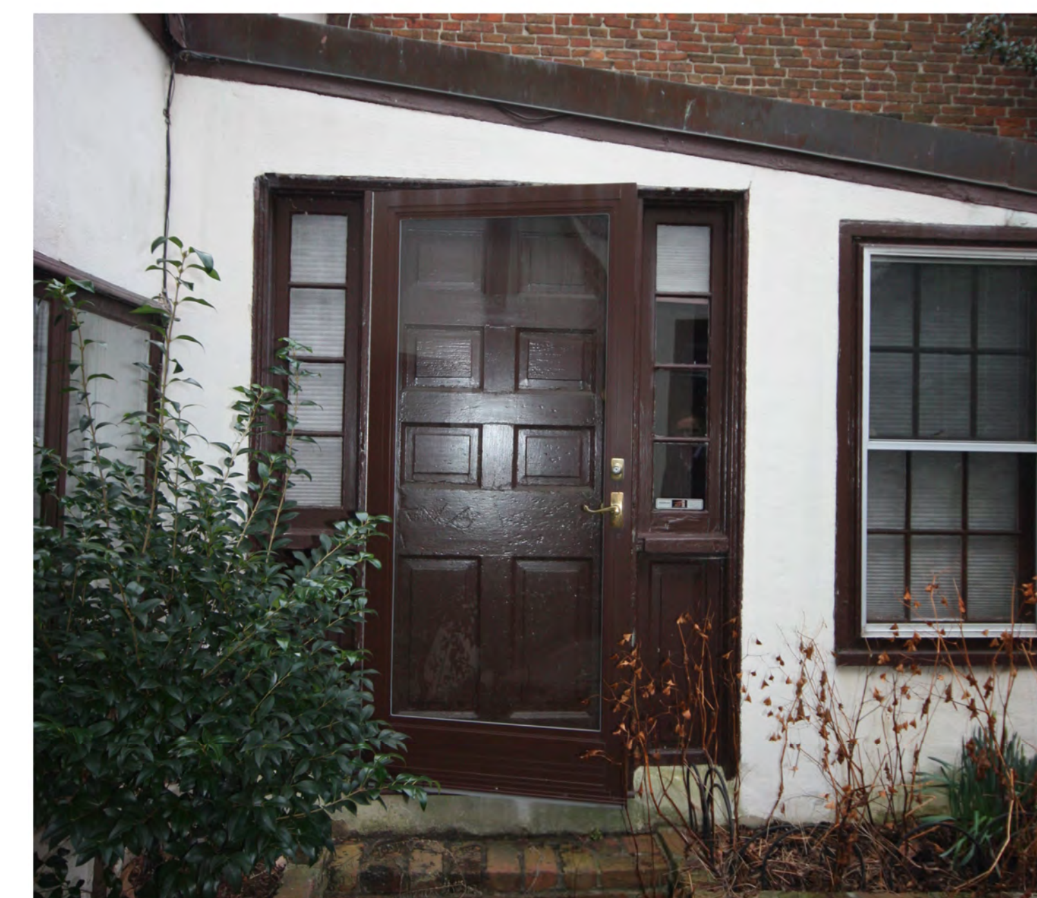
EXISTING DOOR INTO OFFICE
