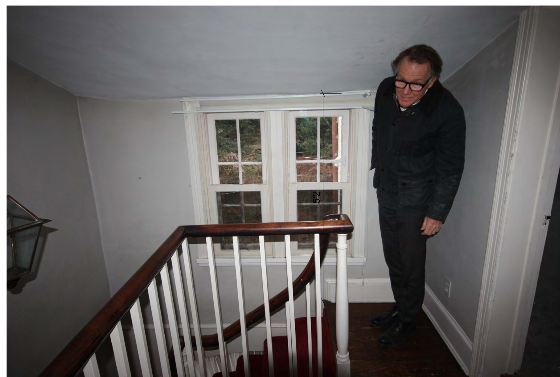
EXISTING SECOND FLOOR LANDING FROM MAIN STAIR
