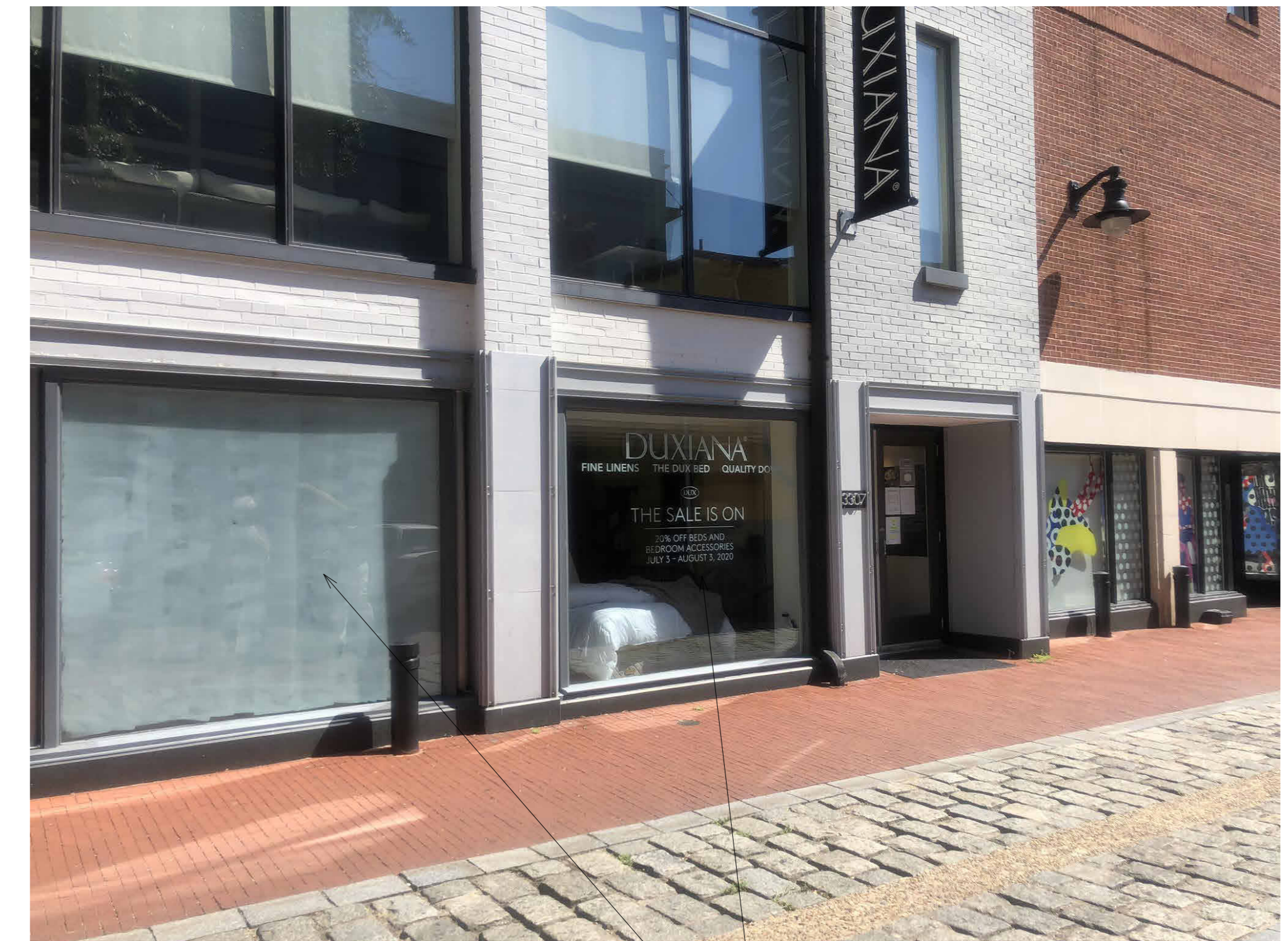
CADY'S ALLEY LEVEL WINDOWS TO BE REPLACED
