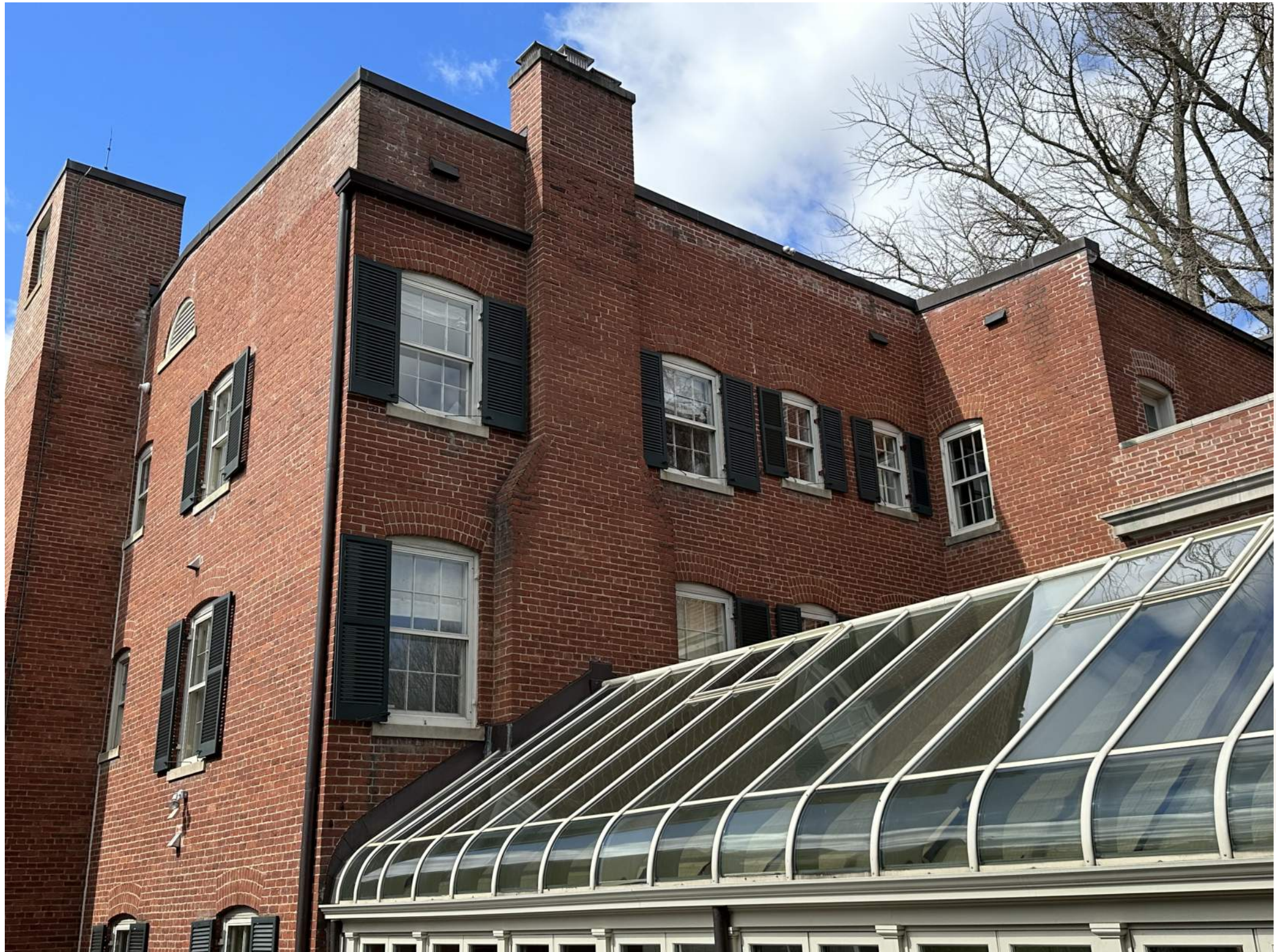
REPOINT EXISTING MASONRY BRICK WALLS
