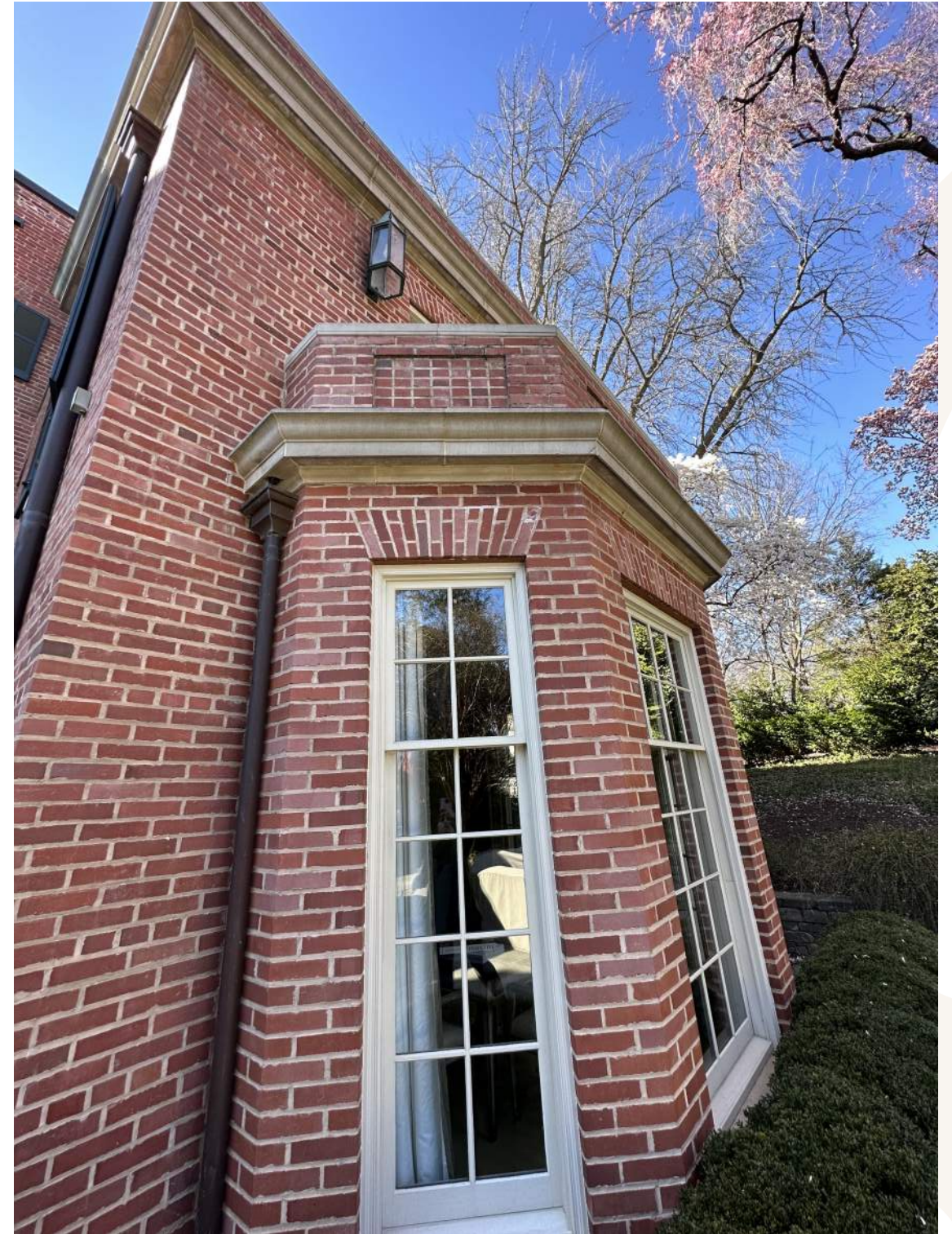
REPOINT EXISTING MASONRY BRICK WALLS
