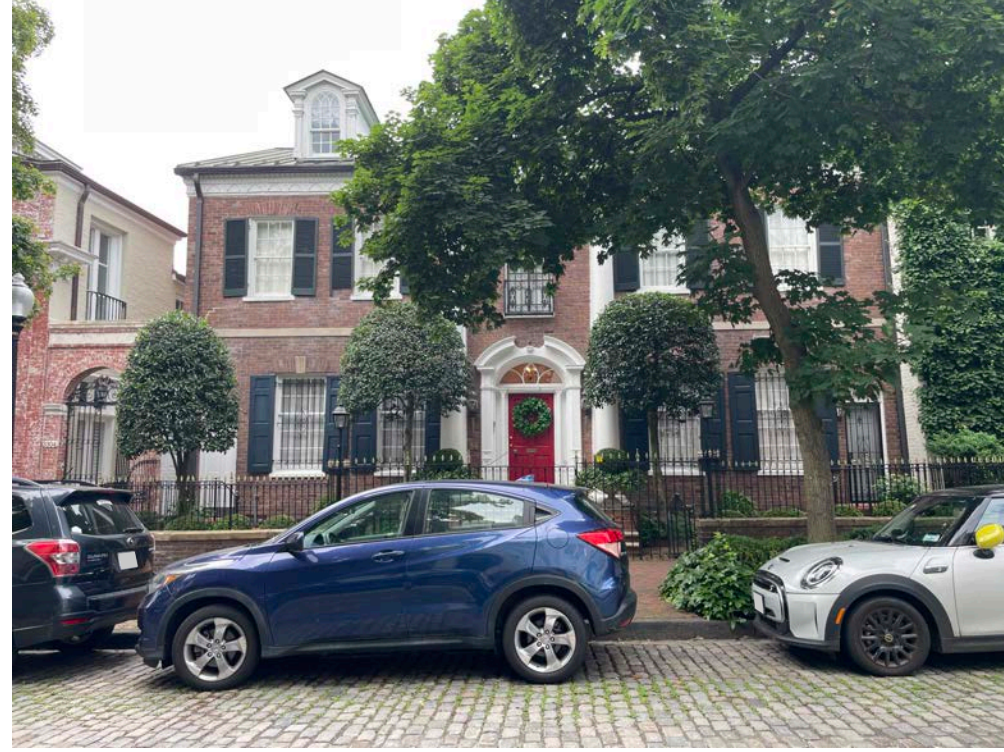
APPROACHING FRONT OF SITE FROM CENTER
