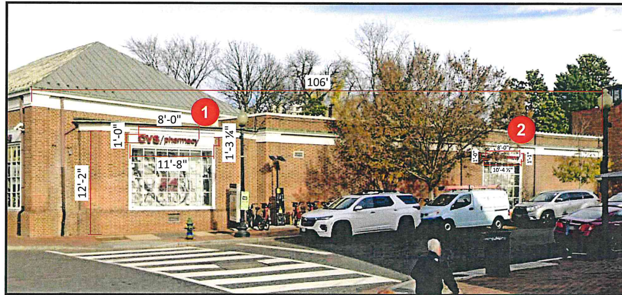
EXISTING CONDITIONS - LONG FRONT ELEVATION
