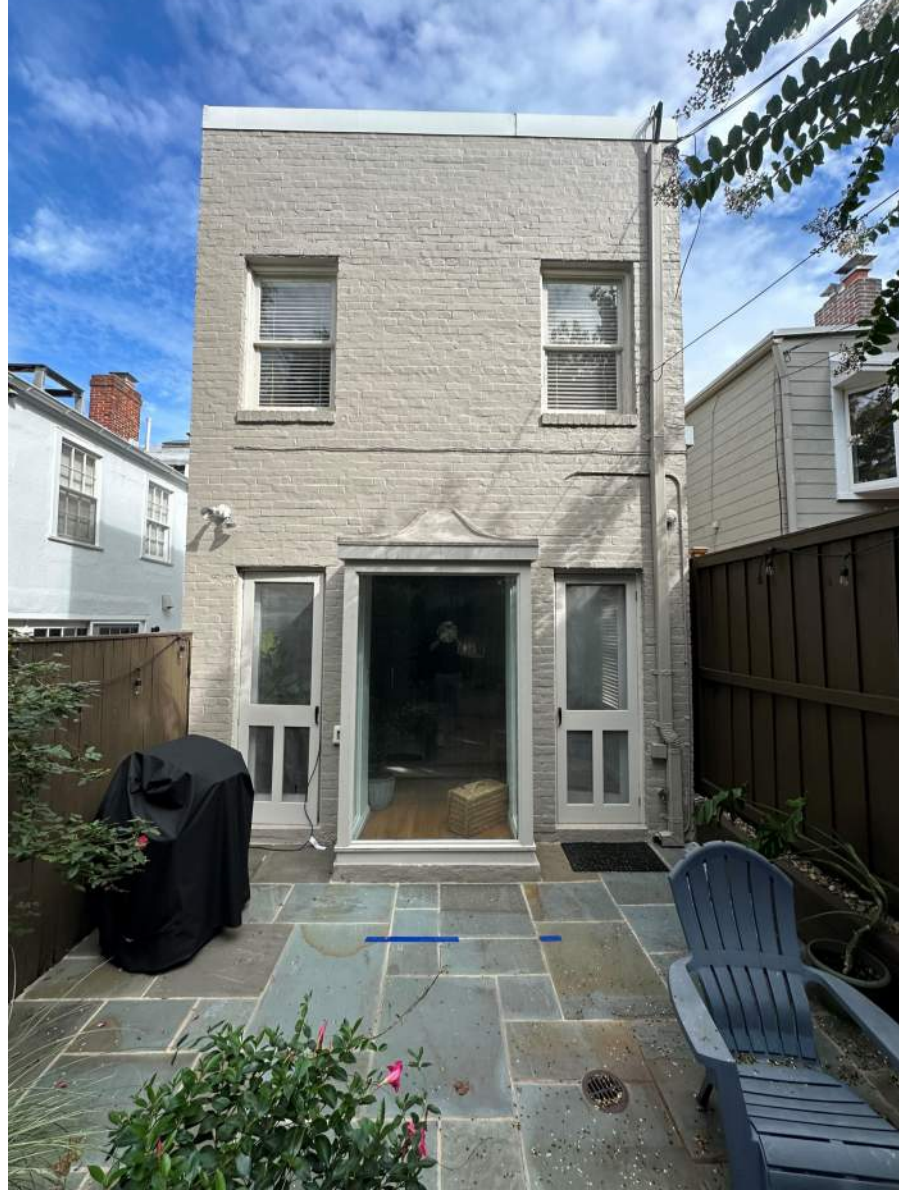
REAR EXISTING VIEW
