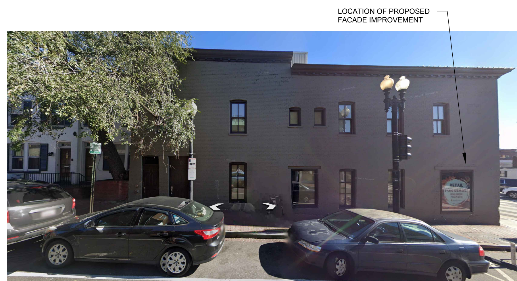
VIEW OF WEST SIDE OF BUILDING
