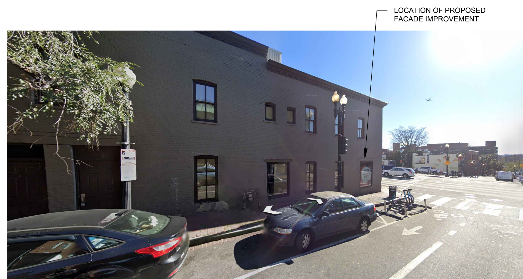
VIEW APPROACHING FROM WEST SIDE OF BUILDING
