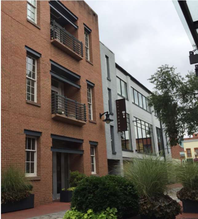
4 CONTEXT PHOTO CADY'S ALLEY LOOKING NORTHEAST
