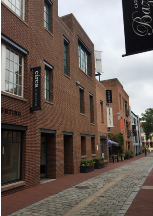
6 CONTEXT PHOTO CADY'S ALLEY LOOKING NORTH
