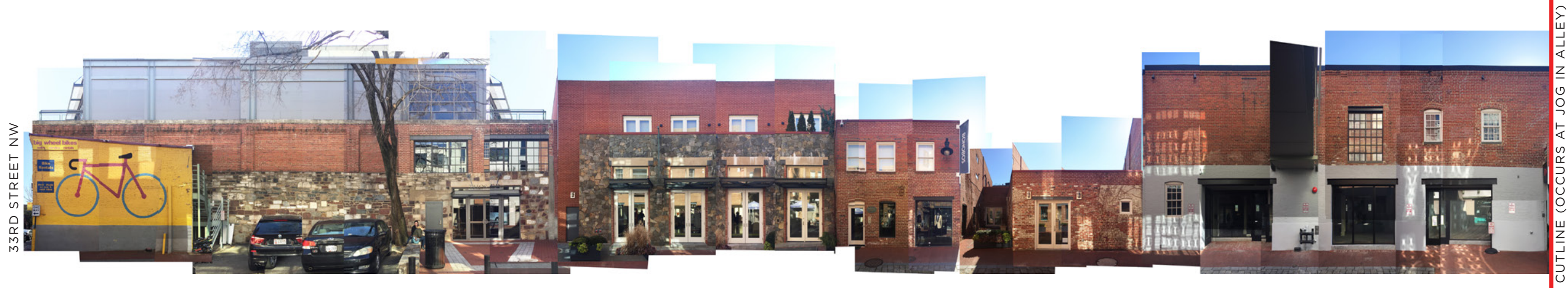
1a CONTEXT PHOTO COLLAGE CADY'S ALLEY LOOKING SOUTH - EASTERN PORTION
