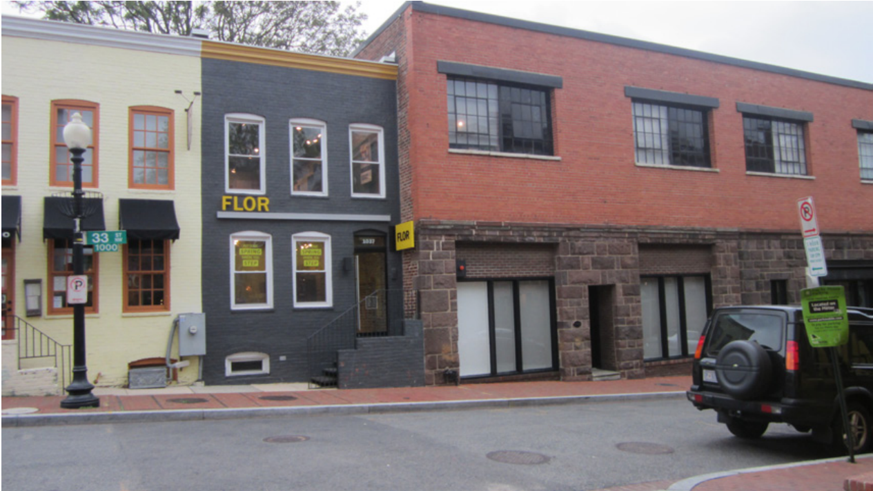
7 CONTEXT PHOTO 33RD STREET LOOKING EAST
