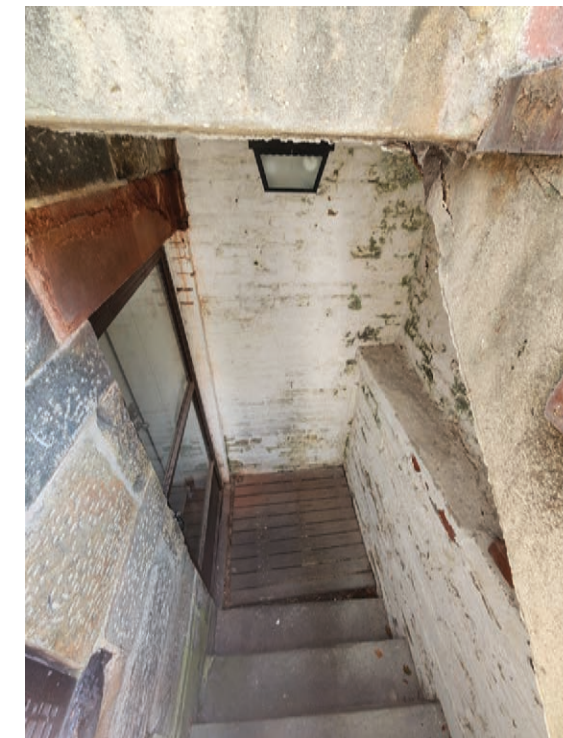
VIEW OF THE BASEMENT AREAWAY
