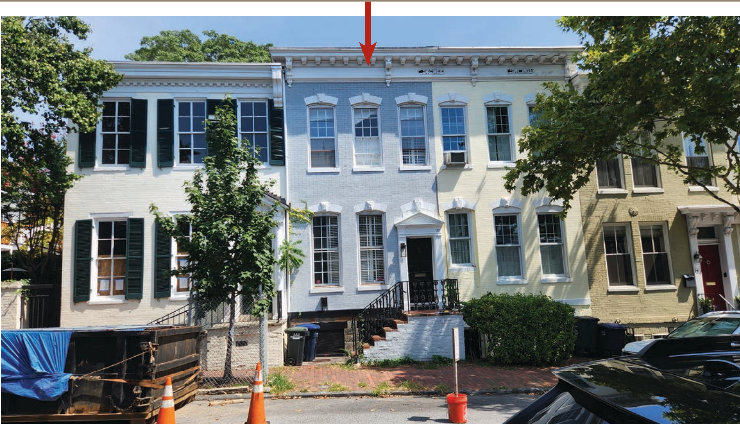
VIEW OF PROPERTY FROM ACROSS THE STREET
