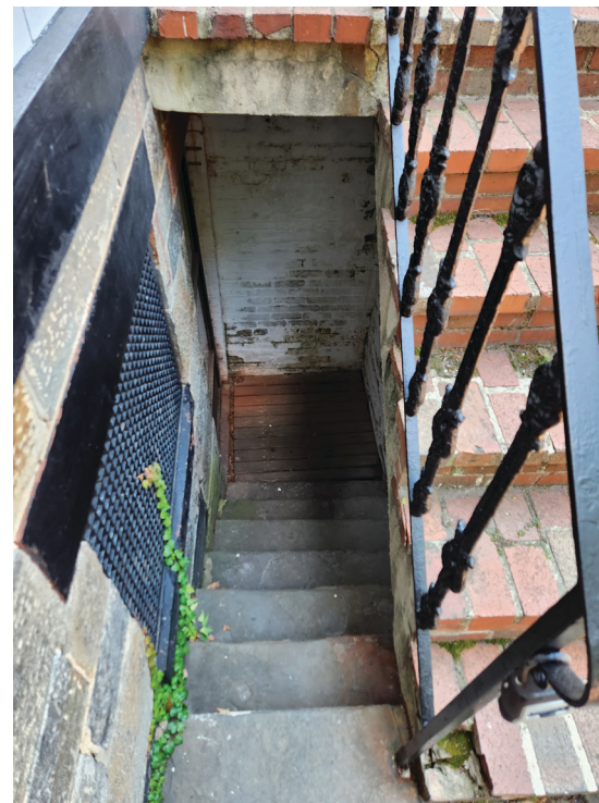
STAIRS DOWN TO THE BASEMENT
