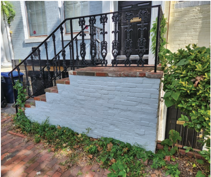
DETAIL VIEW OF FRONT STOOP
