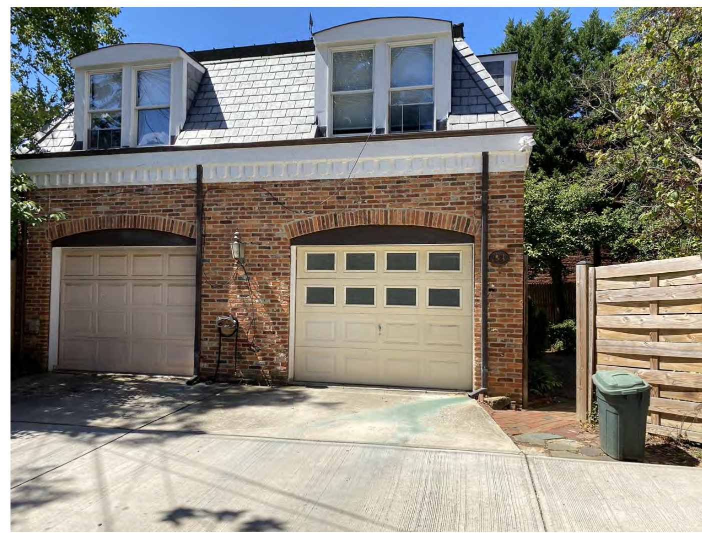
View of Garage and Concrete Pad and Gate From The Alley (Prior to Start of House Renovation)
