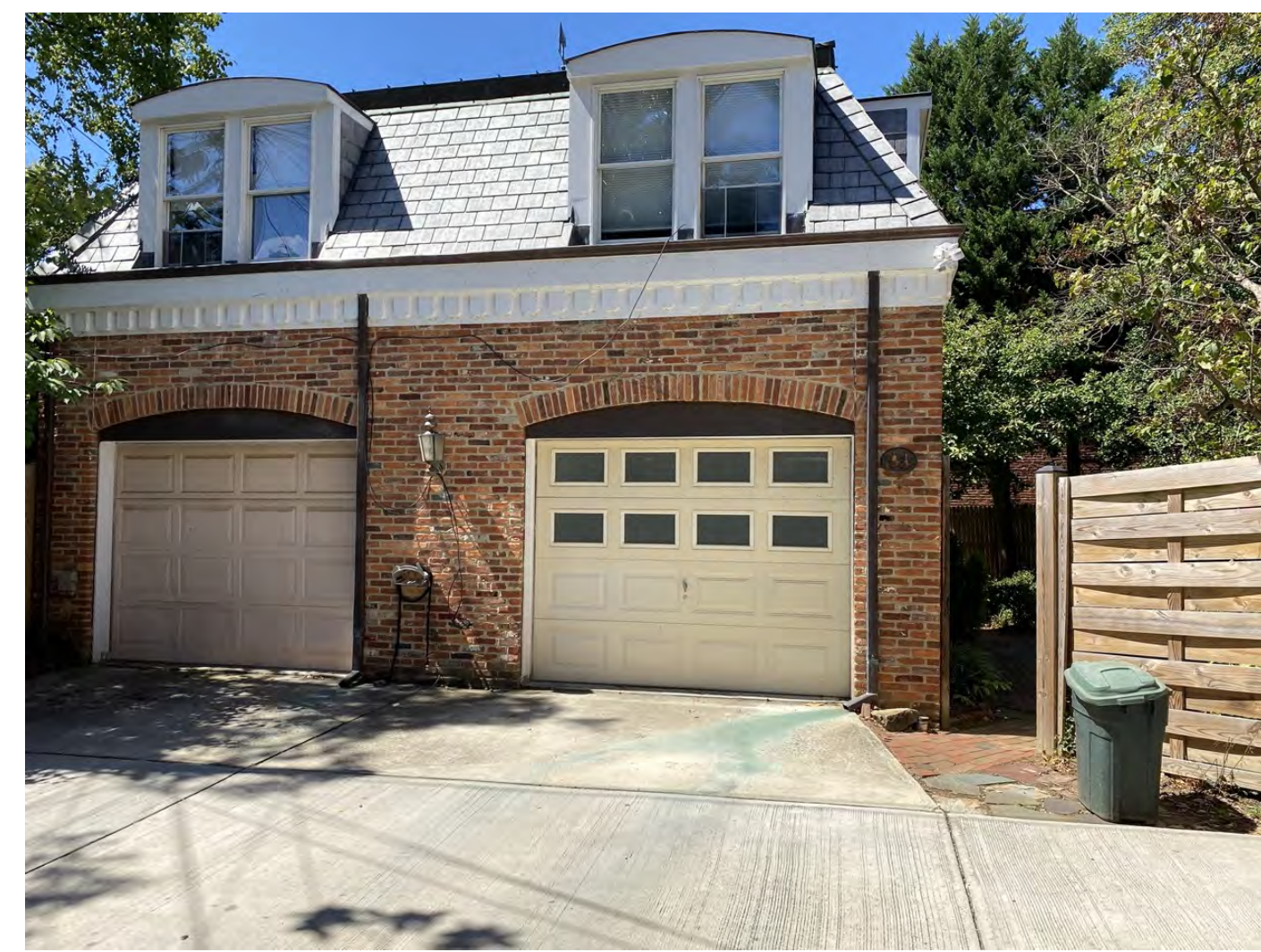
View of Garage and Concrete Pad and Gate From The Alley (Prior to Start of House Renovation)
