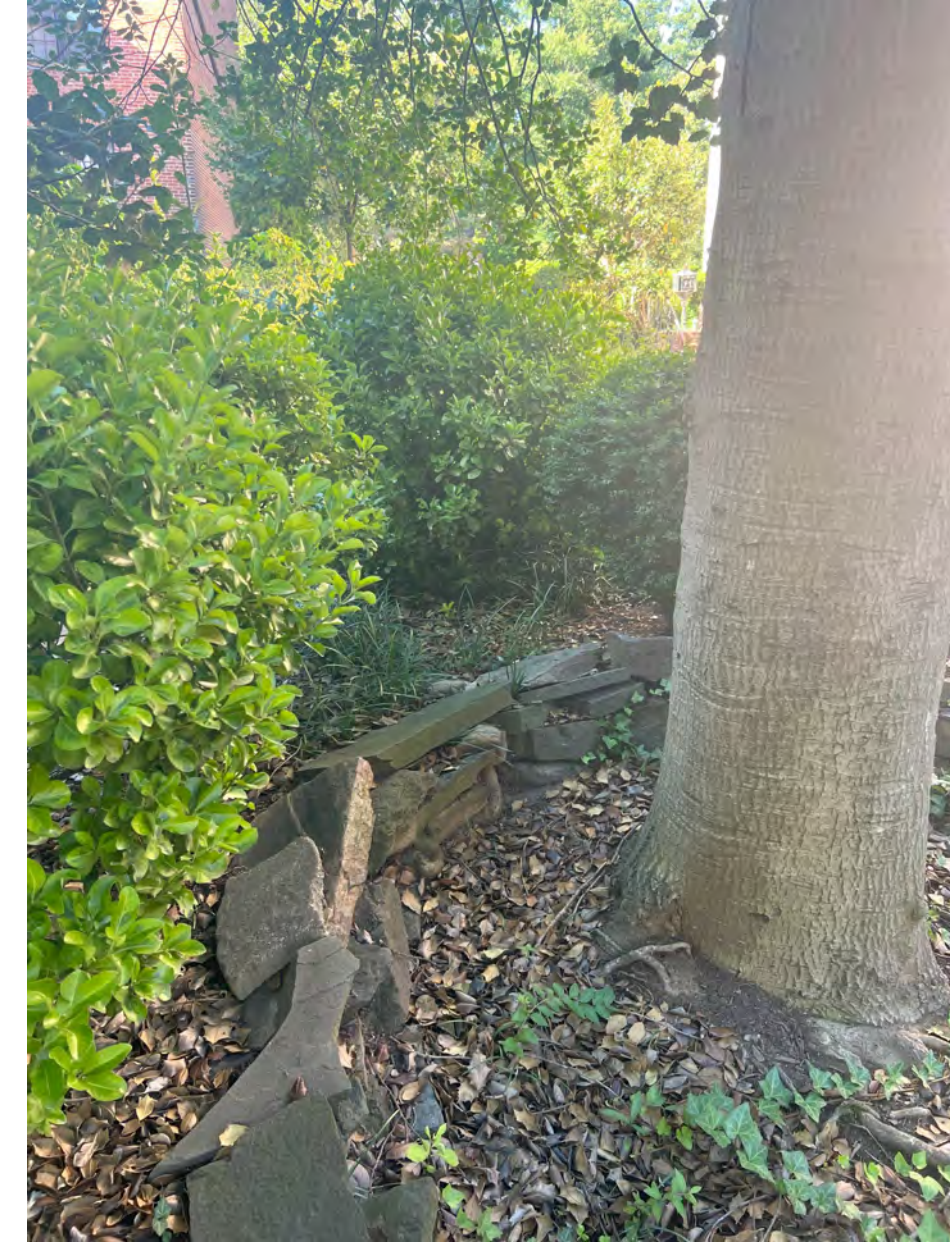
2. Existing low wall around Holly
