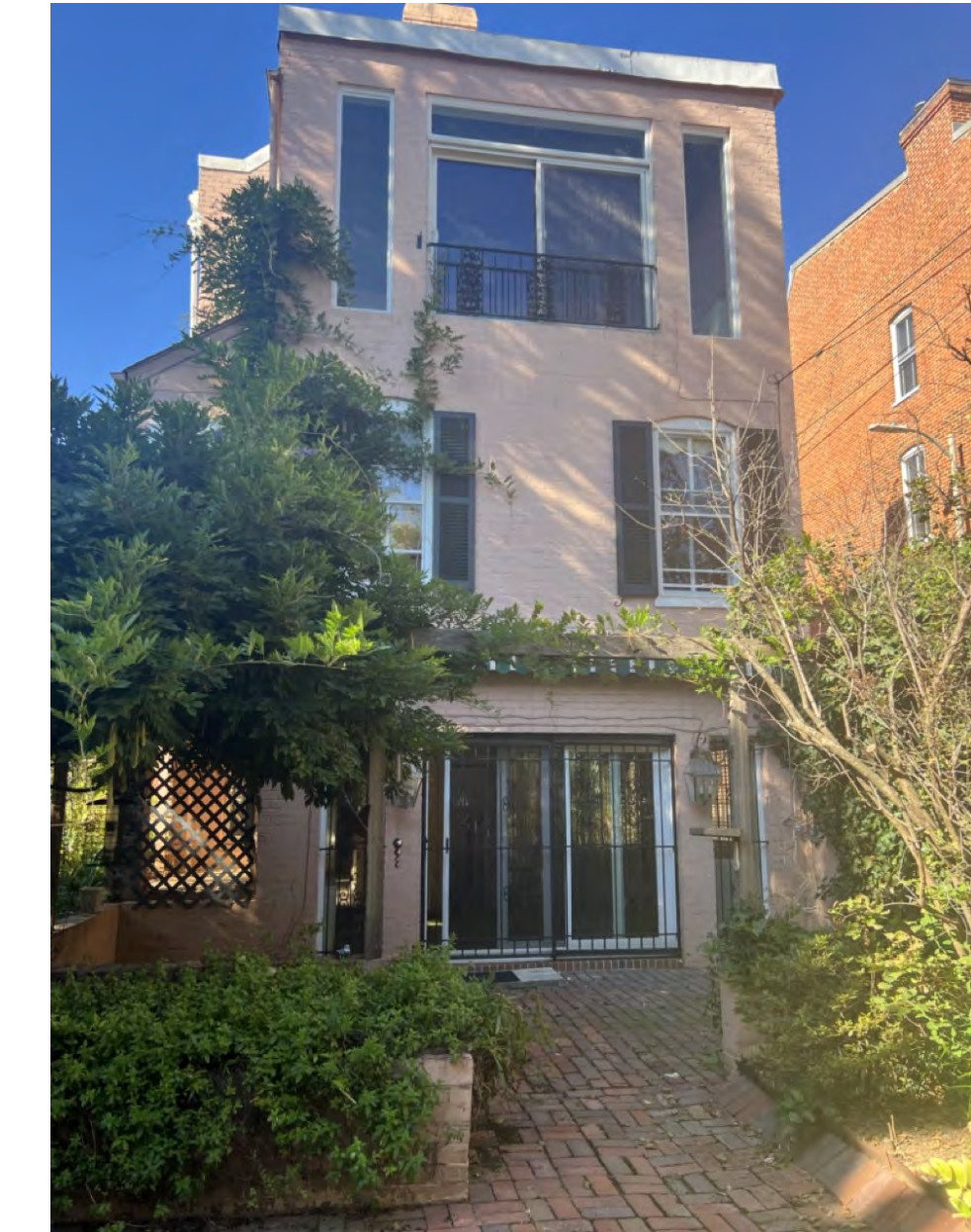
Existing Paved Terrace at Back of House (Prior to Start of House Renovation)
