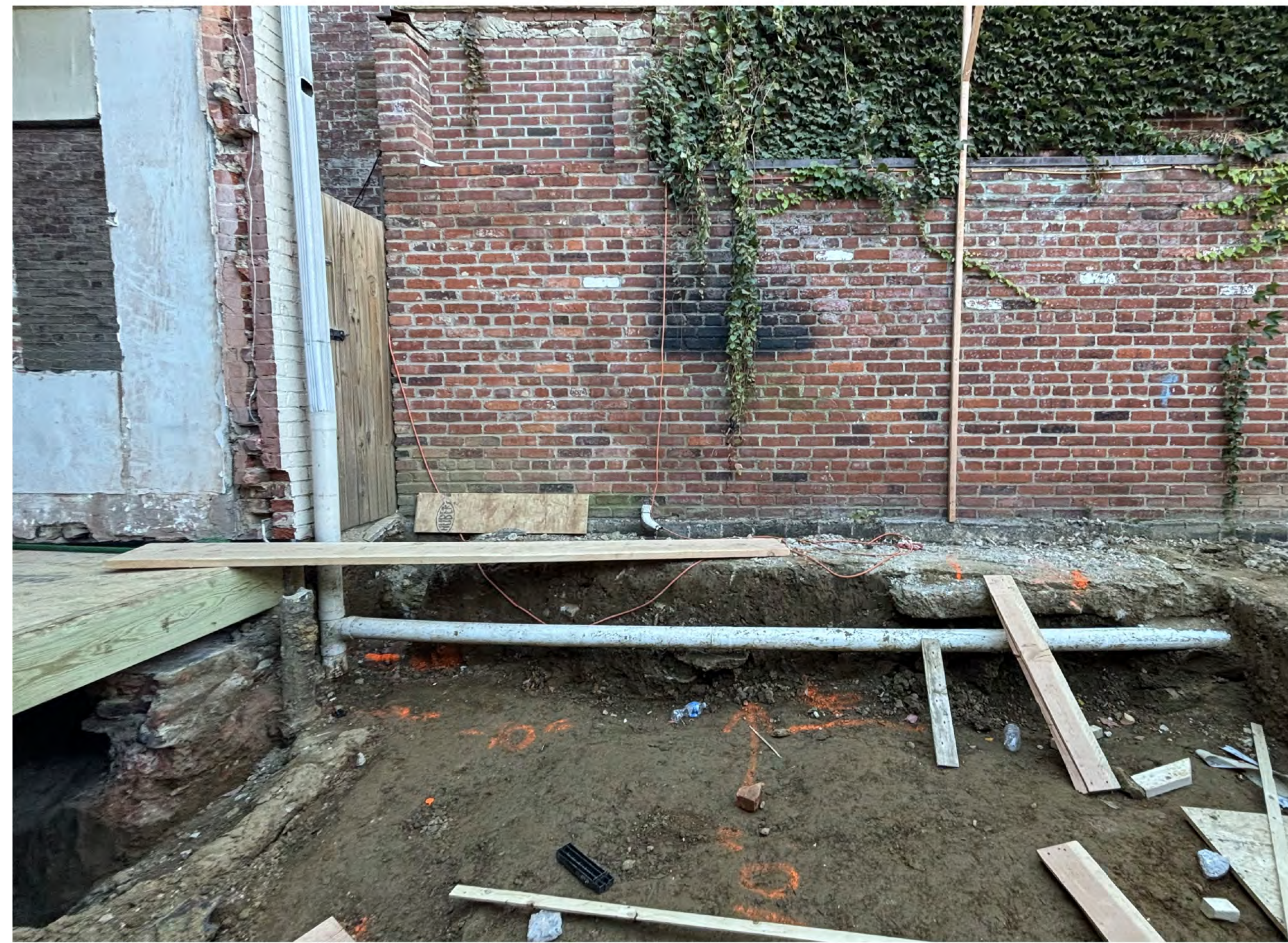
VIEW OF CONSTRUCTION - AREA OF NEW ADDITION
