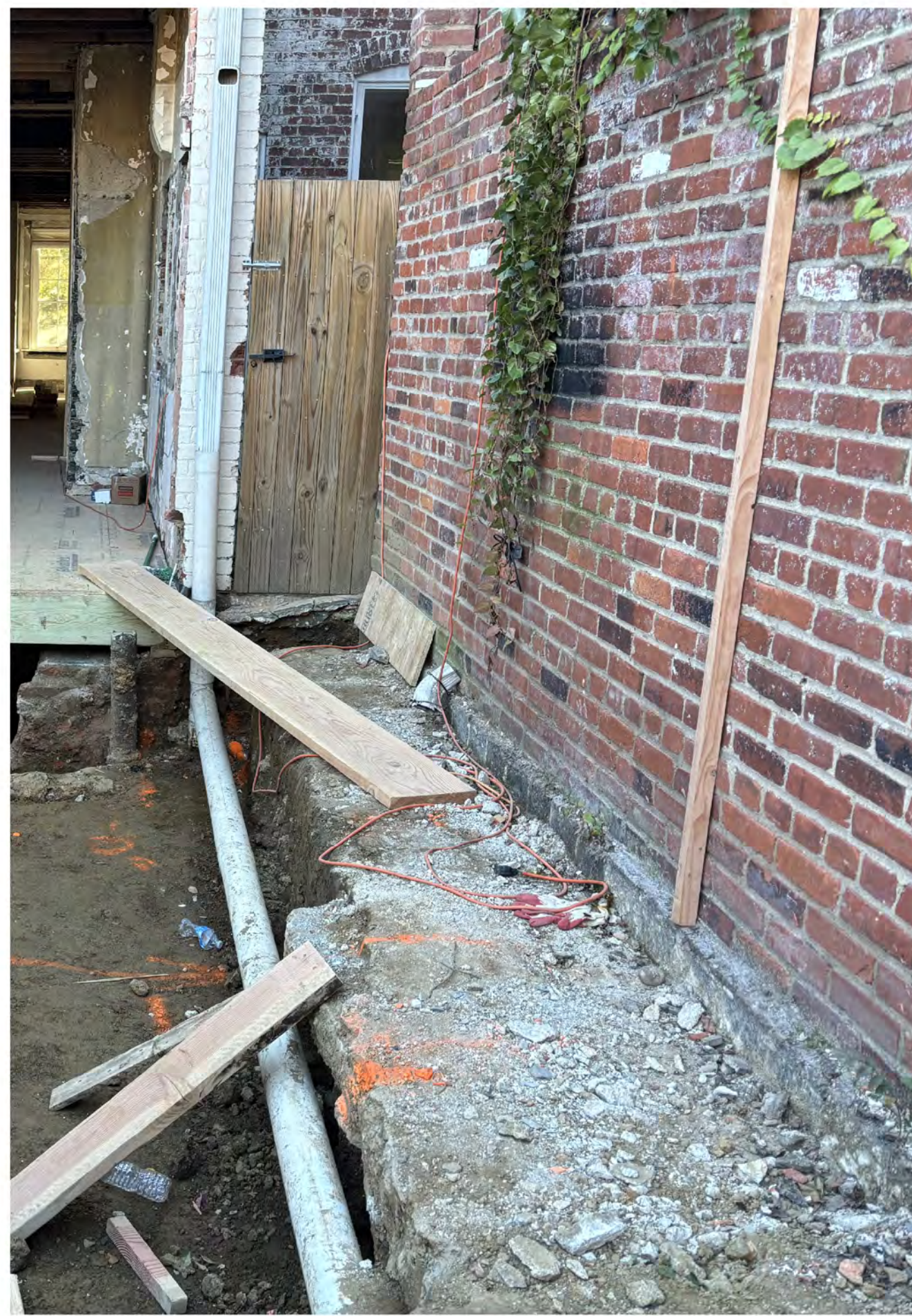
VIEW OF CONSTRUCTION - AREAWAY
