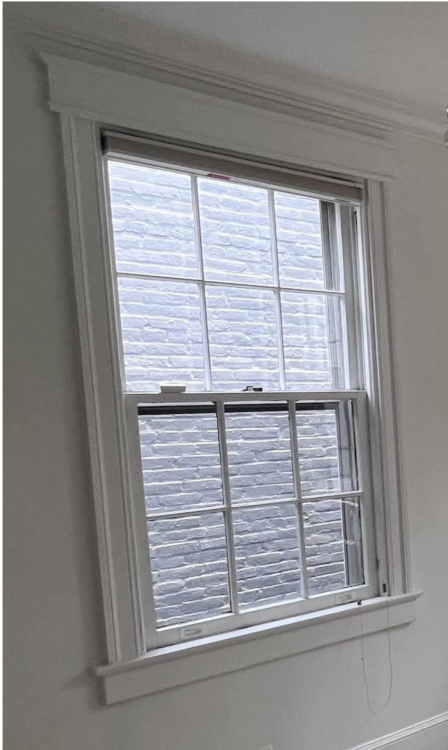
PHOTO OF THE EXISTING WINDOW
