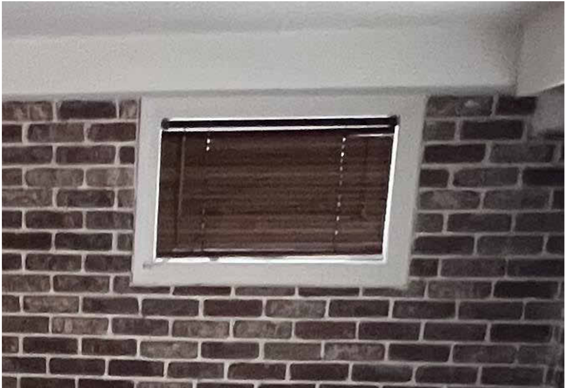
PHOTO OF THE EXISTING WINDOW
