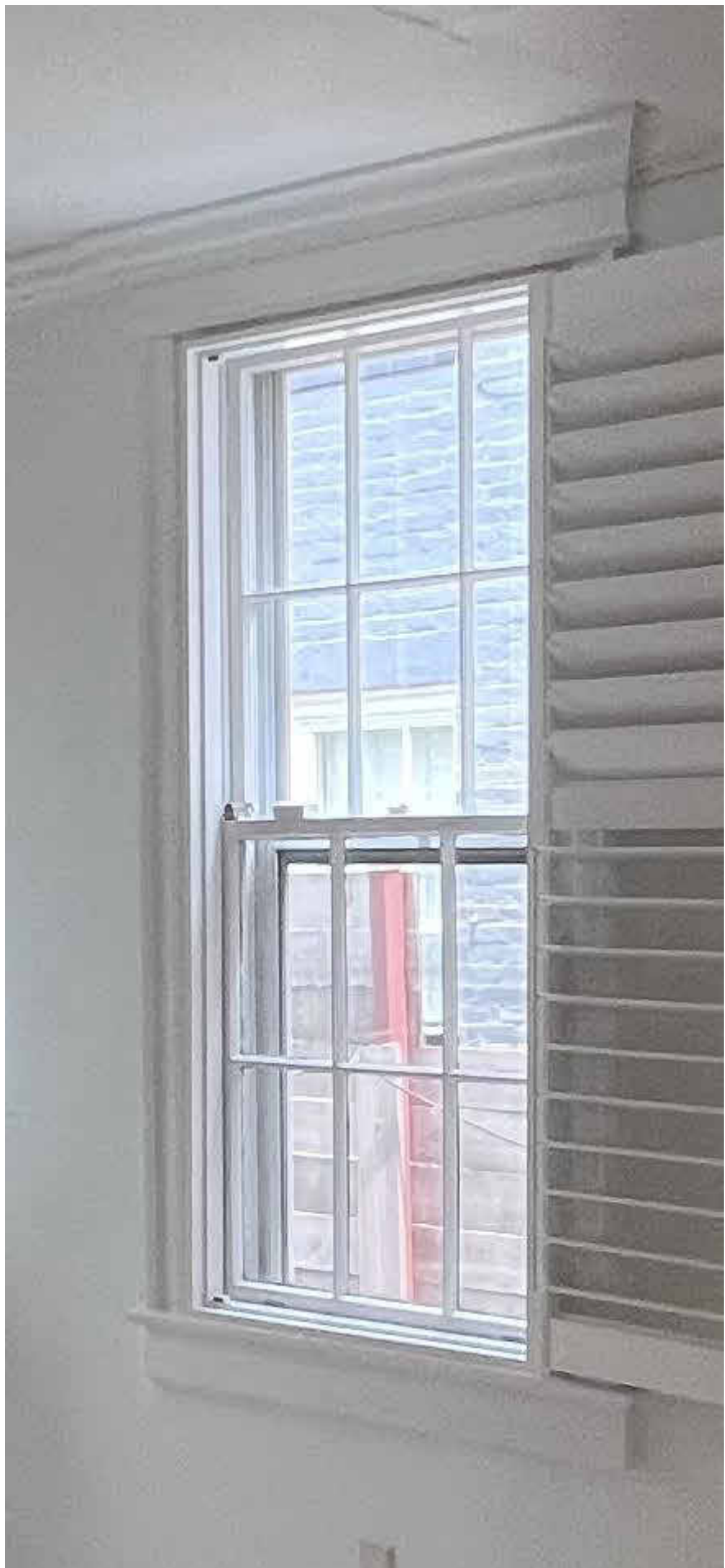
PHOTO OF THE EXISTING WINDOW
