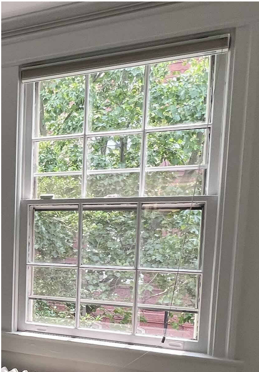
PHOTO OF THE EXISTING WINDOW
