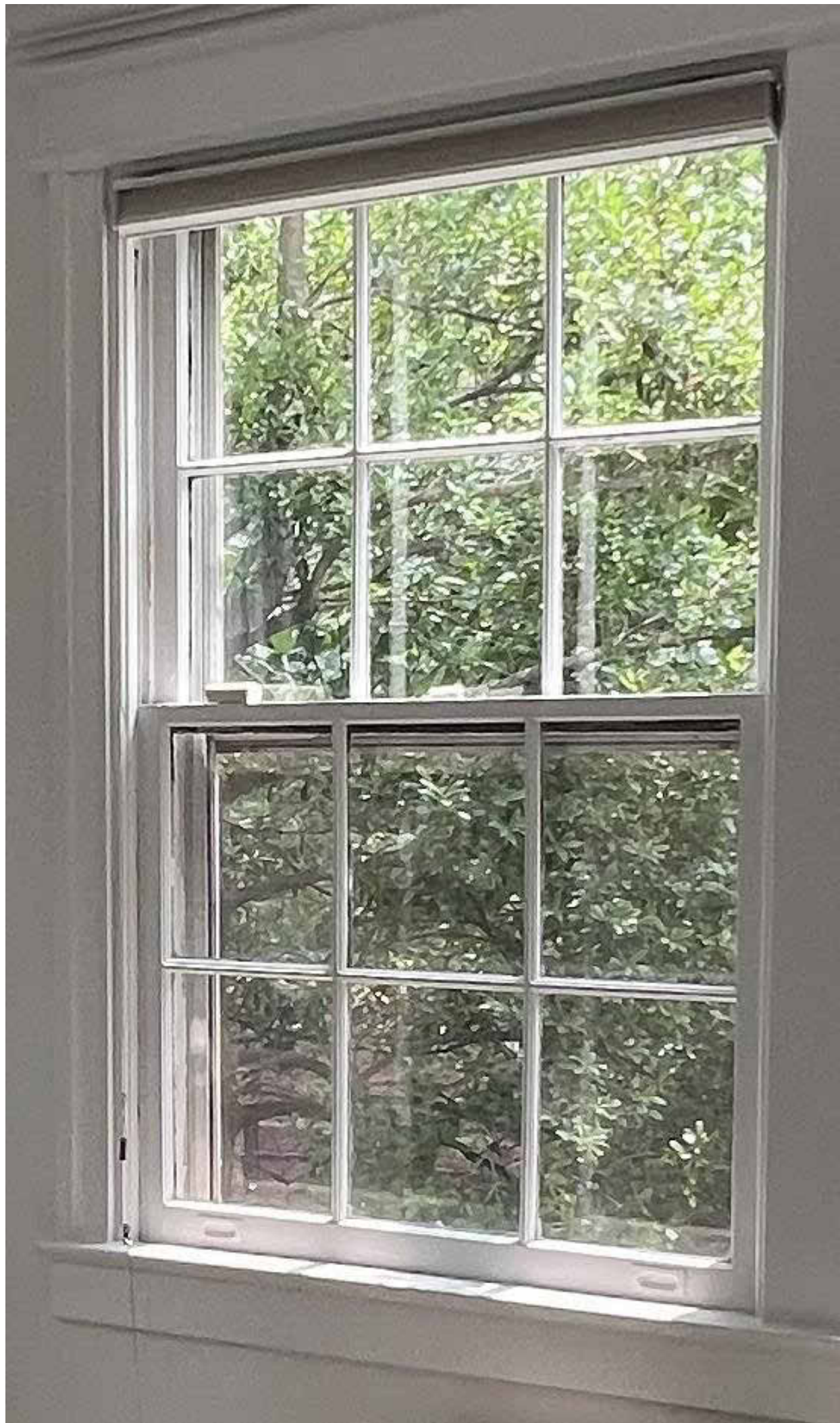
PHOTO OF THE EXISTING WINDOW
