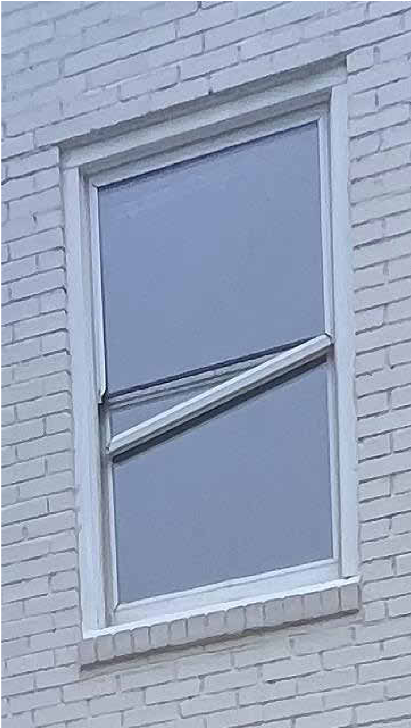
PHOTO OF THE EXISTING WINDOW
