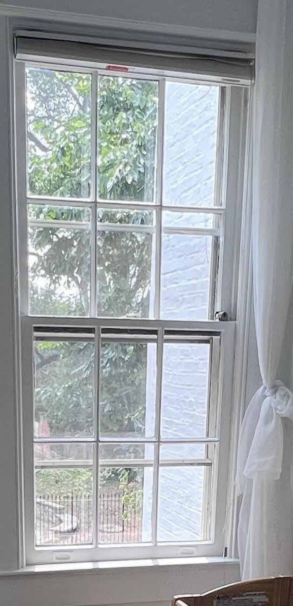
PHOTO OF THE EXISTING WINDOW
