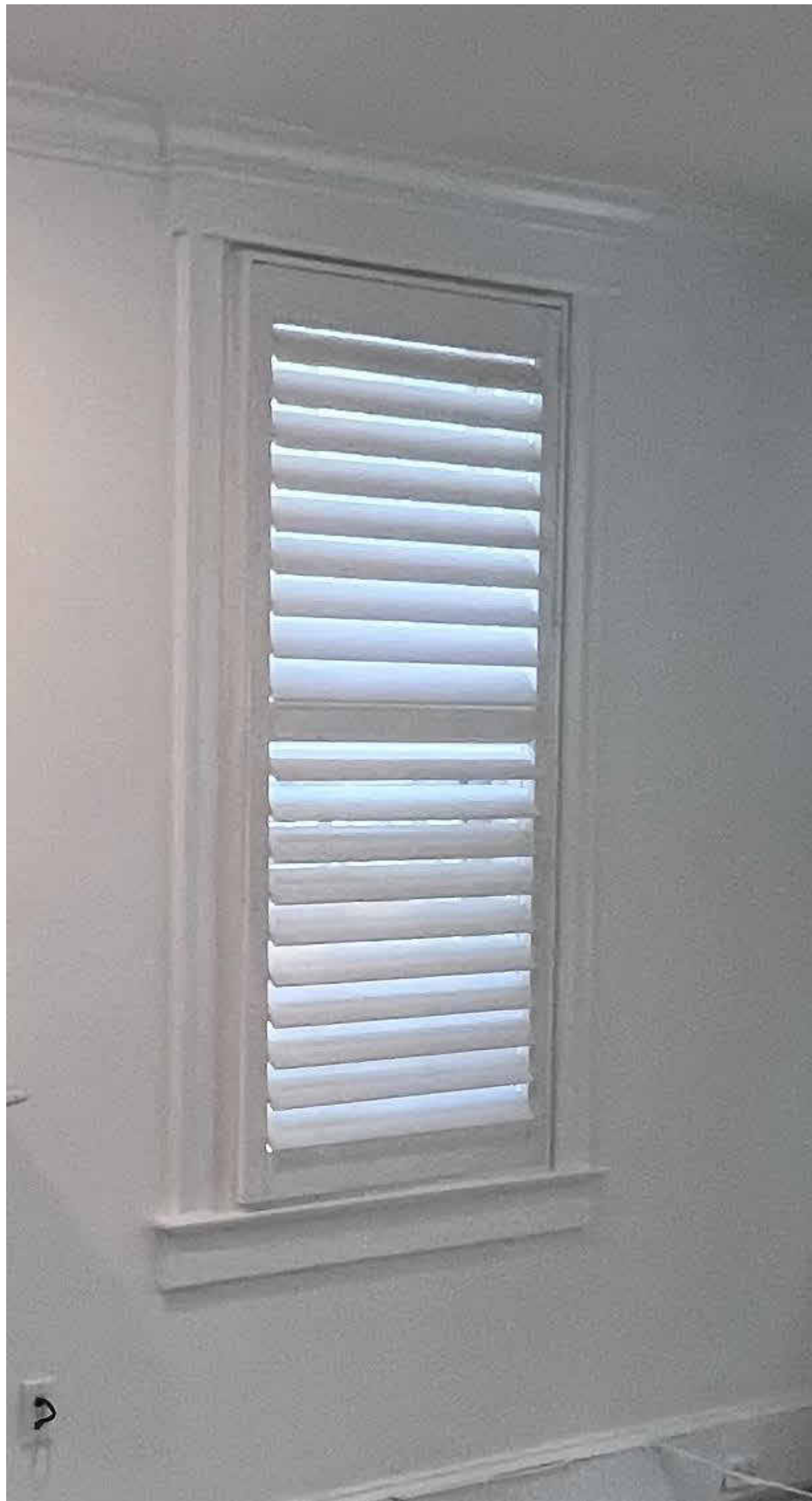
PHOTO OF THE EXISTING WINDOW
