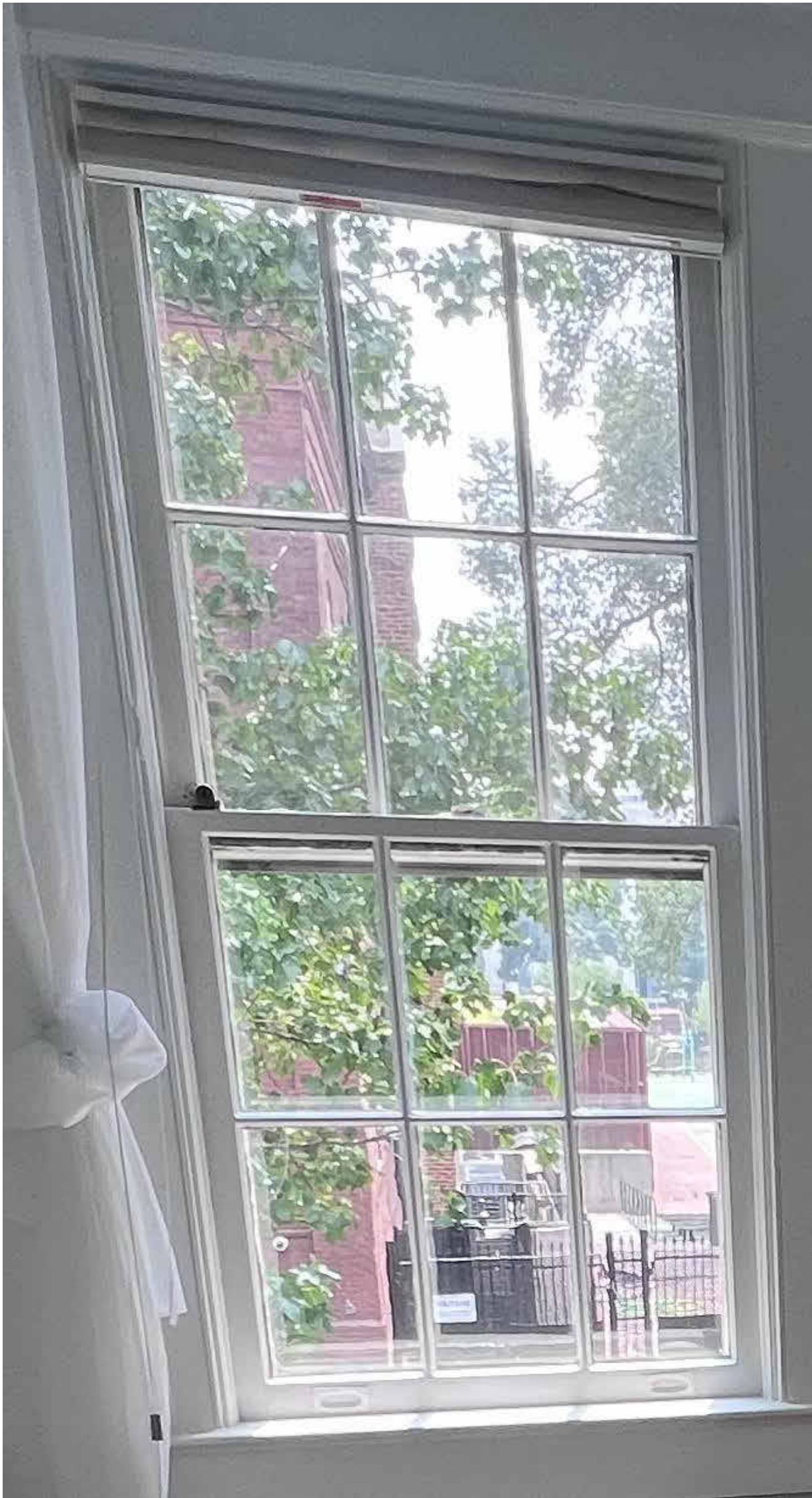
PHOTO OF THE EXISTING WINDOW
