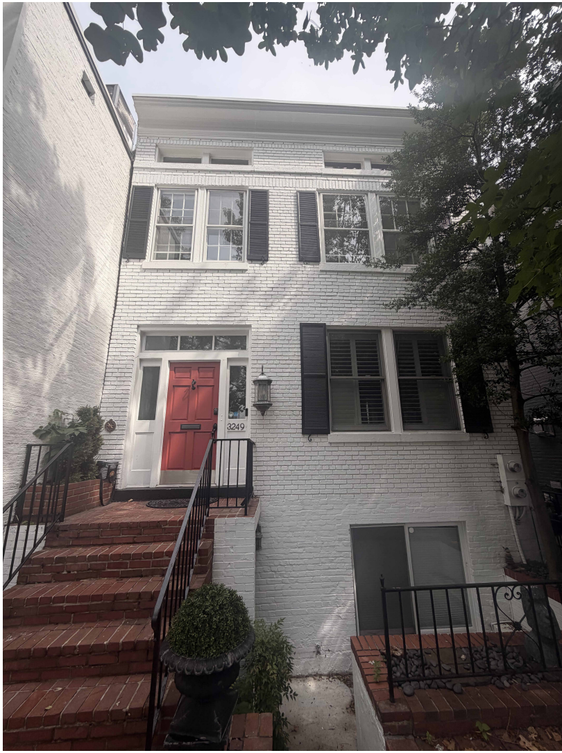
EXISTING FRONT FACADE
