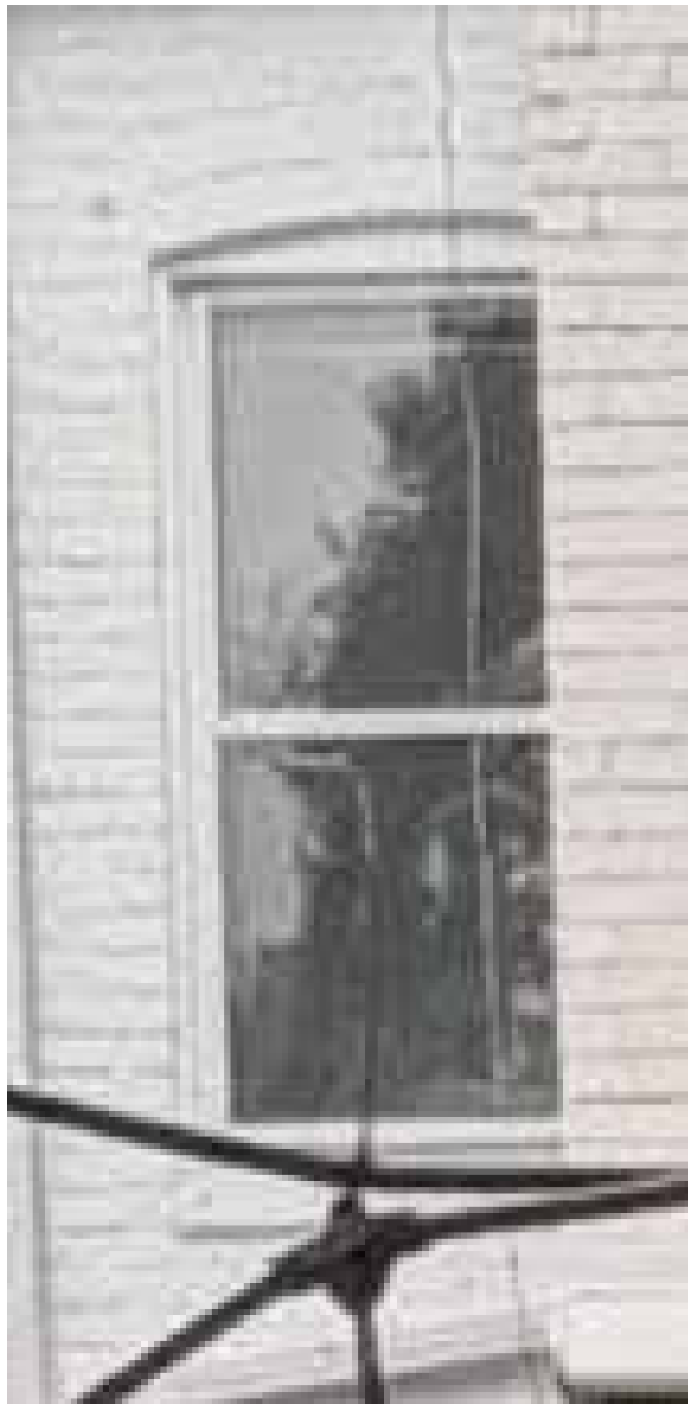
PHOTO OF THE EXISTING WINDOW
