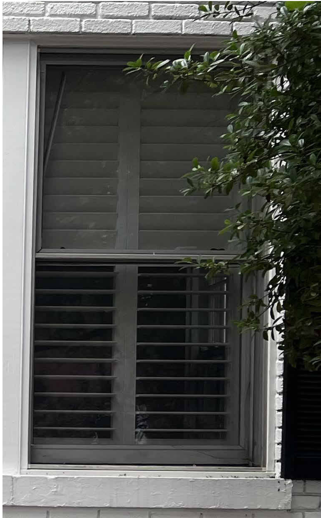
PHOTO OF THE EXISTING WINDOW
