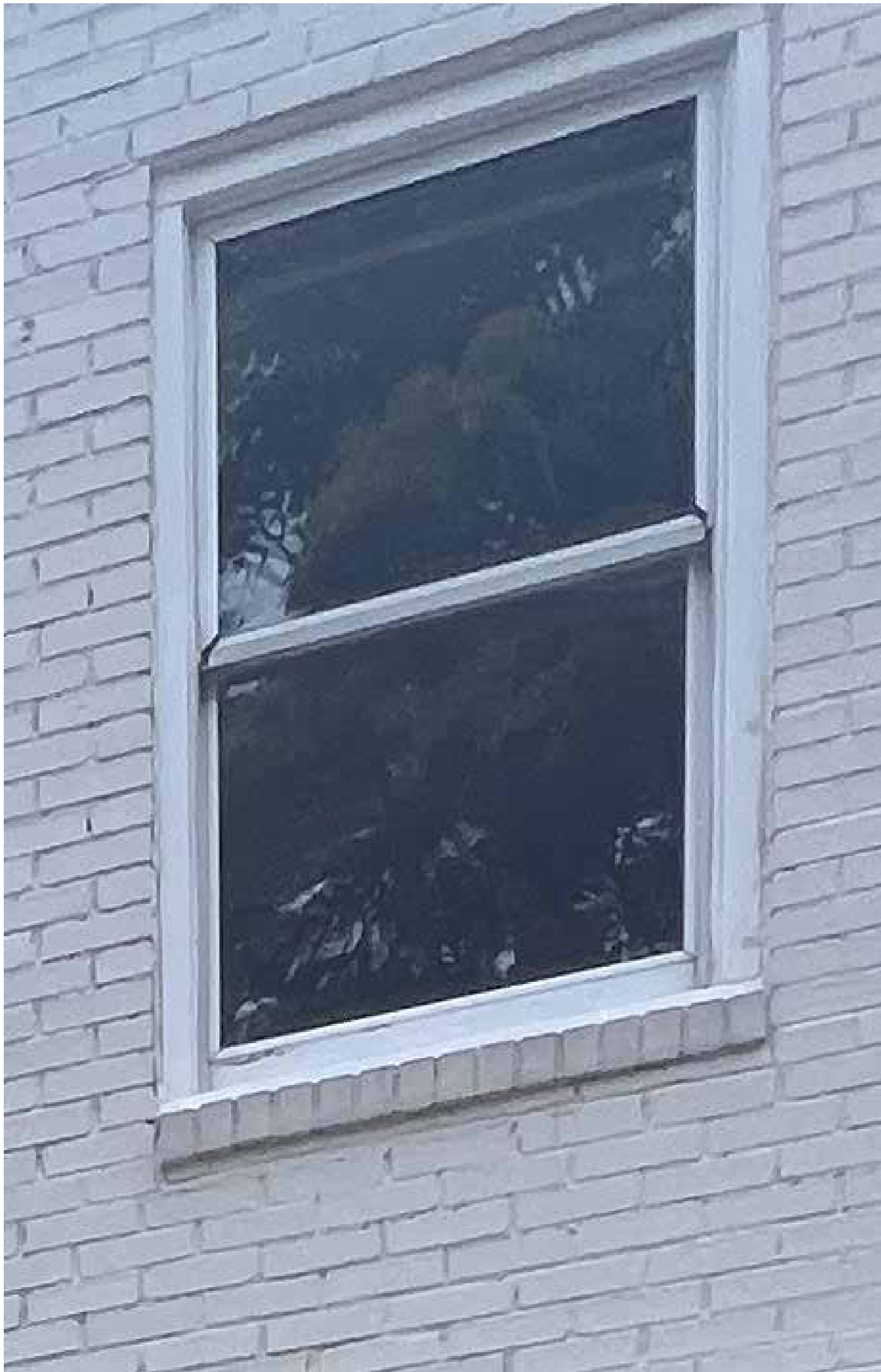
PHOTO OF THE EXISTING WINDOW
