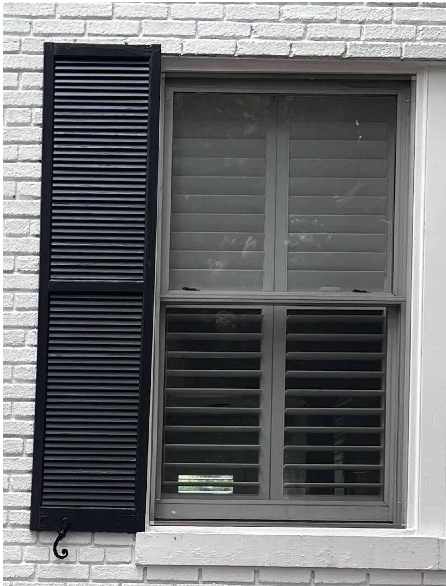
PHOTO OF THE EXISTING WINDOW
