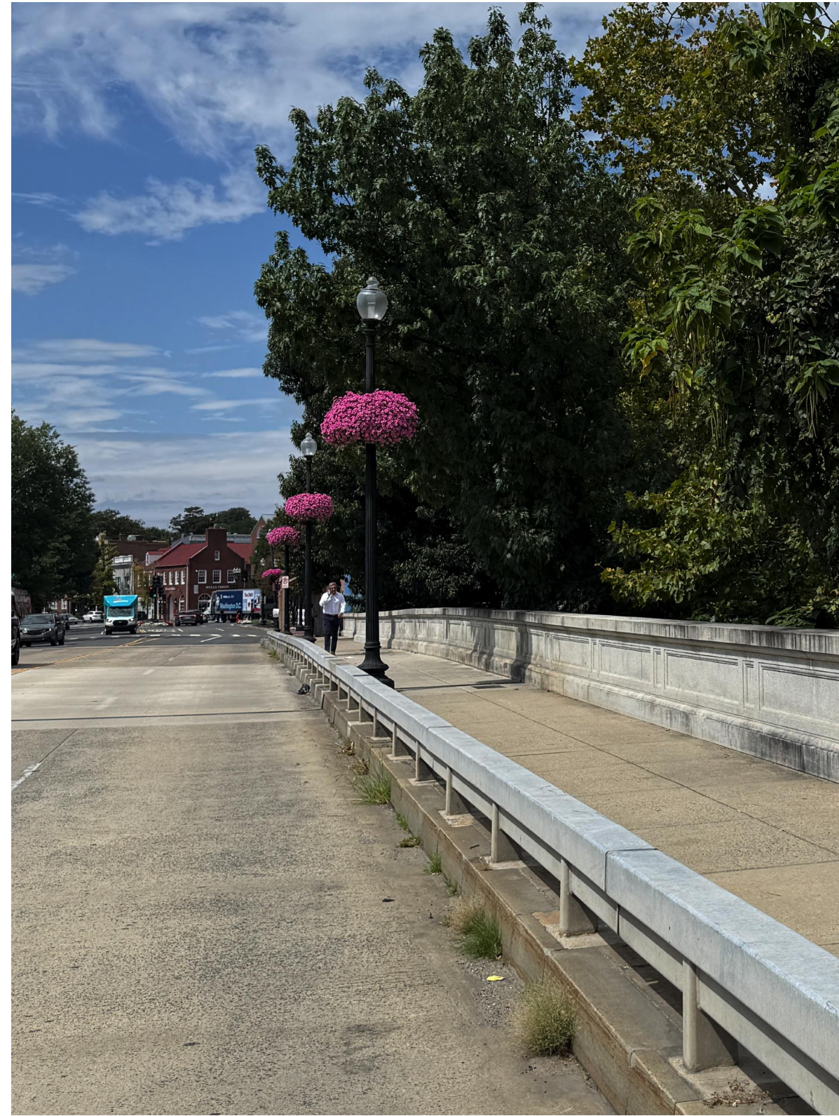
3 2600 BLOCK OF PENNSYLVANIA AVE. (BRIDGE)
