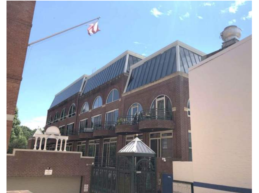
VIEW FROM STREET TO BACK OF BLDG
