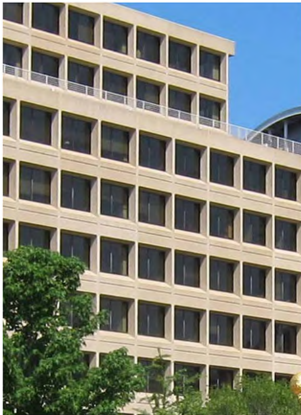
Judiciary Plaza Office Building
