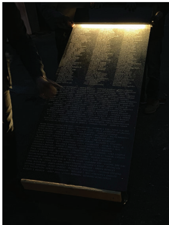
LED light strip at top beneath stone trim - Visible hot spot - Not enough light at bottom of wall
