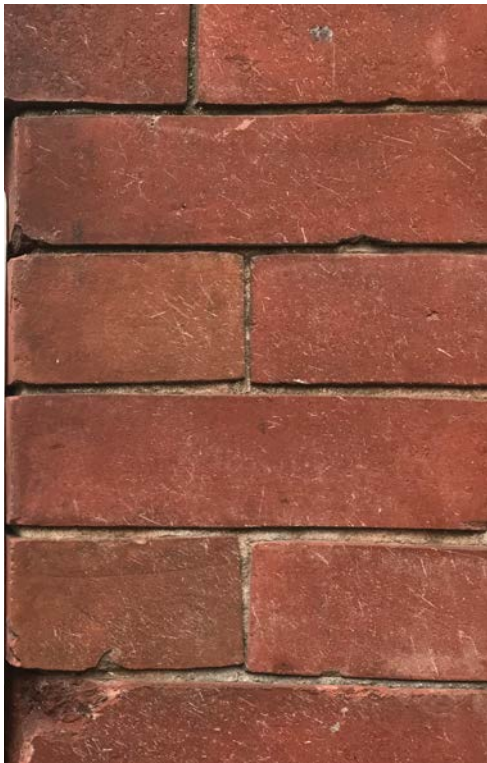
BRICK @ EXISTING BUILDING
