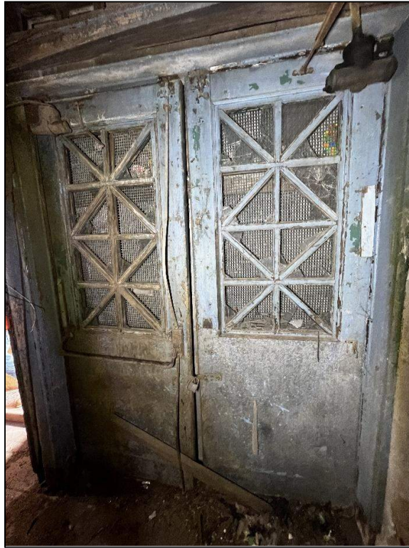
Figure 5: Wooden door at northern entrance.
