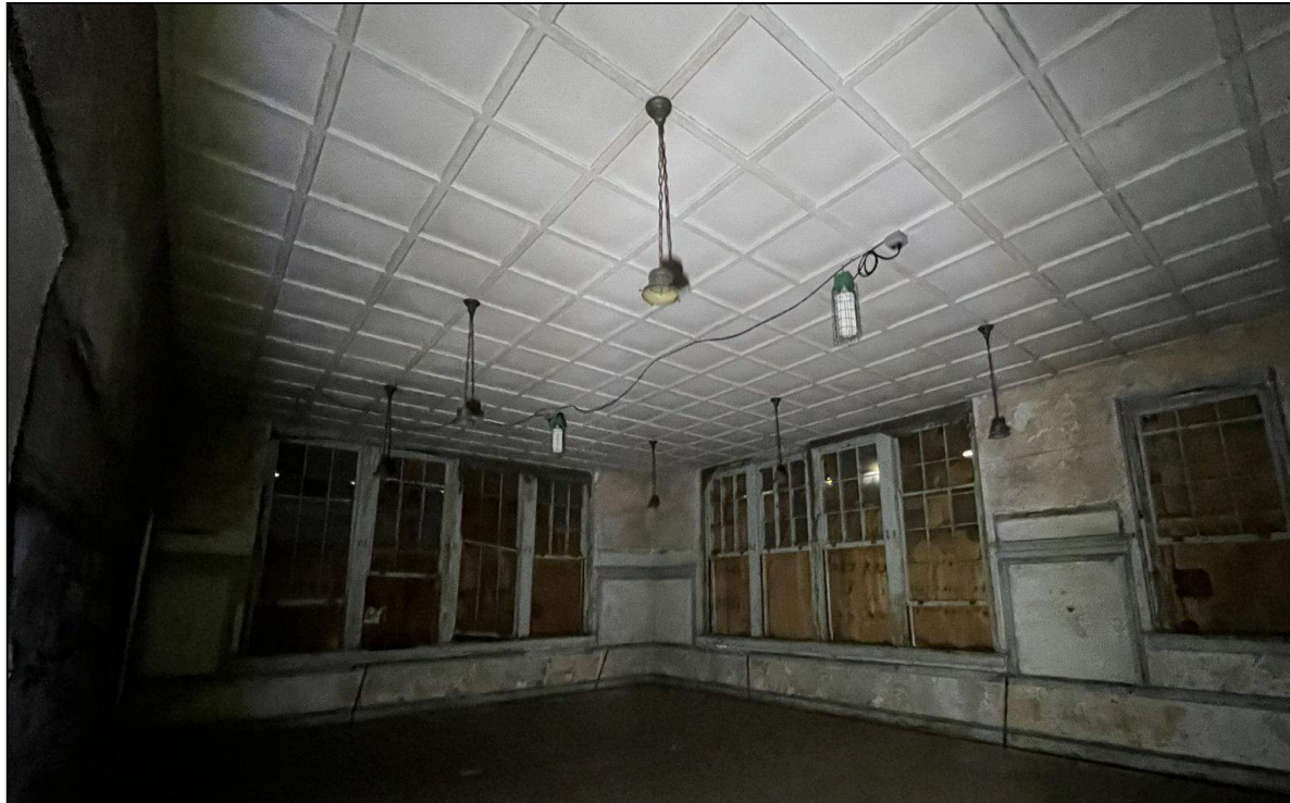
Figure 7: Second floor classroom, note intact ceiling.
