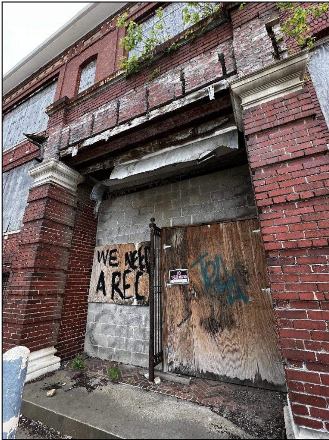
Figure 3: Entrance on north elevation.
